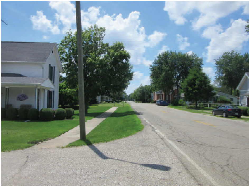
10. From approximately 0.05 mile west of the SR 59 (Main Street) and Cross Street intersection looking west at SR 59 and street scape
