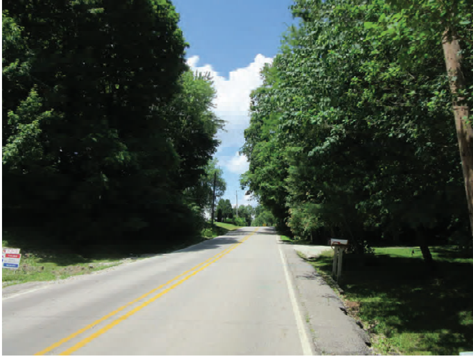
3. From approximately 0.05 mile north of the SR 59 and CR 1150 intersection looking north at SR 59 (roadside ditch (RSD) 1 shown right)
