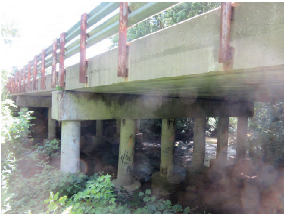
22. From southwest quadrant of Structure No. 059-54-05061 looking northeast at Structure No. 059-54-05061
