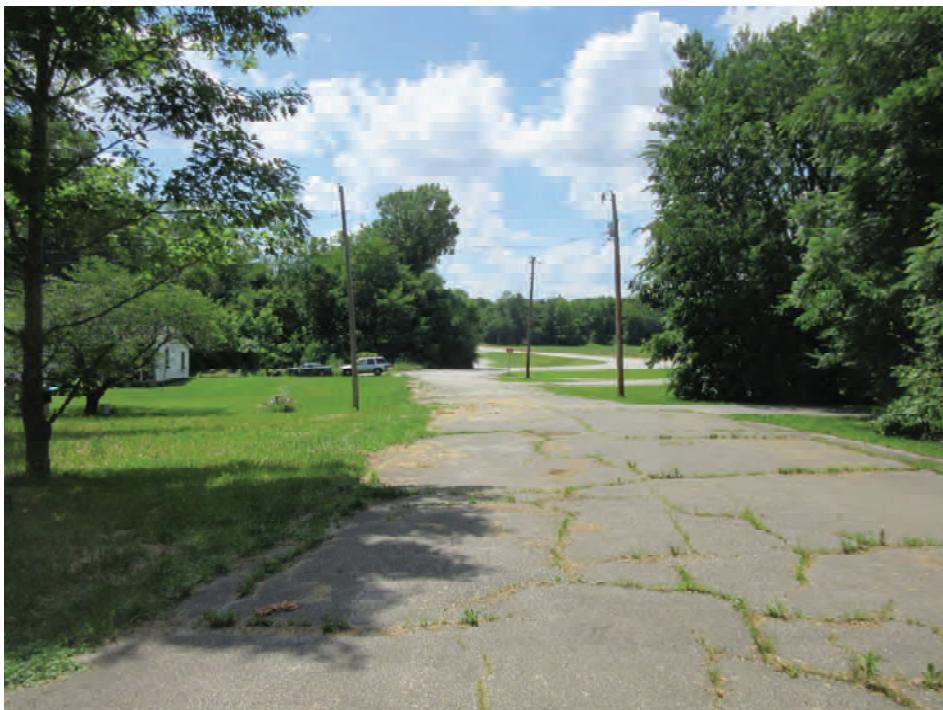
30. From Old SR 59 looking west at roadway/residential area
