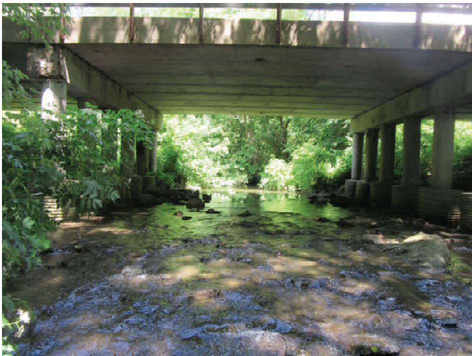
20. From Little Raccoon Creek looking east at Structure No. 059-54-05061 (upstream)
