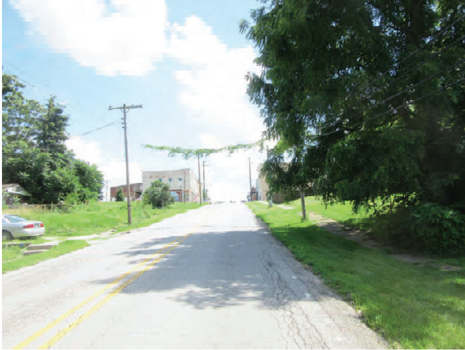
15. From approximately 0.05 mile north of the SR 59 (Cross Street) and Green Street intersection looking south at SR 59 and sidewalk
