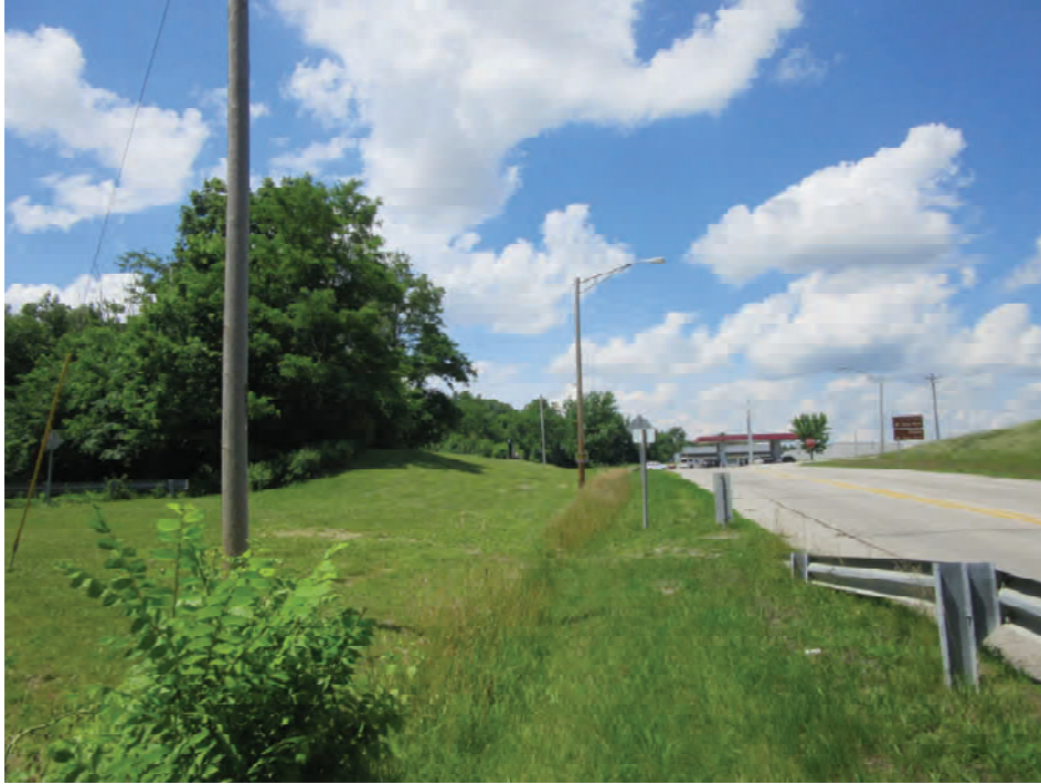
23. From northwest quadrant of Structure No. 059-54-05061 looking north at roadside ditch and SR 59
