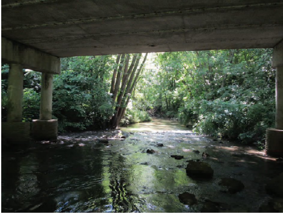
21. From underneath Structure No. 059-54-05061 looking west at Little Raccoon Creek (downstream)
