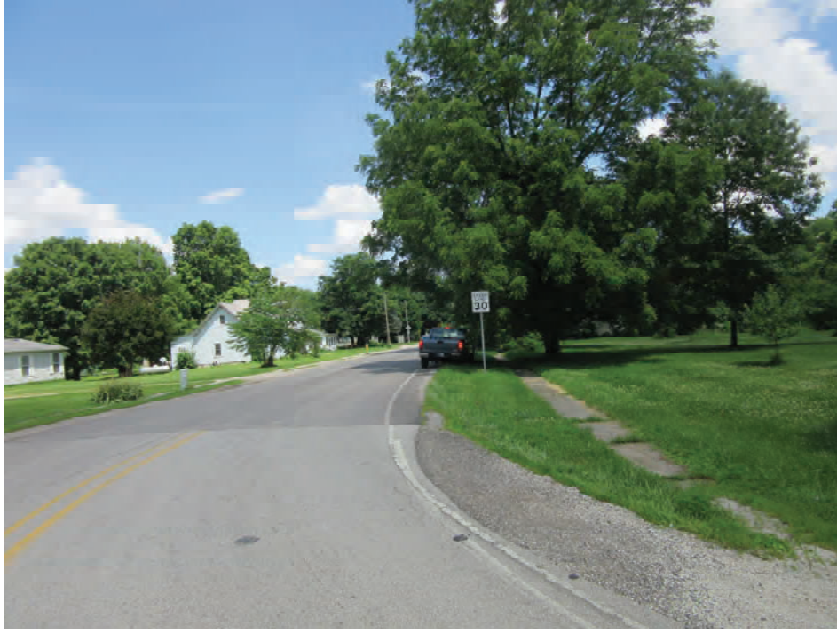
5. From approximately 0.49 mile west of the SR 59 (Main Street) and Cross Street intersection looking east at SR 59 and sidewalk
