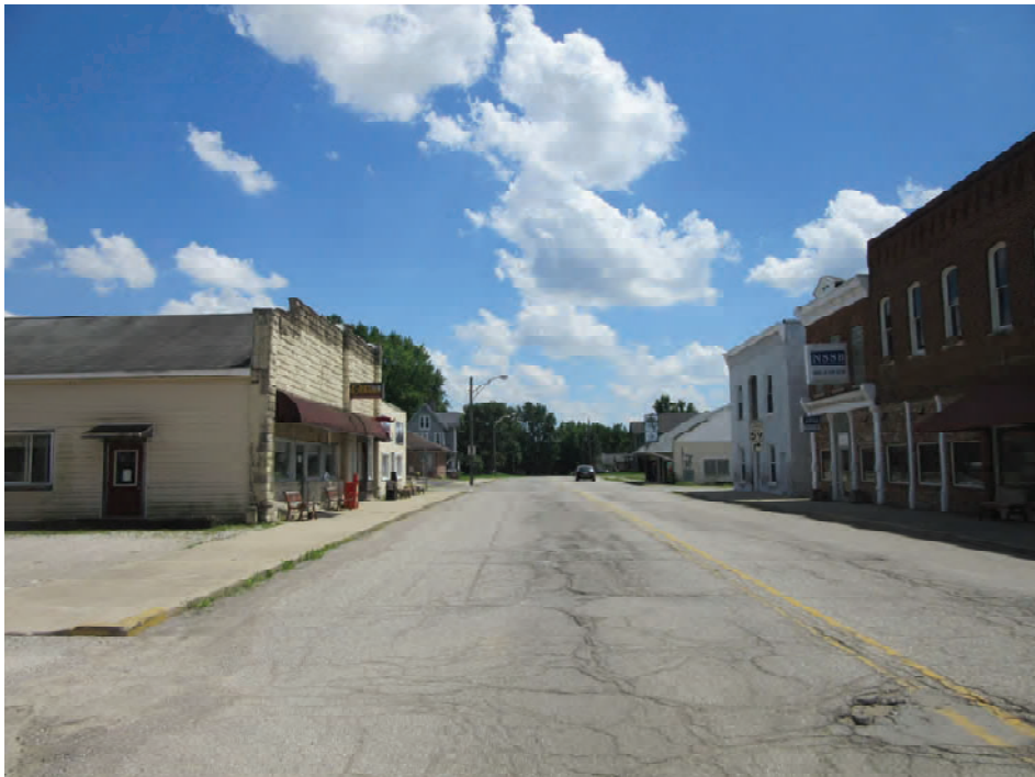
12. From the SR 59 (Cross Street) and Green Street intersection looking south at SR 59 and sidewalk
