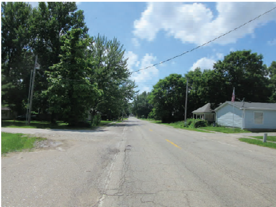
8. From approximately 0.27 mile west of the SR 59 (Main Street) and Cross Street intersection looking west at SR 59 and adjacent landscape
