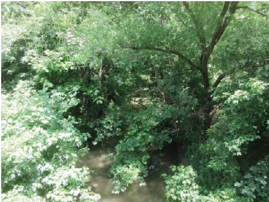
18. From on top Structure No. 059-54-05061 looking east at Little Raccoon Creek (upstream)
