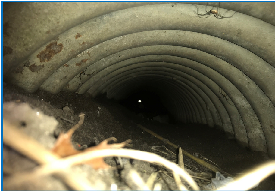
Photo 3 —View of the south end of the clogged culvert (CLV-29637) facing north (05/24/2023).
