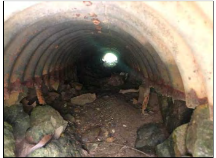
Photo 14. Looking through Str. 2 at inlet, viewing east, 5/13/2022
