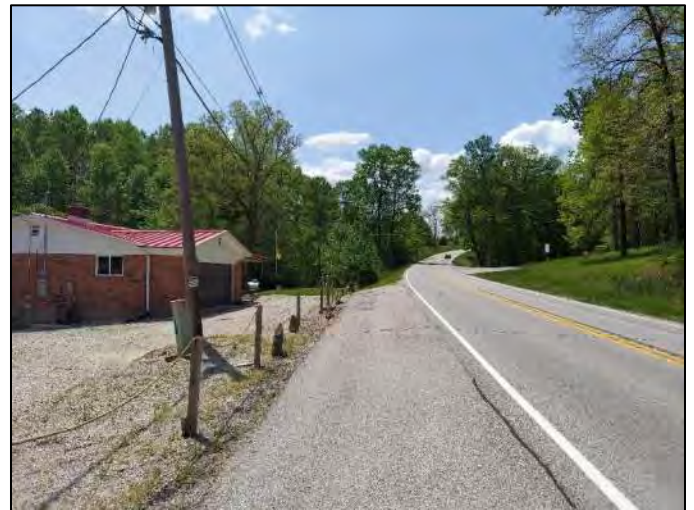
Photo 52. Roadside with residence south of SR 445, viewing west, 5/13/2022
