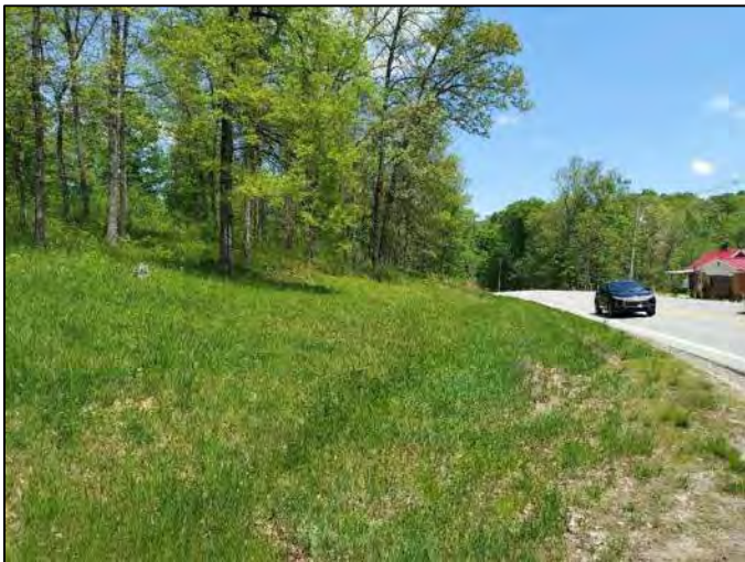
Photo 51. Roadside swale northeast of the SR 445 and Lawrence Hollow Drive intersection, viewing east, 5/13/2022
