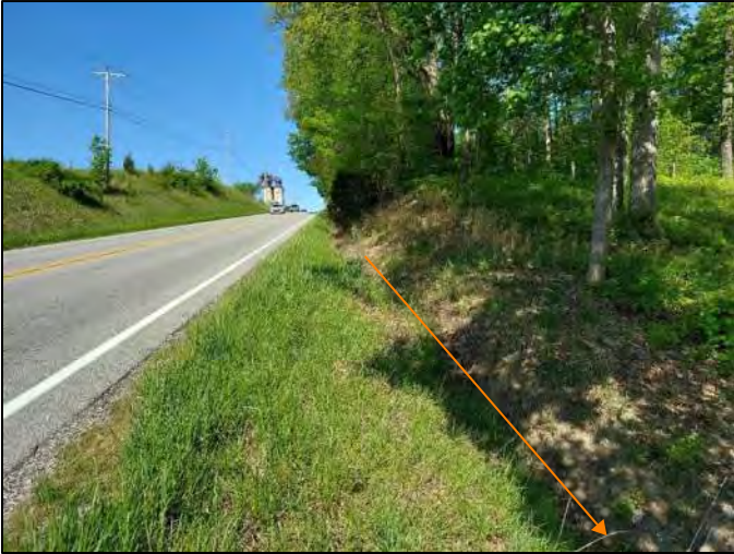
Photo 1. RSD 1 on north side of SR 445, viewing west, 5/13/2022
