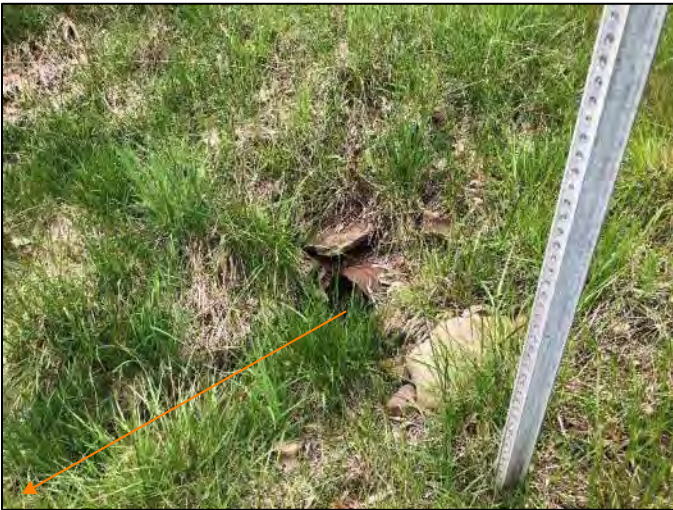
Photo 15. Outlet of Str. 2 with RSD 4, viewing west, 5/13/2022
