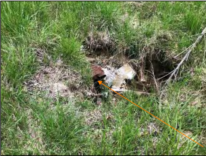
Photo 13. Inlet of Str. 2 with RSD 3, viewing east, 5/13/2022
