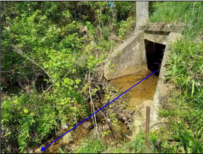
Photo 45. Outlet of culvert (CV 445-28-000.52) with UNT 1 to Beech Creek, viewing west, 5/13/2022
