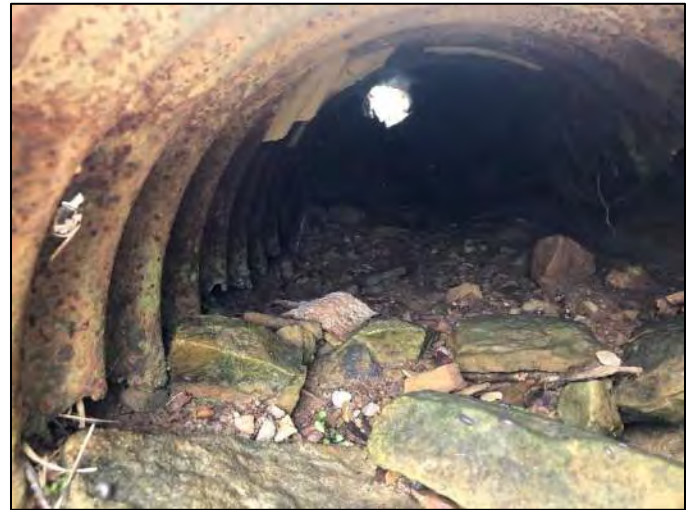
Photo 16. Looking through Str. 2 at outlet, viewing west, 5/13/2022
