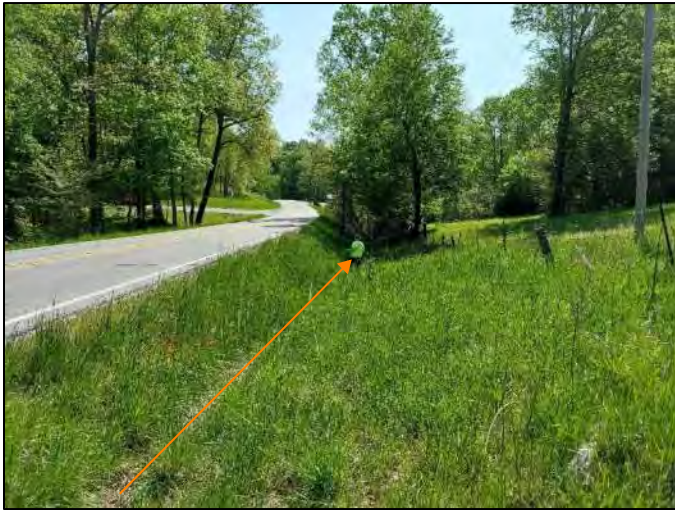
Photo 29. RSD 5 flowing towards UNT 1 to Beech Creek, eroded area starts at trees within the ditch line, viewing east, 5/13/2022
