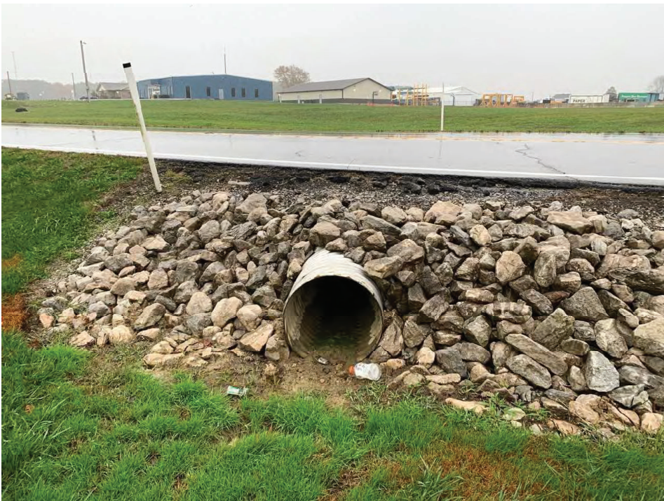
3. Looking southeast at culvert under SR 56
