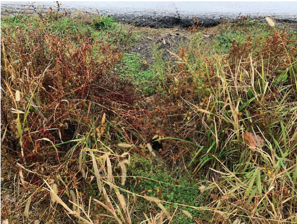
19. Looking west at culvert under Boatman Road
