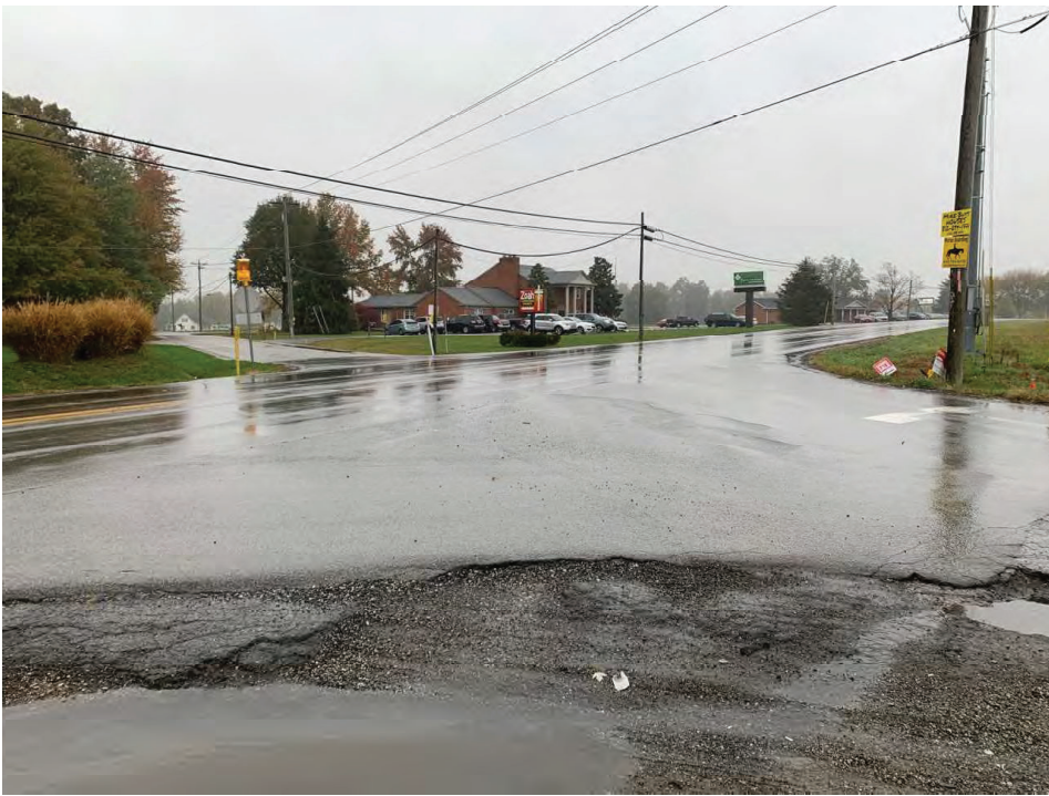
9. Looking northeast at intersection of SR 56 and Boatman Road
