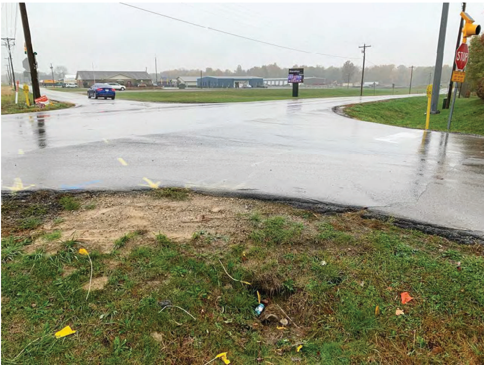
11. Looking southwest at intersection of SR 56 and Boatman Road
