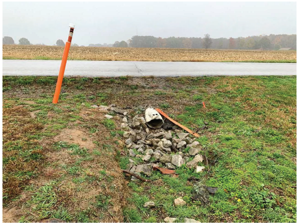
18. Looking east at Culvert under Boatman Road
