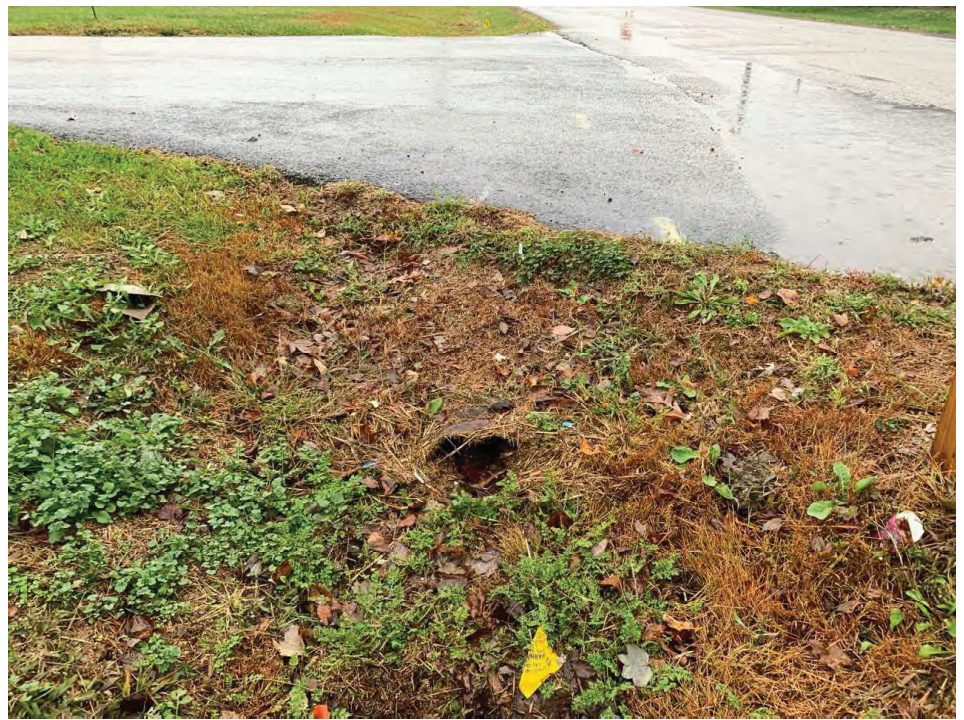
22. South at culvert under entrance drive
