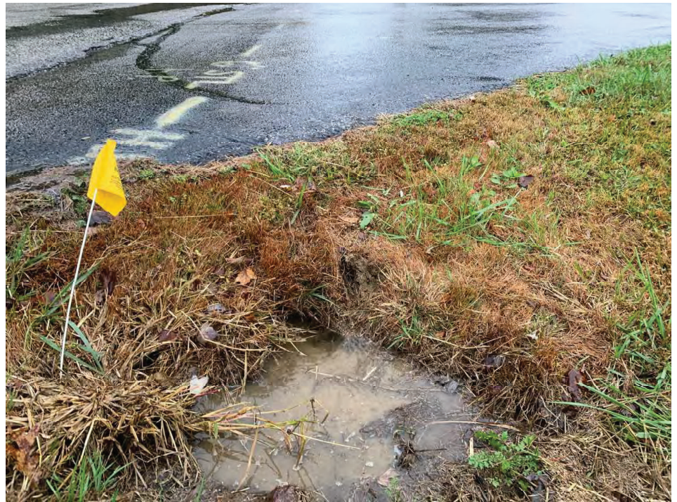
20. Looking north culvert under entrance drive
