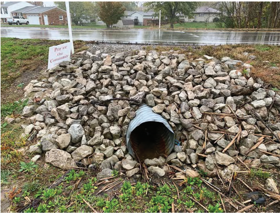
5. Looking northwest at culvert under SR 56
