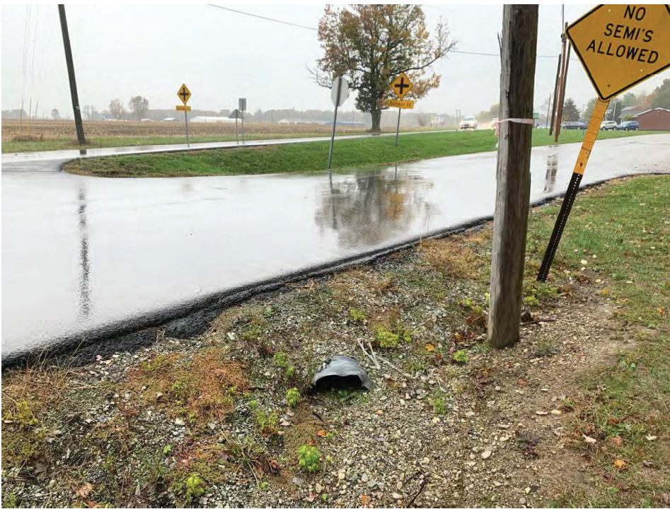
13. Looking southwest at culvert under Mount Drive
