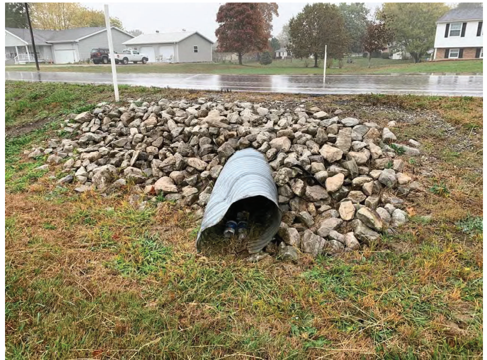
4. Looking northwest at culvert under SR 56
