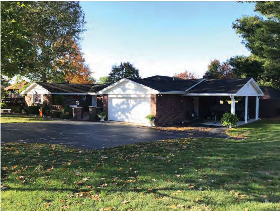
44. Looking SW outside APE in Lake Hosea Subdivision at Lochmueller #14, Contributing, 2173 Bob White Drive
