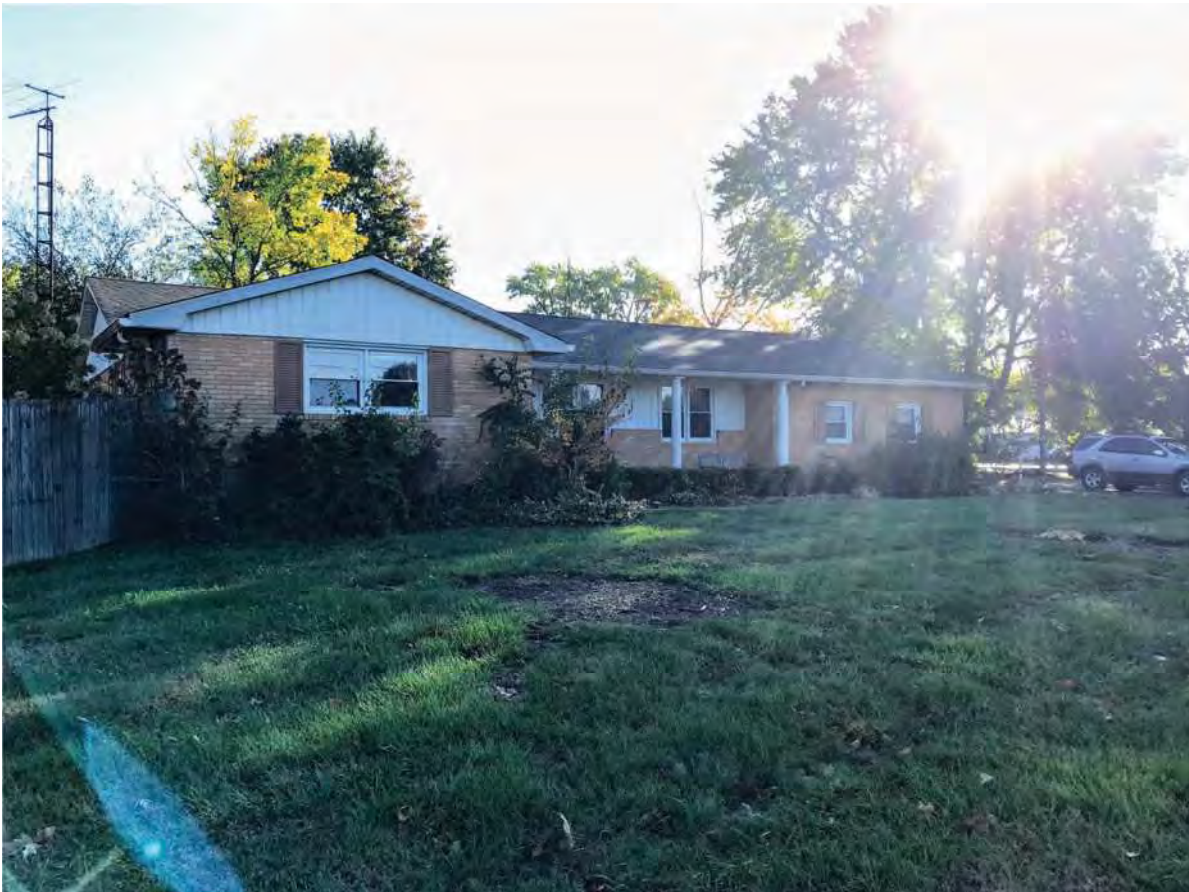
42. Looking E outside APE in Lake Hosea Subdivision at Lochmueller #12, Contributing, 2152 Bob White Drive
