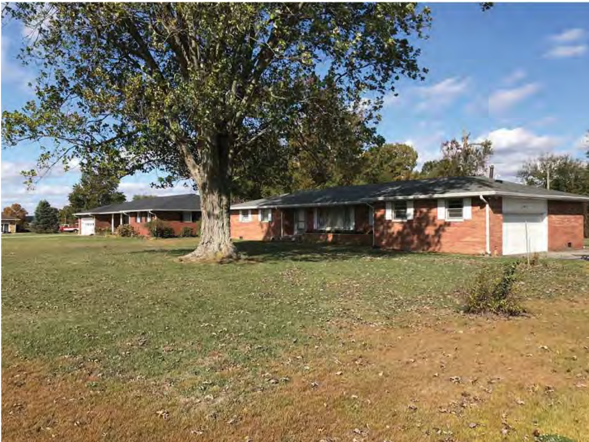
54. Looking NW outside APE in Lake Hosea Subdivision at 2324 W. State Road 56 and 514 S Whippoorwill Lane
