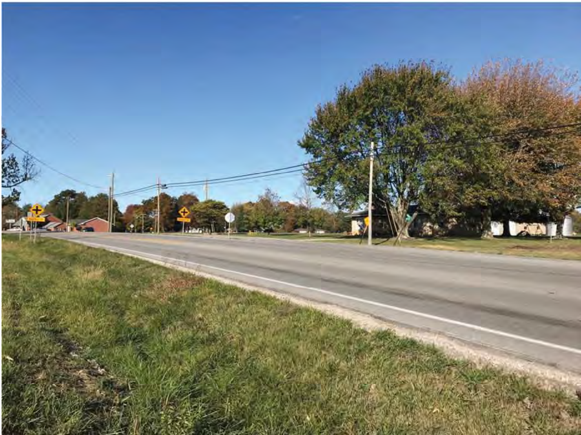
30. Looking NW at the intersection of SR 56 and Mount Drive
