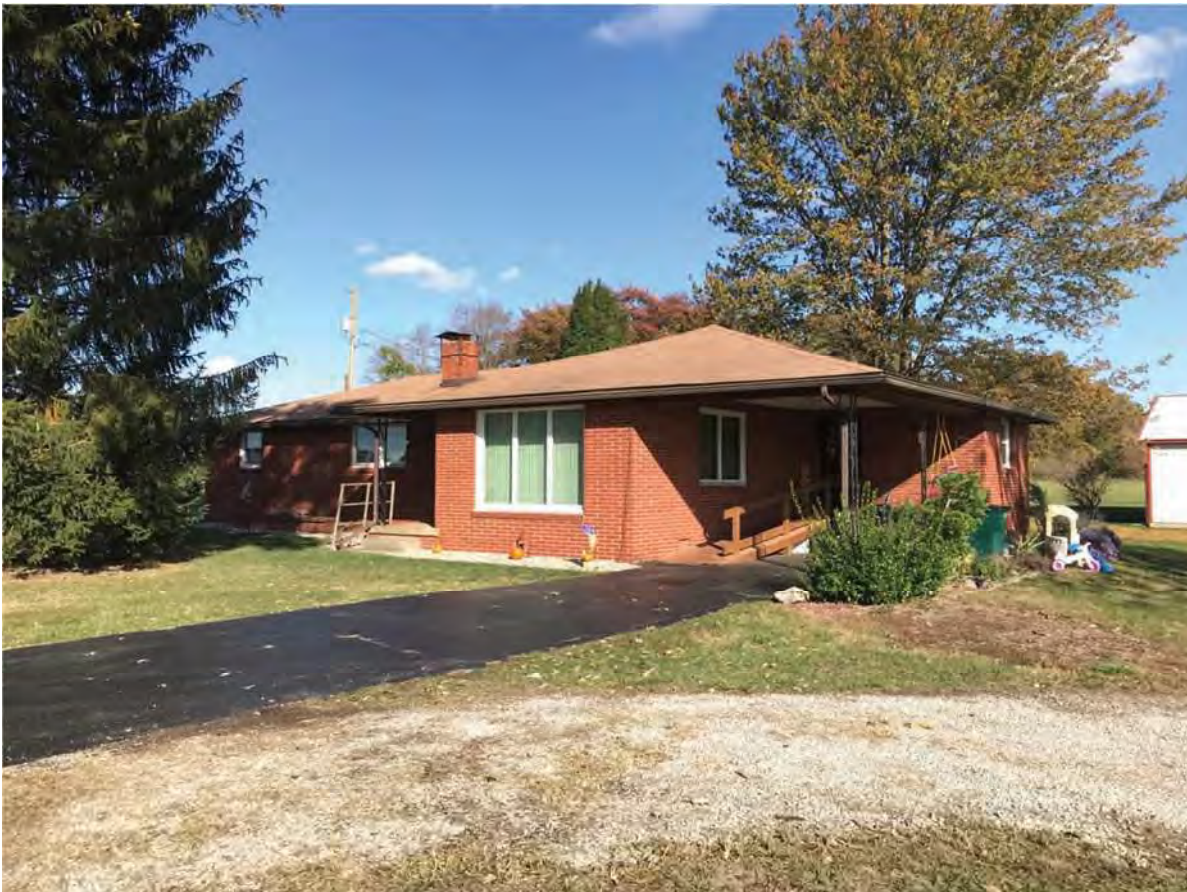
32. Looking NW at IHSSI #143-578-15032, Contributing, 1678 SR 56
