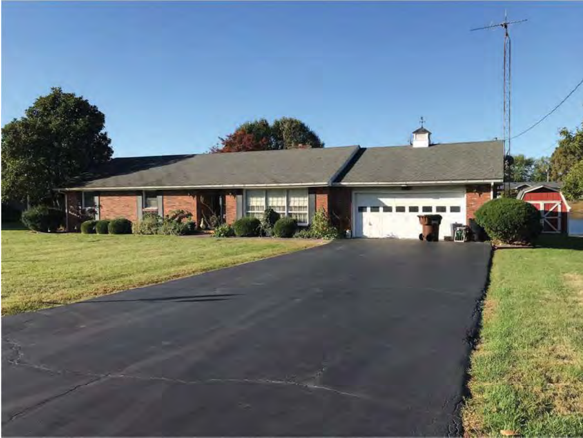
41. Looking SW outside APE in Lake Hosea Subdivision at Lochmueller #11, Contributing, 2153 Bob White Drive
