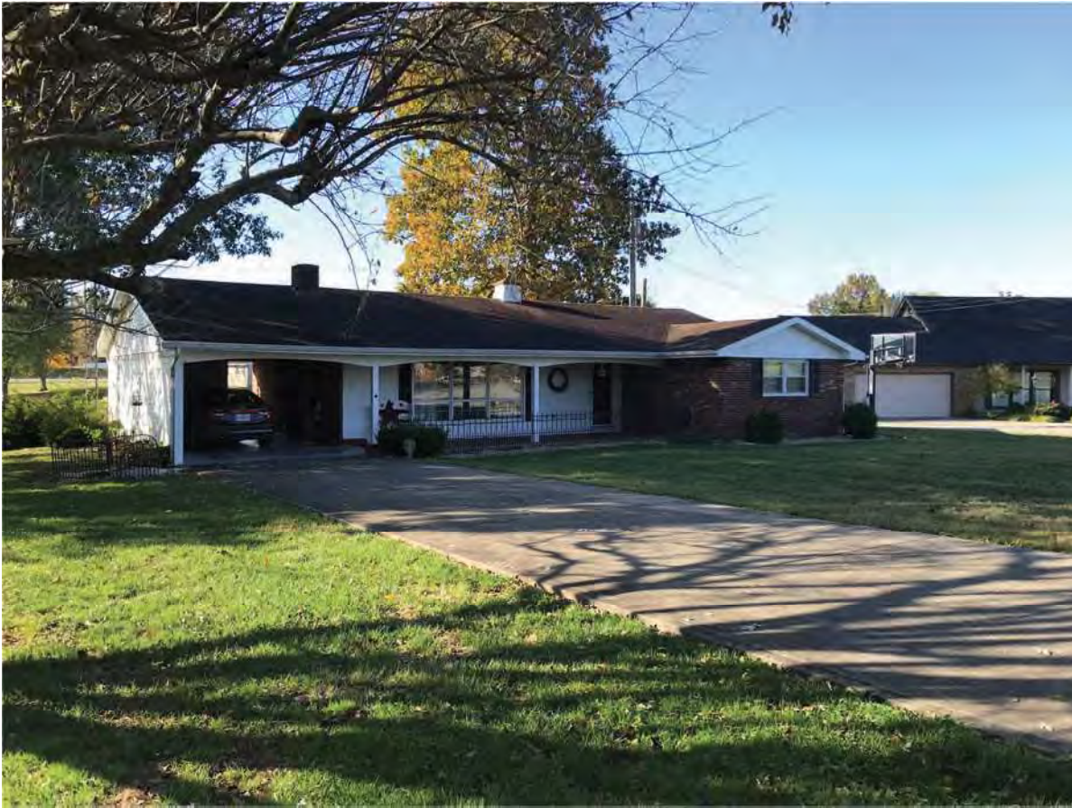
39. Looking SW outside APE in Lake Hosea Subdivision at Lochmueller #9, Contributing, 2137 Bob White Drive
