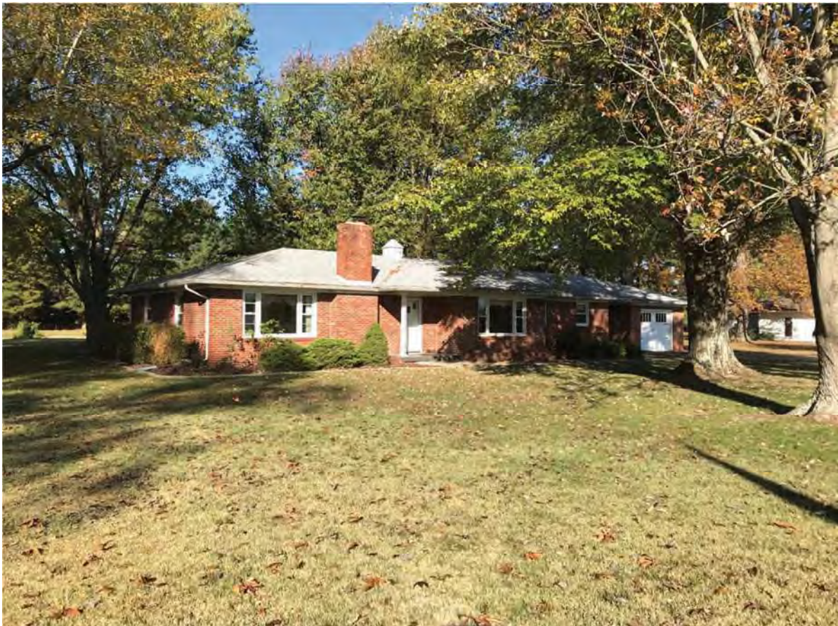
24. Looking NW at Lochmueller #3, Contributing, 462 S. Boatman Road
