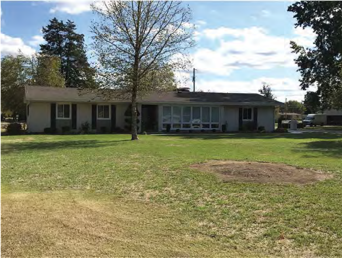
63. Looking E outside APE in Lake Hosea Subdivision at Lochmueller #27, Contributing, 453 S. Whippoorwill Lane
