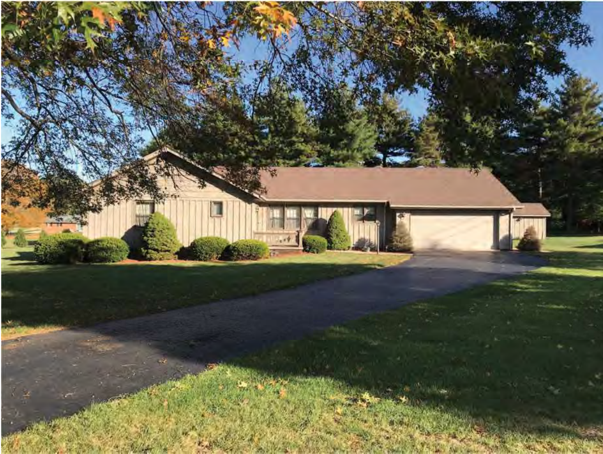
53. Looking N outside APE in Lake Hosea Subdivision at Lochmueller #22, Contributing, 2257 Bob White Drive
