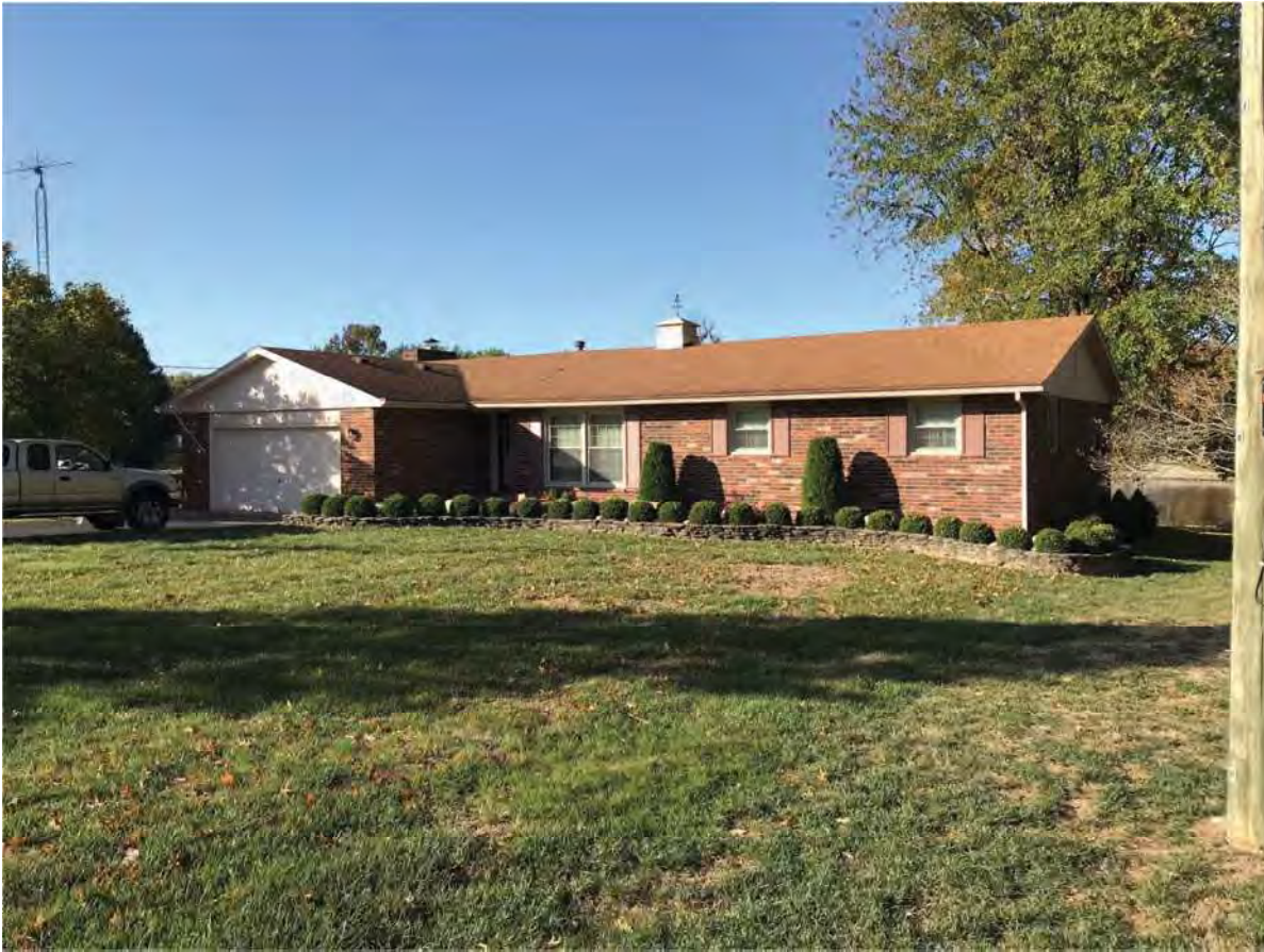
43. Looking SW outside APE in Lake Hosea Subdivision at Lochmueller #13, Contributing, 2167 Bob White Drive
