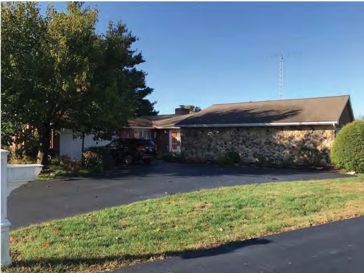
46. Looking SW outside APE in Lake Hosea Subdivision at Lochmueller #15, Contributing, 2181 Bob White Drive
