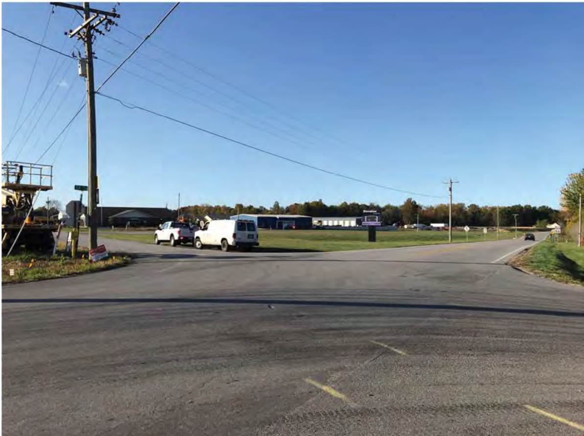
6. Looking SSW at the intersection of SR 56 and Boatman Road
