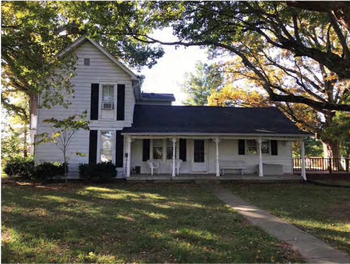
17. Looking S at IHSSI #143-578-15036, Contributing, 518 Boatman Road
