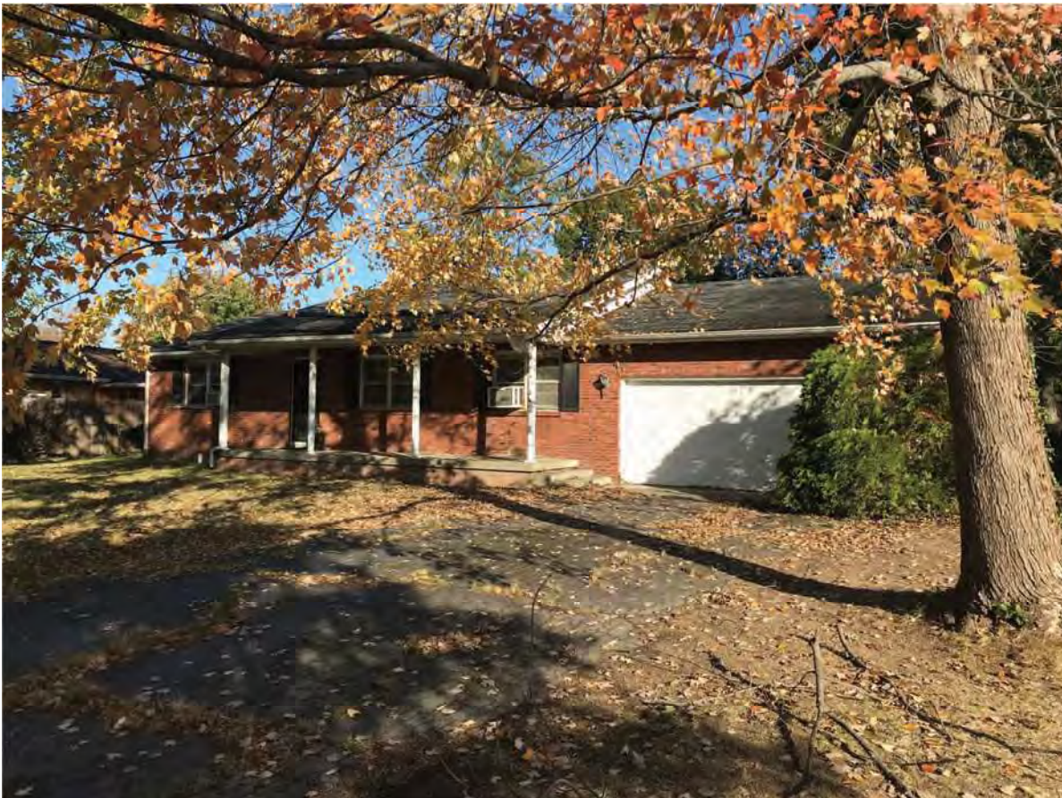
38. Looking NW outside APE in Lake Hosea Subdivision at Lochmueller #8, Contributing, 2124 Bob White Drive
