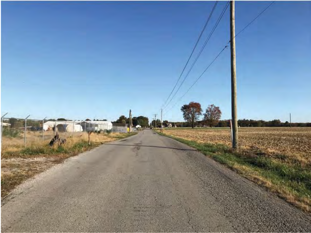
11. Looking N from S end of APE on Boatman Road
