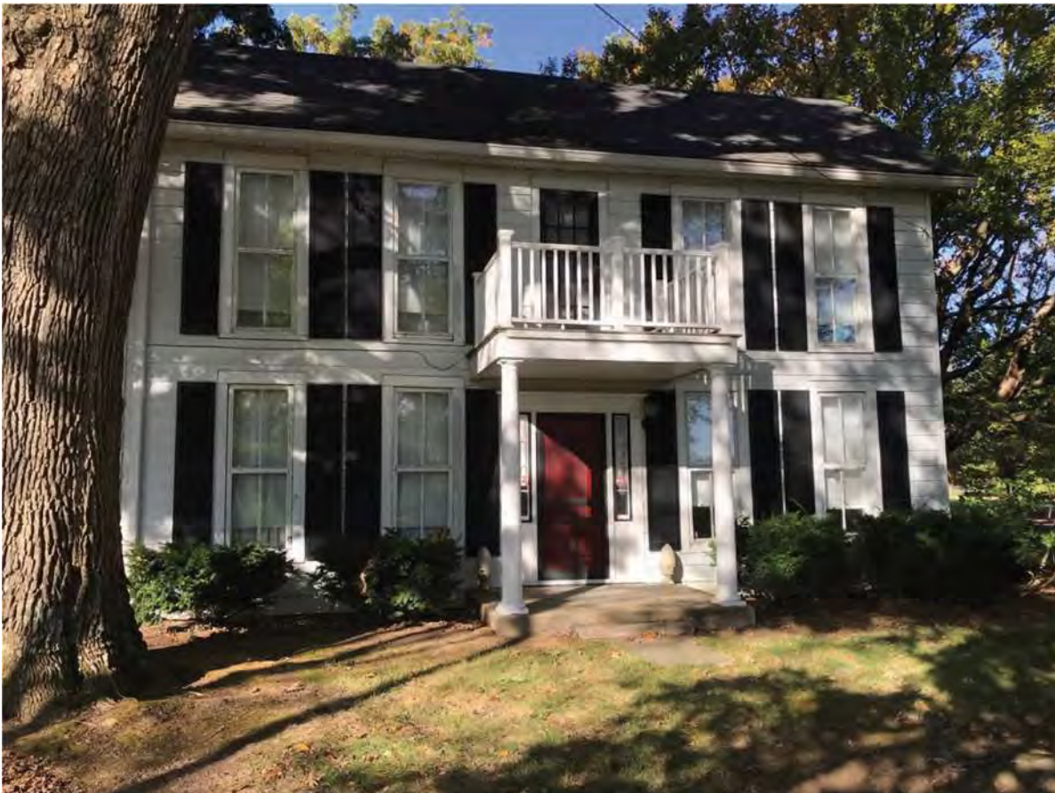
16. Looking W at IHSSI #143-578-15036, Contributing, 518 Boatman Road
