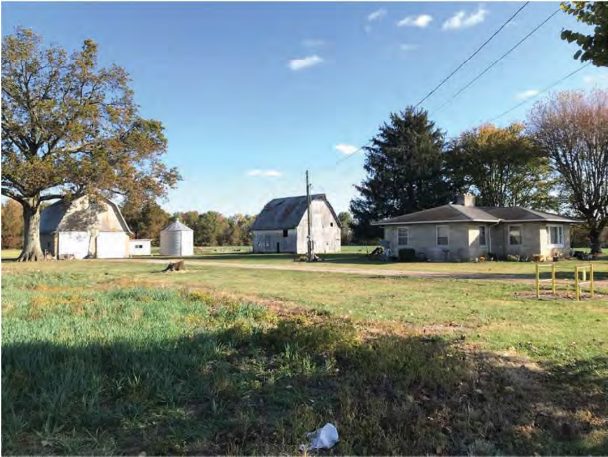
27. Looking NE at IHSSI #143-578-15033, Contributing, 1872 Mount Drive
