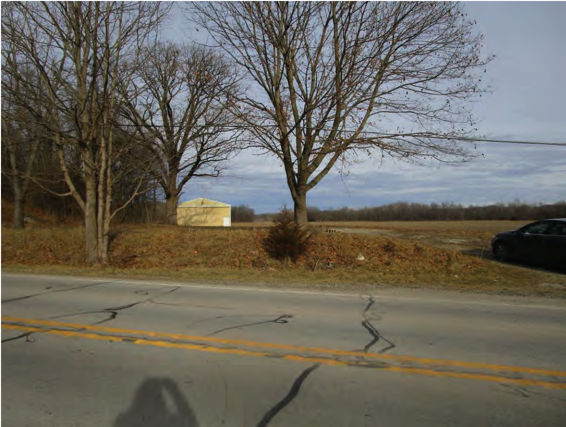
Photo 2 – Looking north toward remaining outbuilding at 225 E SR 163
