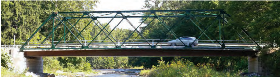
Forest Home Drive bridge, Ithaca, NY
