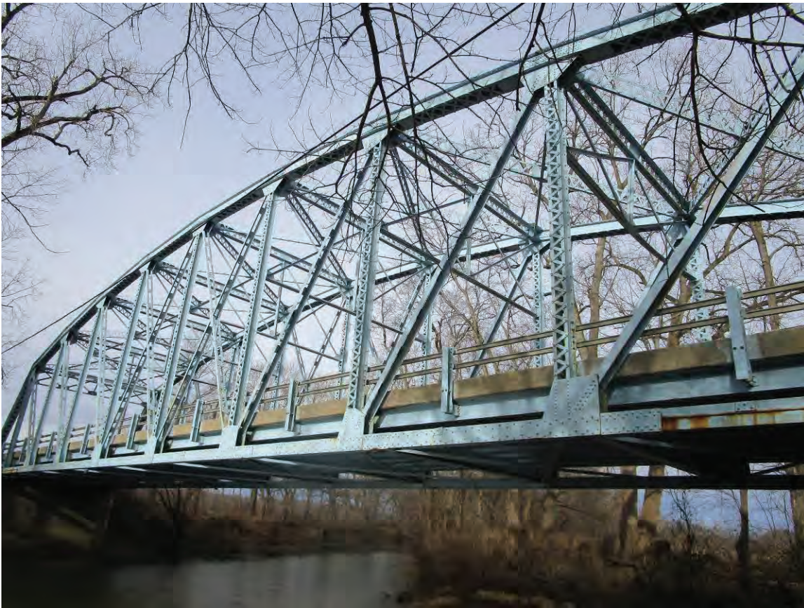
Photo 5 – Looking northwest at bridge
