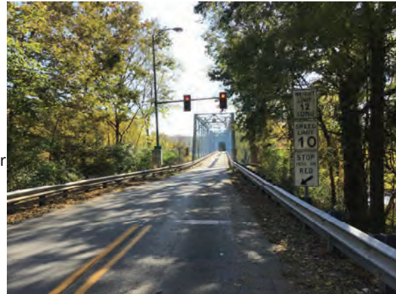
SR 225 over Wabash River
