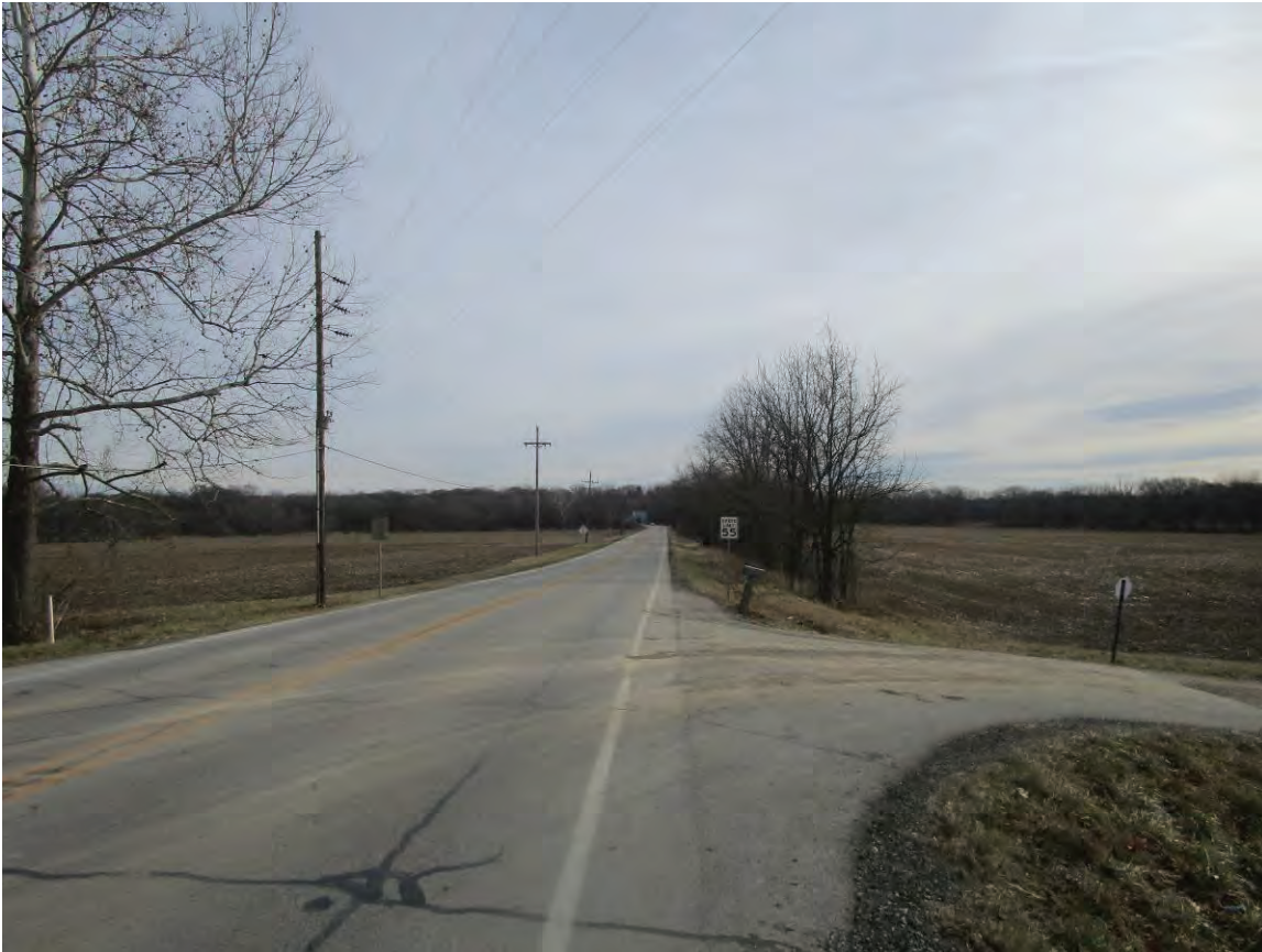
Photo 1 - Looking east toward bridge from S. Gorton Rd.
