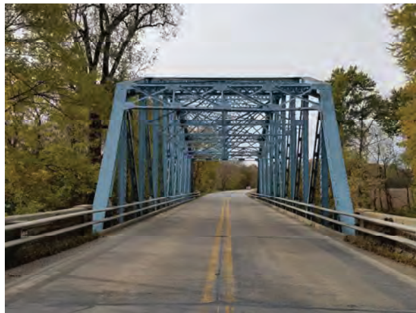
SR 163 over Brouilletts Creek
