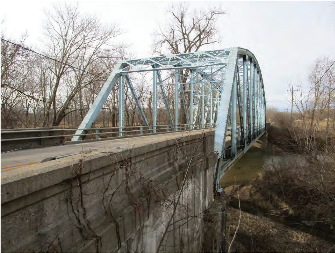
Photo 4 – Looking southwest at bridge
