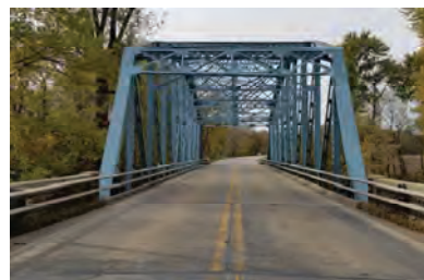
SR 163 over Brouilletts Creek
