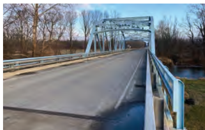
SR 75 over Wildcat Creek
