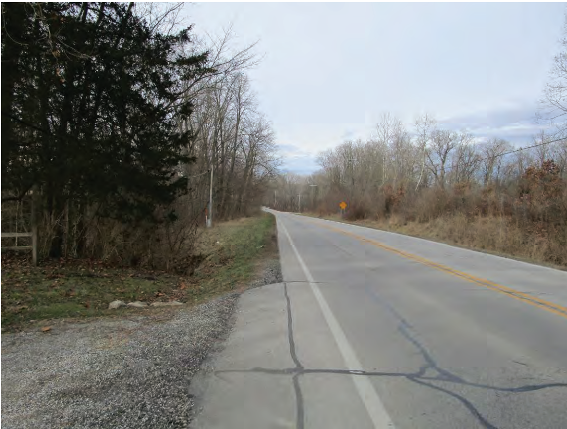
Photo 7 – Looking west toward bridge from Spangler Cemetery entrance
