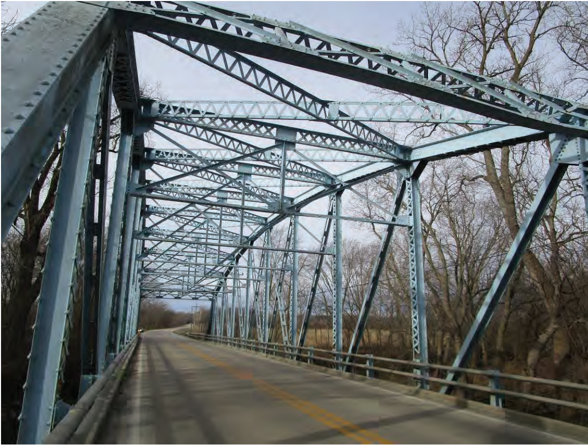
Photo 6 – Looking west through bridge
