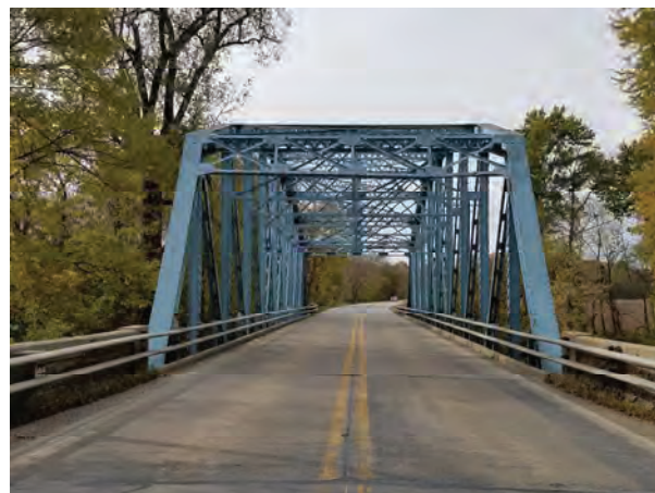
SR 163 over Brouilletts Creek
