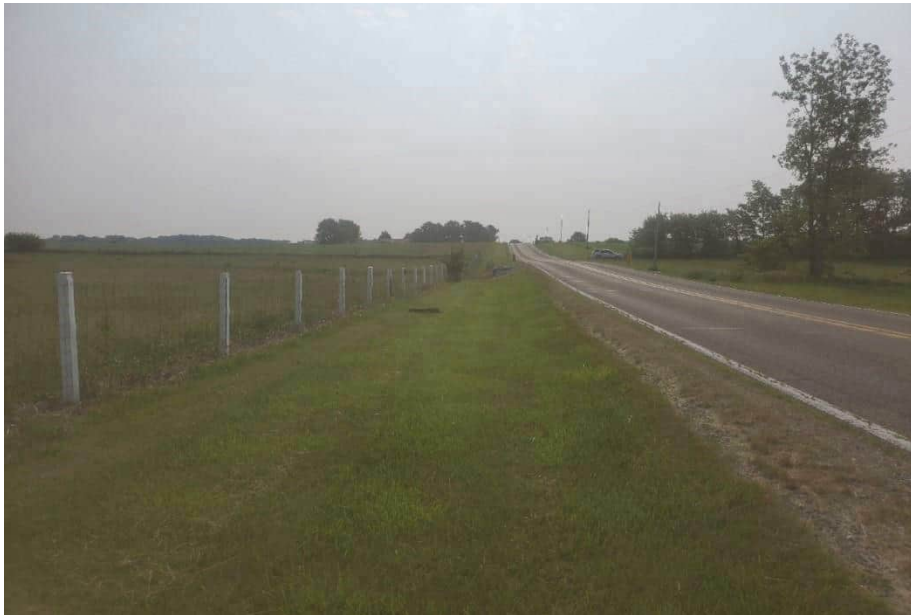
Photo 2. Facing east toward the project structure along north side of SR 32 from western terminus of the investigated area.
