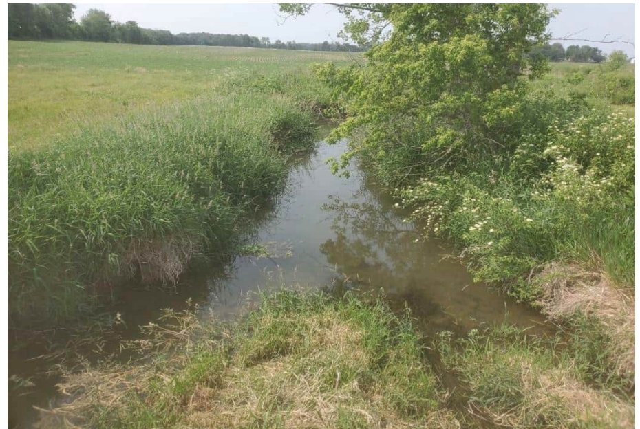
Photo 8. Facing south toward McFarland Ditch from the project structure (outlet), southside of SR 32.
