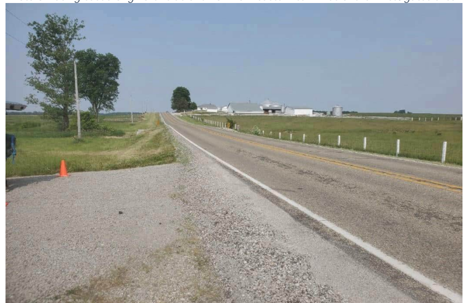
Photo 4. Facing west toward the project structure along south side of SR 32 from eastern terminus of the investigated area.
