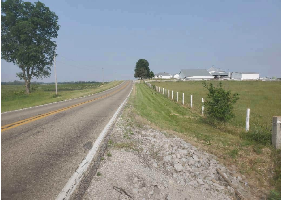
Photo 13. Facing east from the project structure along north side of SR 32.
