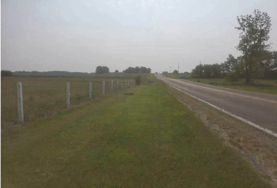
Photo 1. Facing east toward the project structure along north side of SR 32 from western terminus of the investigated area.
