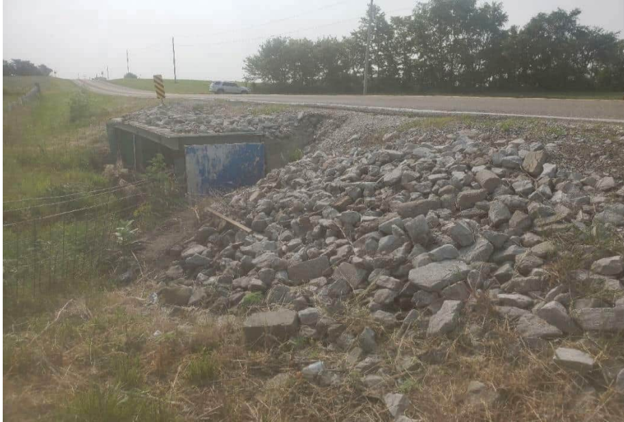
Photo 5. Facing southeast toward the project structure from north side of SR 32.
