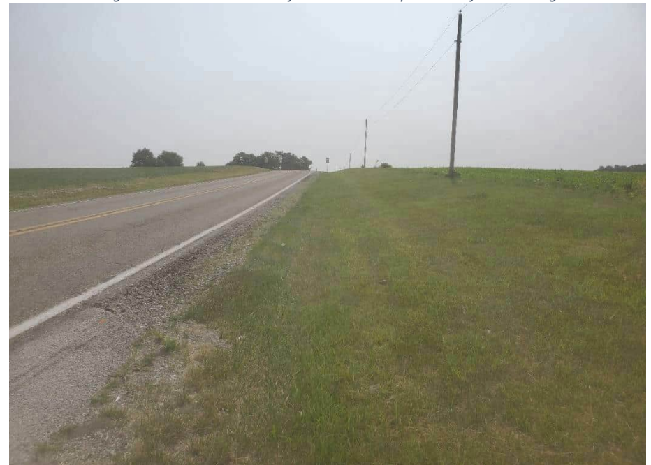
Photo 28. Facing east along south side of SR 32 from eastern terminus of the investigated area.
