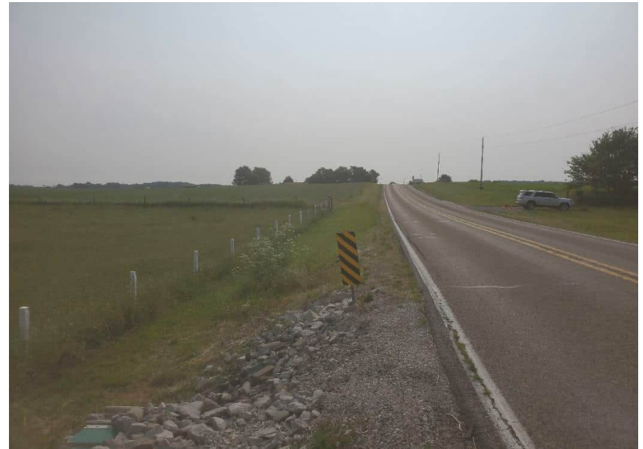
Photo 12. Facing east from the project structure along the north side of SR 32.
