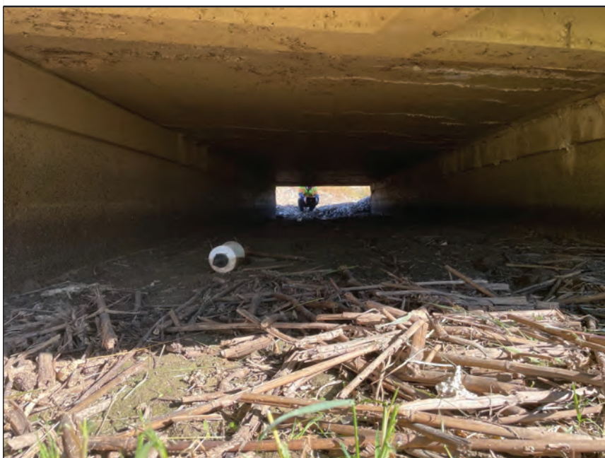
PHOTO #Culvert interior: South interior overall condition. Close spaced longitudinal cracking that runs full length with moderate to heavy efflorescence
