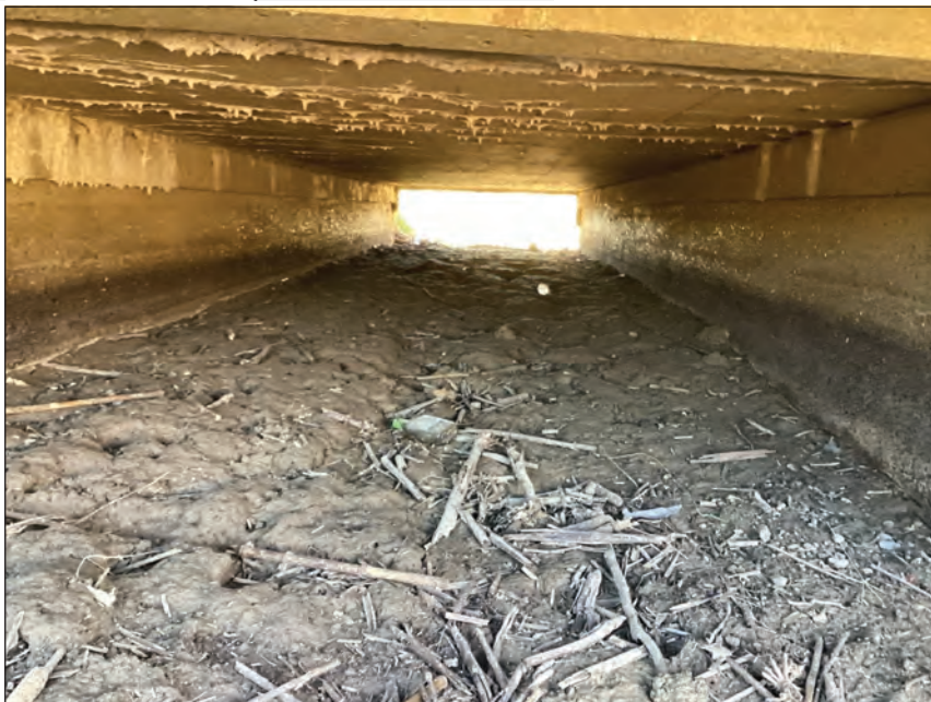
PHOTO #Culvert interior: North interior overall condition. Significant map cracking at north end of slab w/ heavy efflorescence. Minor width longitudinal cracking w/ moderate efflorescence throughout remainder of slab.
