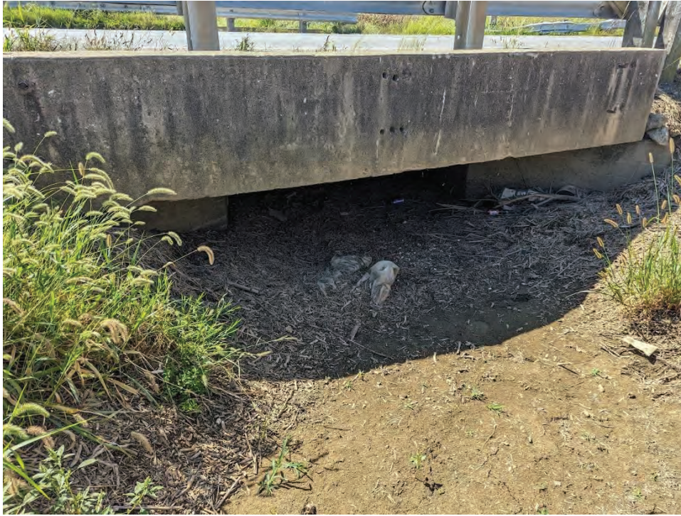
Photograph 43. View of UNT to Willow Pond Ditch with evidence of drift deposits and extreme sedimentation under SR 66 and CV 066-074-51.62, looking southwest.
