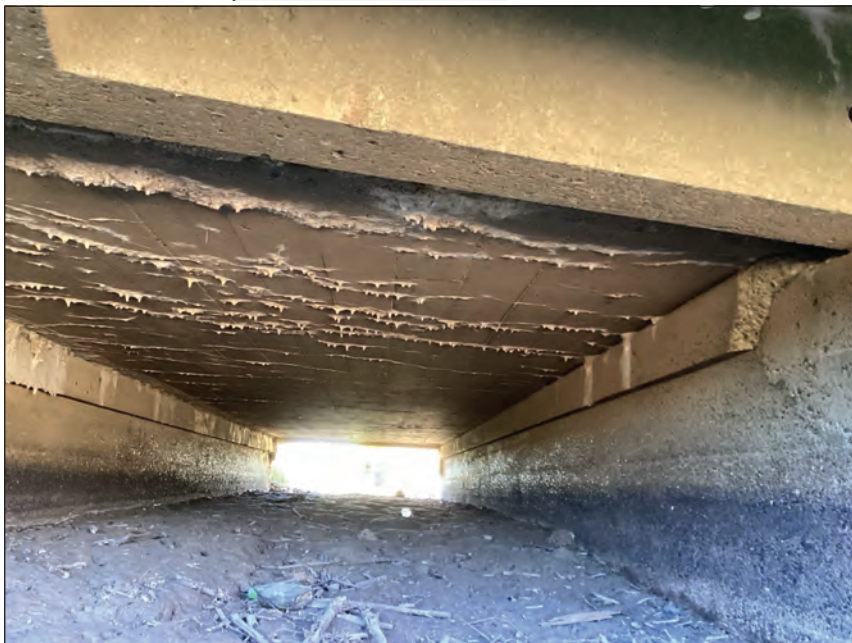
PHOTO #Original Slab.: Underside overall condition. Significant map cracking at north end of slab w/ heavy efflorescence. Minor width longitudinal cracking w/ moderate efflorescence throughout remainder of slab.
