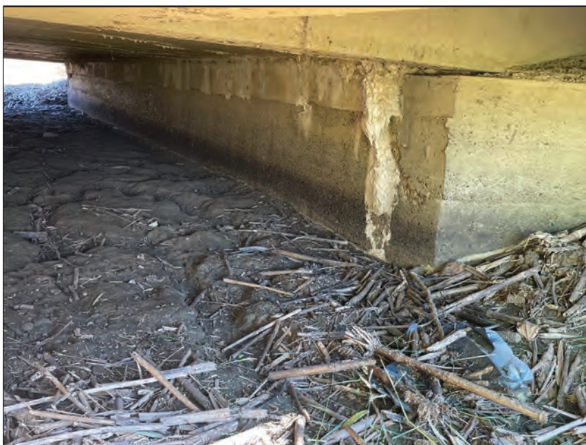
PHOTO #Abutment 2: Abutment 2 overall condition. Moderate scaling and leaching on Abutment 2.
