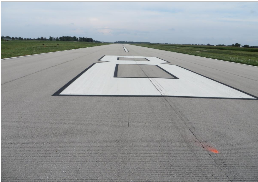
Figure 2-5. Typical Good AC Pavement (Feature 6105)
