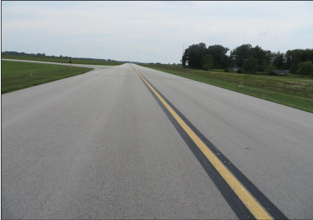
Figure 2-4. Typical Good AC Pavement (Feature 105)
