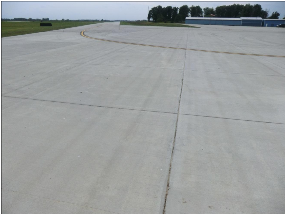
Figure 2-3. Typical Good PCC Pavement (Feature 3105)
