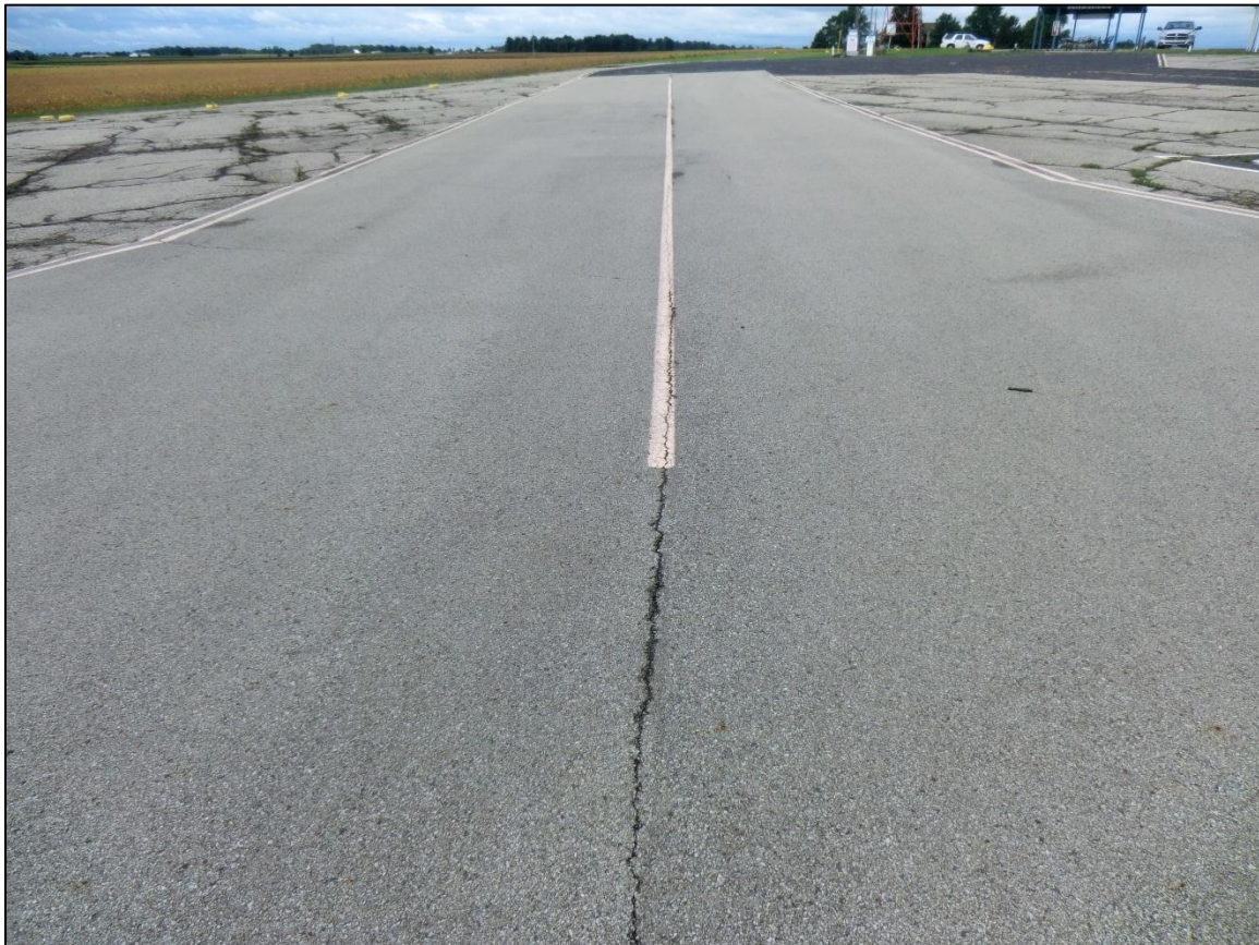
Figure 2-3. Typical Good AC Pavement (Feature 4010)
