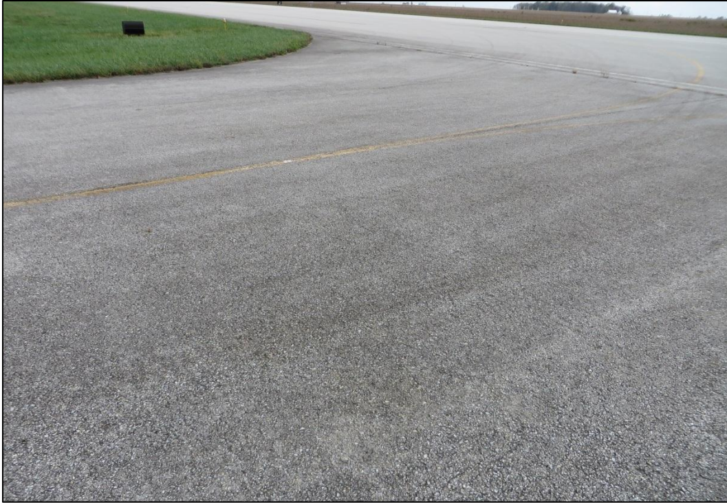
Figure 2-4. Typical Good AC Pavement (Feature 215)
