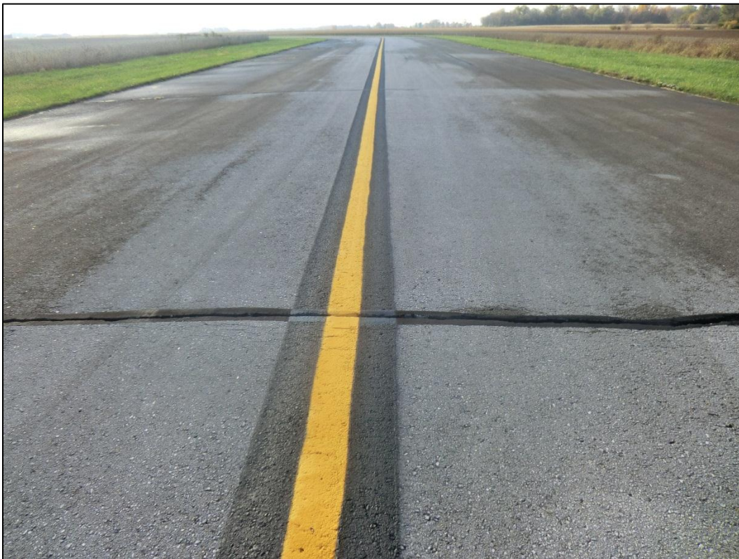
Figure 2-5. Typical Satisfactory AC Pavement (Feature 110)
