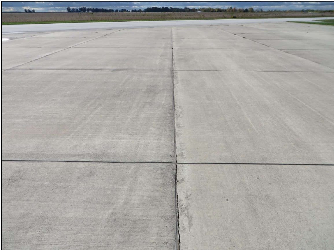
Figure 2-3. Typical Good PCC Pavement (Feature 3105)
