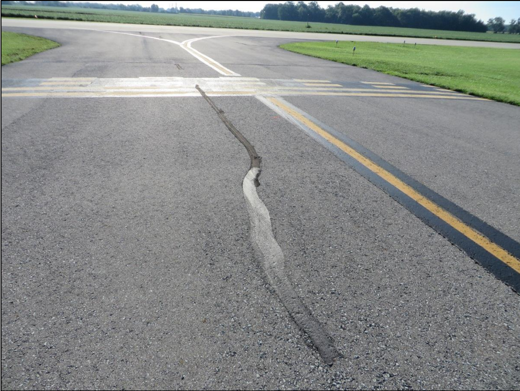
Figure 2-4. Typical Good AC Pavement (Feature 140)
