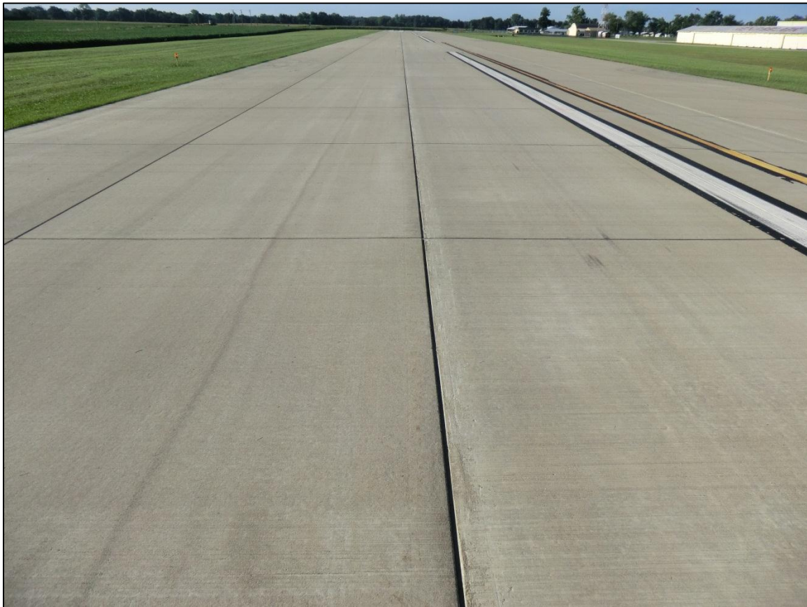
Figure 2-3. Typical Good PCC Pavement (Feature 6105)
