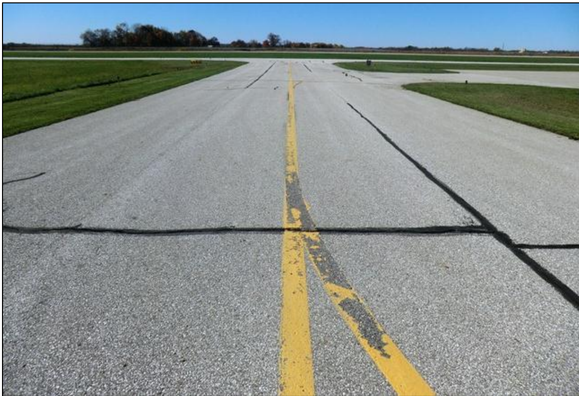
Figure 2-5. Typical Satisfactory AC Pavement (Feature 210)
