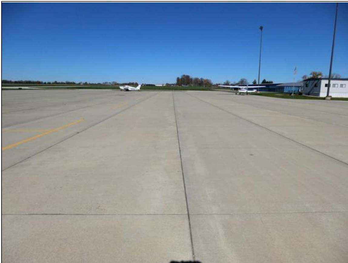
Figure 2-3. Typical Good PCC Pavement (Feature 4105)
