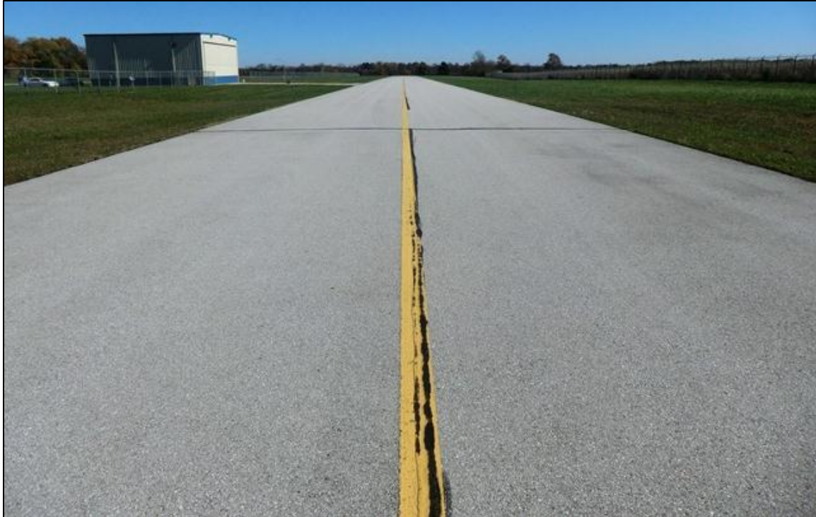
Figure 2-4. Typical Satisfactory AC Pavement (Feature 205)
