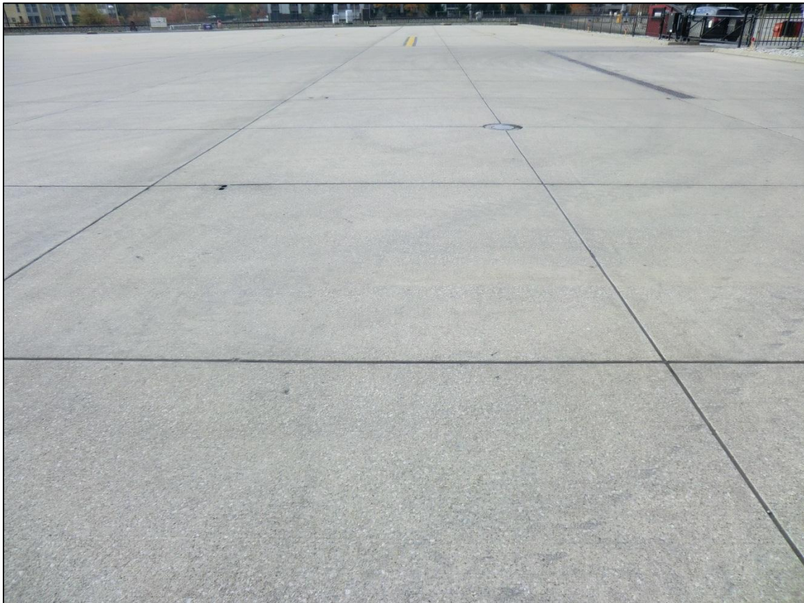
Figure 2-3. Typical Good PCC Pavement (Feature 3015)
