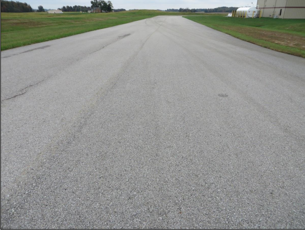
Figure 2-4. Typical Good AC Pavement (Feature 410)
