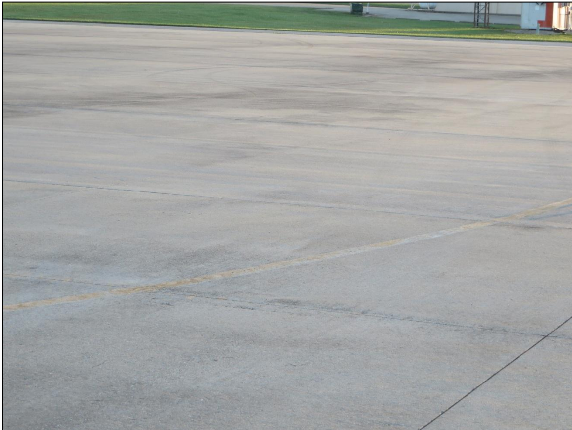
Figure 2-3. Typical Good PCC Pavement (Feature 3205)
