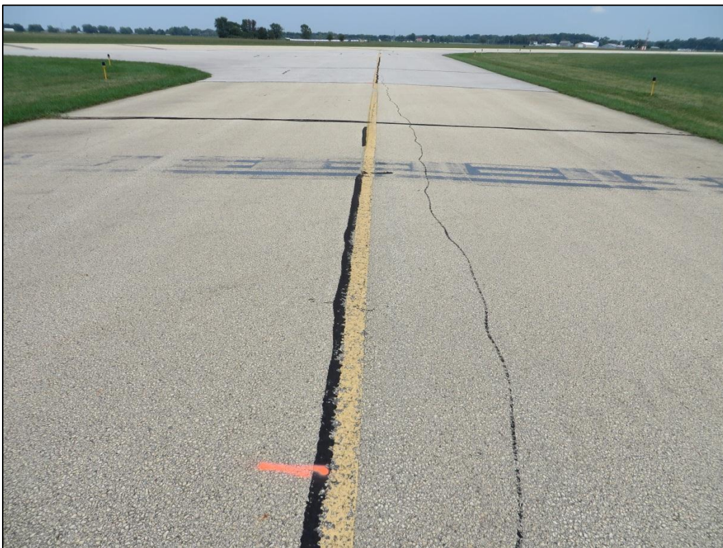
Figure 2-5. Typical Satisfactory AC Pavement (Feature 110)
