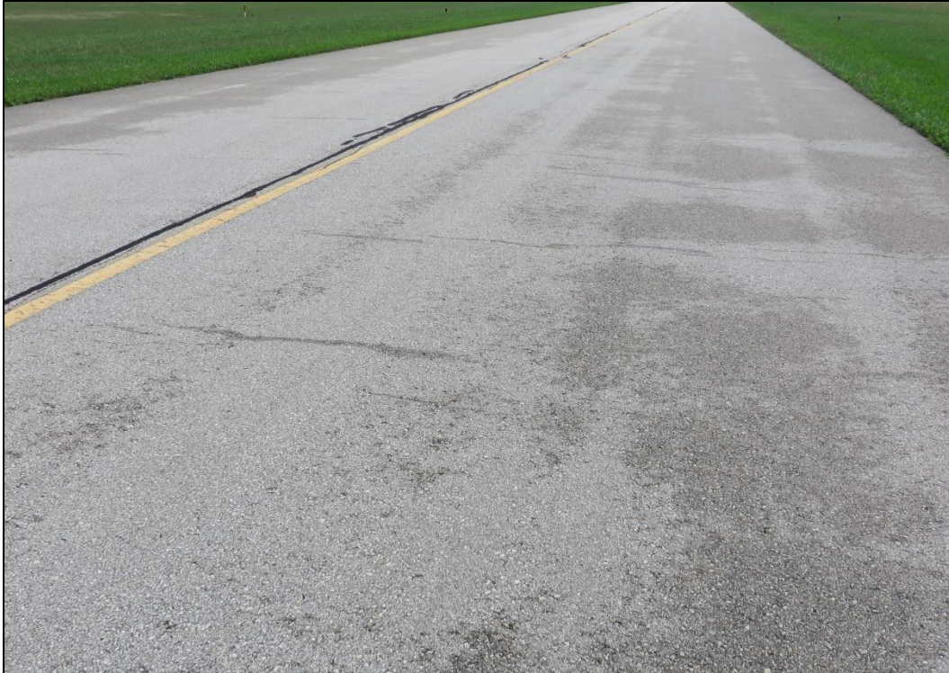
Figure 2-4. Typical Good AC Pavement (Feature 225)
