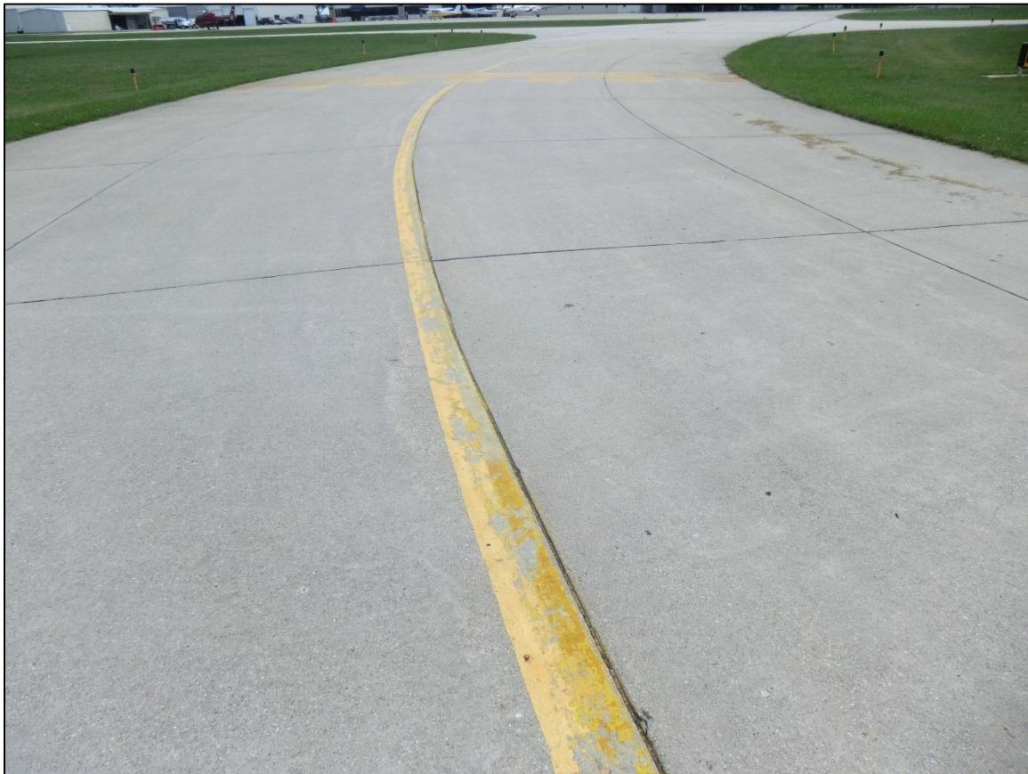
Figure 2-3. Typical Good PCC Pavement (Feature 510)
