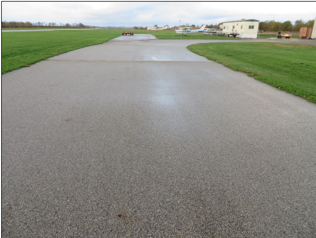
Figure 2-3. Typical Satisfactory AC Pavement (Feature 4115)
