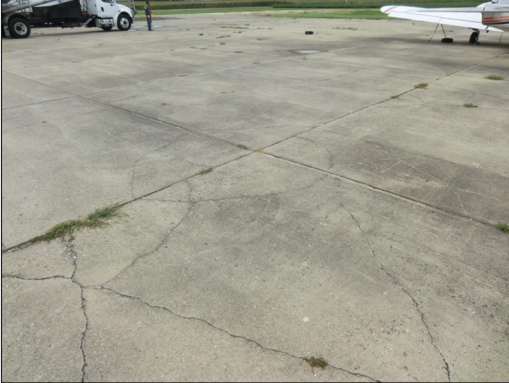
Figure 2-4. Typical Ramp PCC Pavement (Feature 3105)
