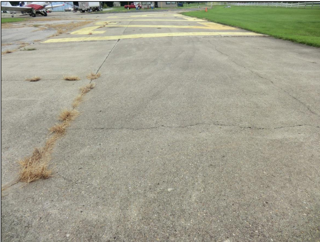
Figure 2-5. Typical Taxiway PCC Pavement (Feature 105)
