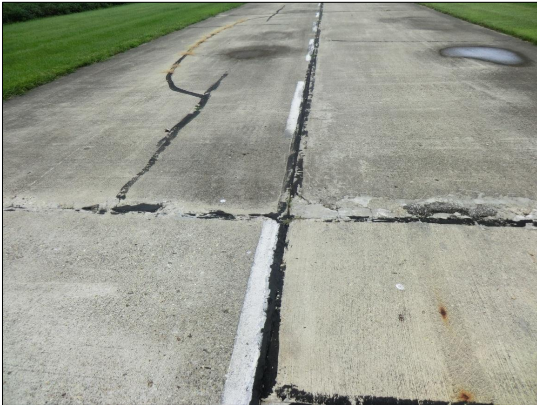
Figure 2-3. Typical Runway PCC Pavement (Feature 6105)
