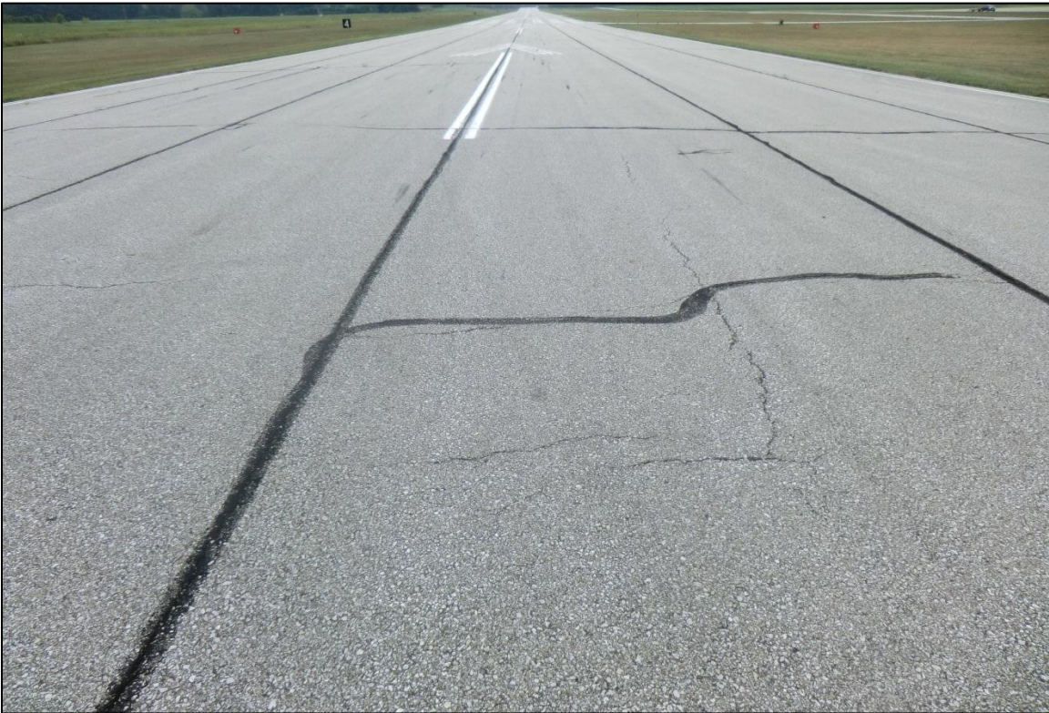
Figure 2-5. Typical Fair AC Pavement (Feature 6105)
