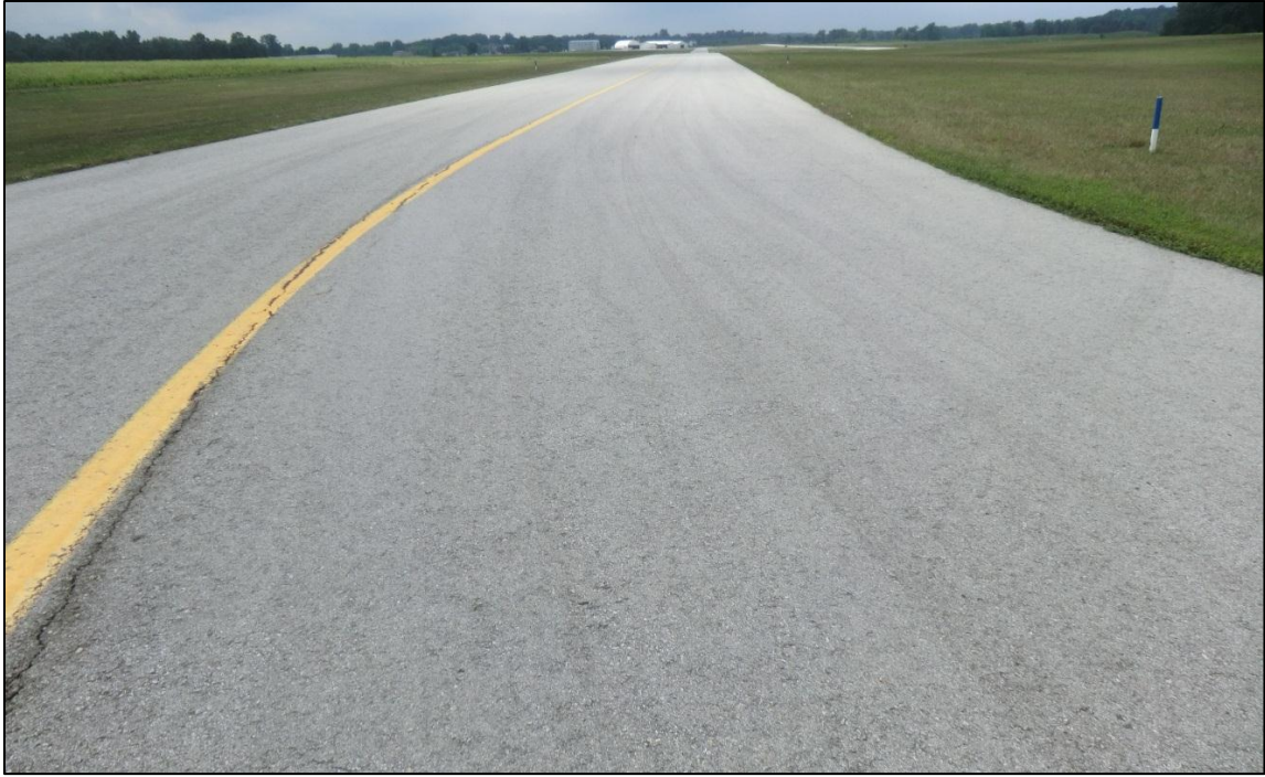
Figure 2-4. Typical Good AC Pavement (Feature 110)
