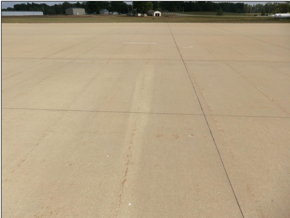
Figure 2-3. Typical Good PCC Pavement (Feature 4105)
