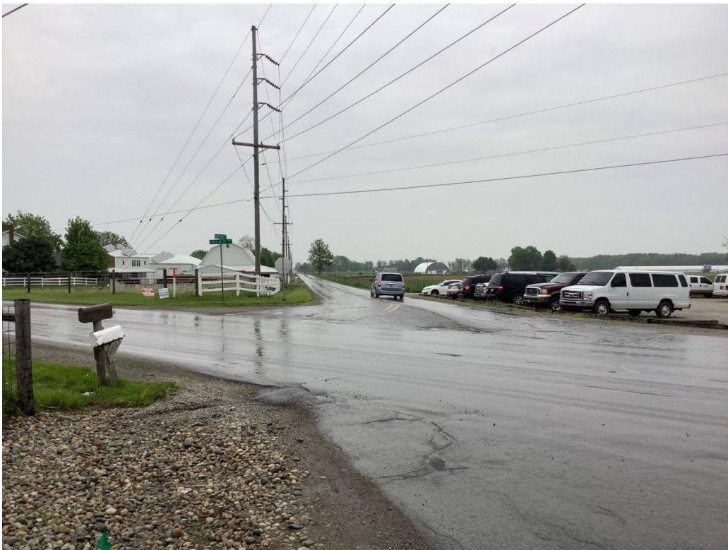
Figure 4-10 Overview of the Intersection of SR 37 and Notestine Road, facing east.
