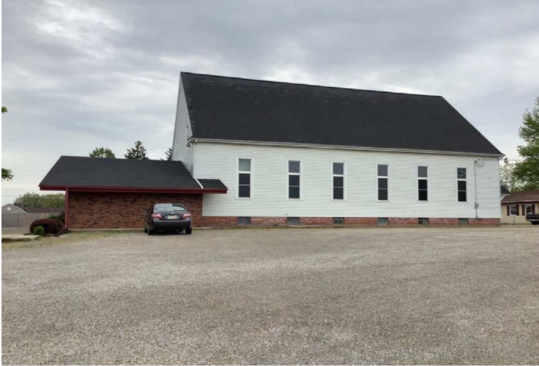
Figure 4-3 View of Non-Contributing Resource at 10835 Cuba Road, looking west.
