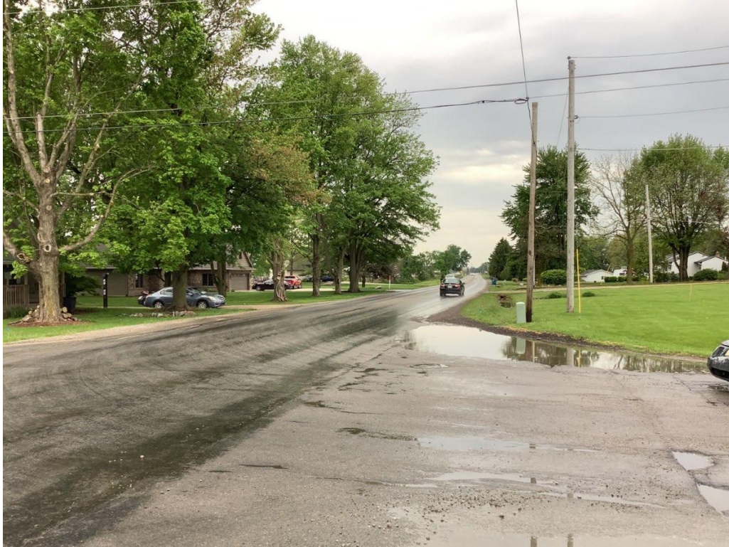
Figure 4-9 Overview of the Intersection of SR 37 and Thimlar Road, facing southwest.
