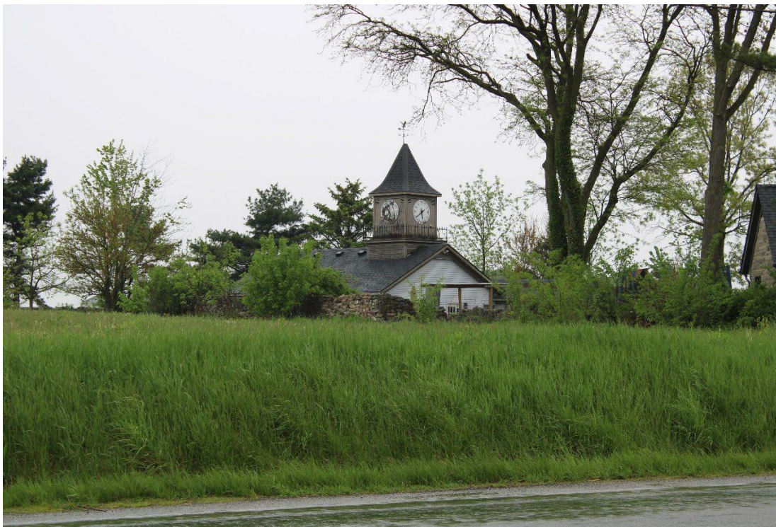
Figure 4-2 View of Ancillary Building, Eligible Resource at 16029 SR 37, looking southwest.
