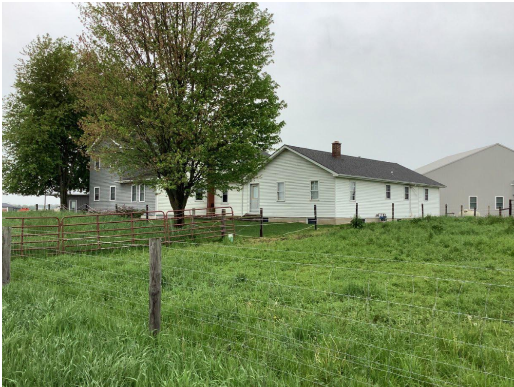
Figure 4-8 Overview of Non-Contributing Resource and Ancillary Buildings at 15525 SR 37, facing northwest.
