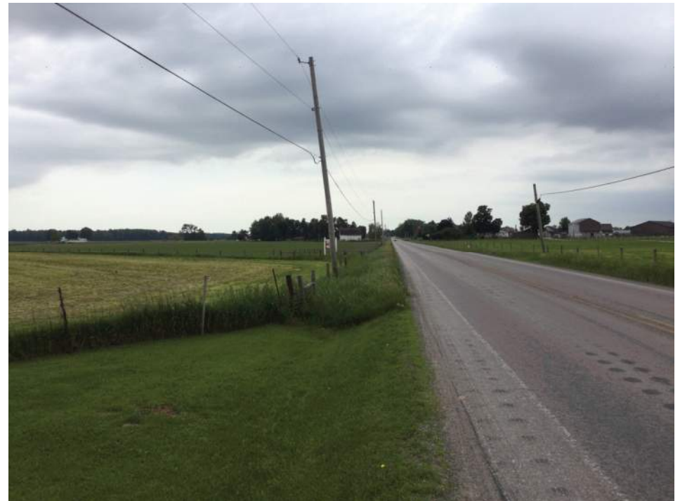
8. Looking southwest along the eastern side of SR 37
