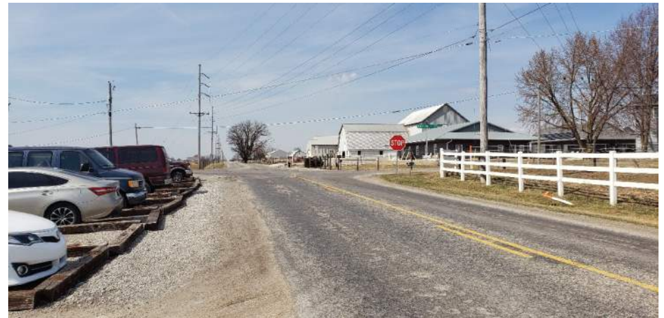
16. Looking west along Notestine Road toward the intersection
