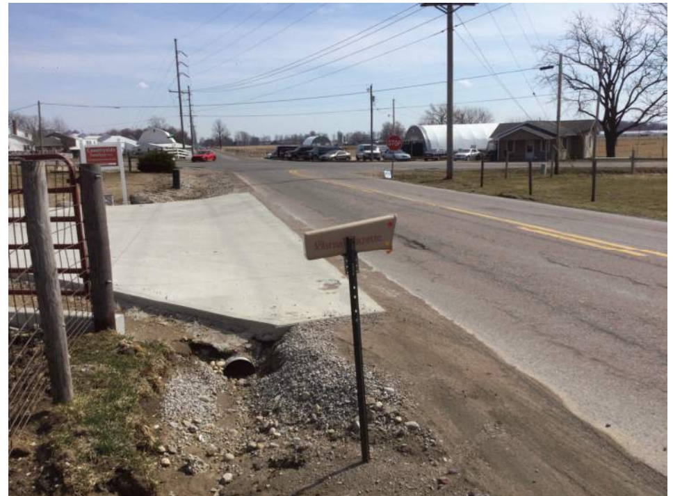
4. Looking southeast at the SR 37 and Notestine Road intersection
