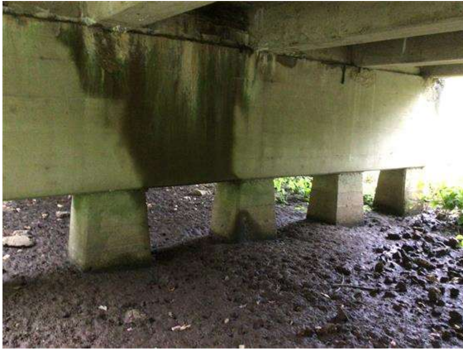
PHOTO 23 Condition Description Pier 8
