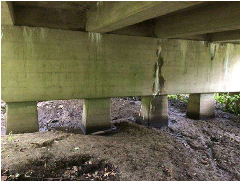
PHOTO 12 Condition Description Pier 5
