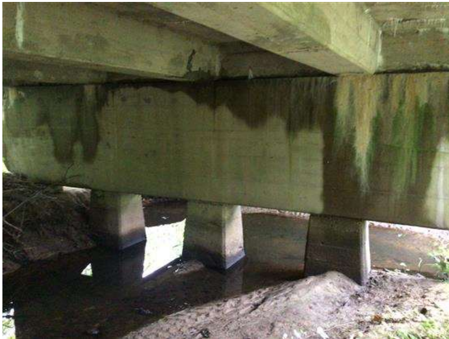
PHOTO 6 Condition Description Pier 3
