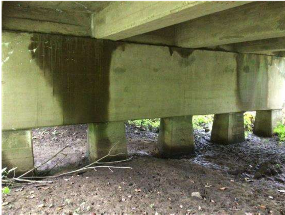
PHOTO 11 Condition Description Pier 6
