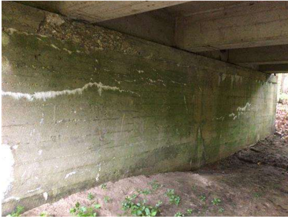
PHOTO 3 Condition Description Abutment 1 looking north
