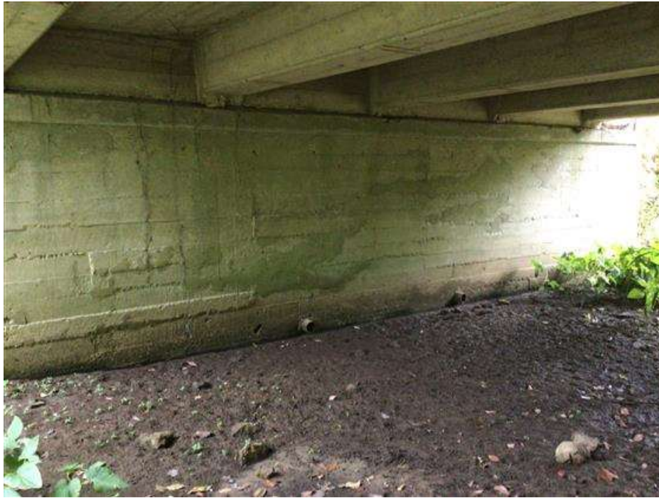
PHOTO 19 Condition Description Abutment 9
