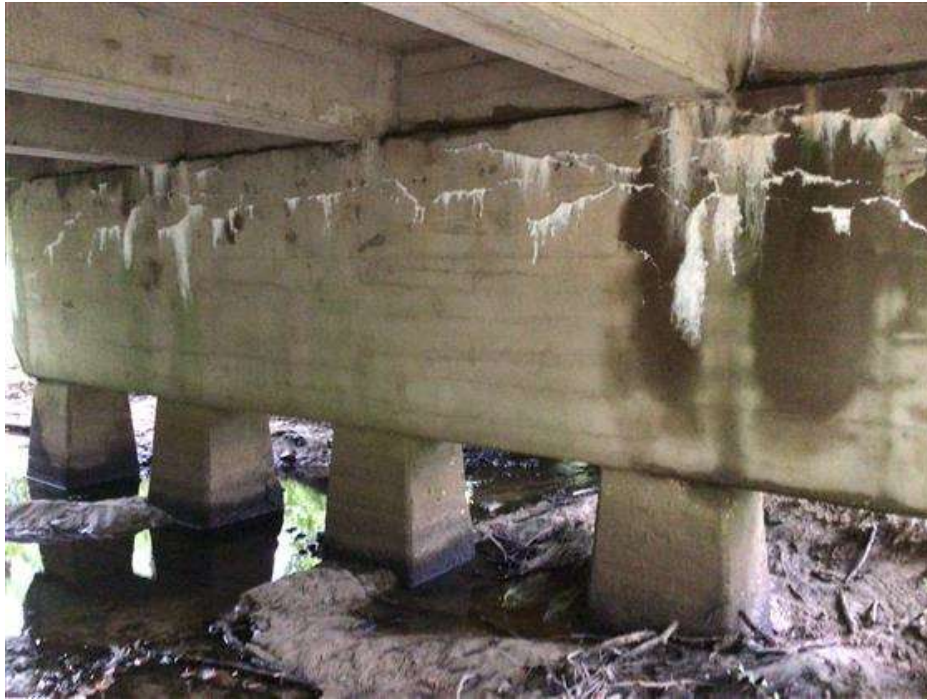
PHOTO 5 Condition Description Pier 2
