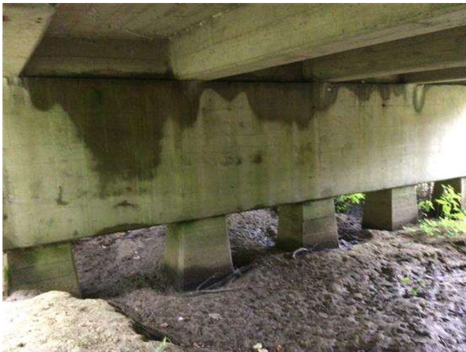
PHOTO 4 Condition Description Pier 4
