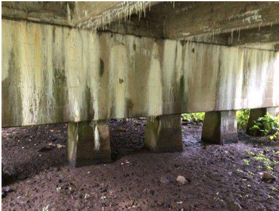
PHOTO 16 Condition Description Pier 7
