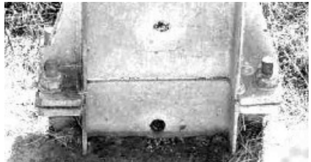
Figure 2-4 Structural Steel Post on a Breakaway Stud
