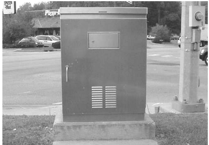
Figure 1-8 Traffic Signal Controller
