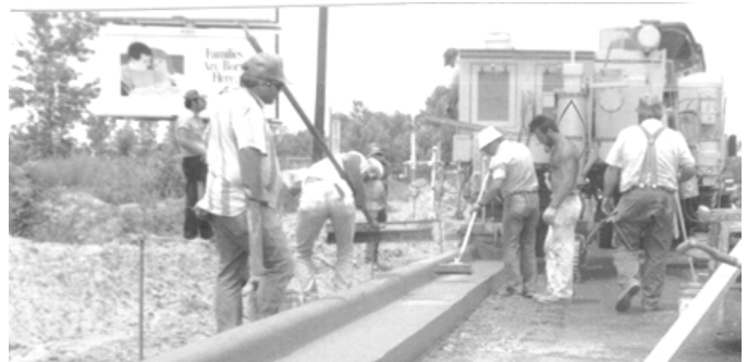
Figure 5-1 Combined Curb and Gutter
