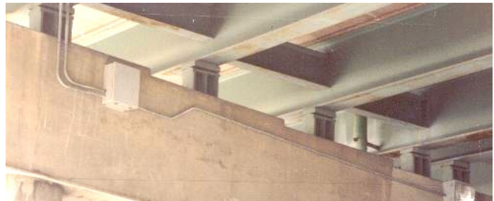
Figure 4-3 Acceptable Underpass Circuitry
