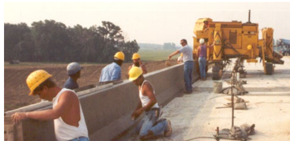
Figure 9-1 Slip-forming a Concrete Barrier
