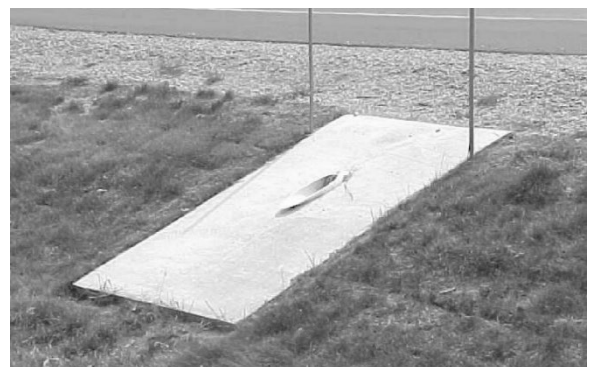
Figure 10-5 Underdrain Outlet Protector
