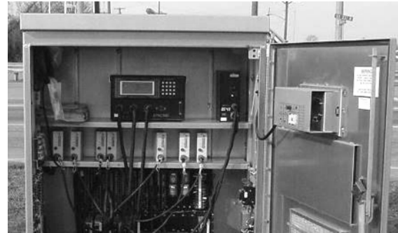
Figure 1-9 Controller Cabinet Wiring
