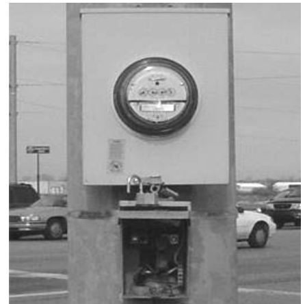
Figure 1-7 Electrical Service and Entrance Switch
