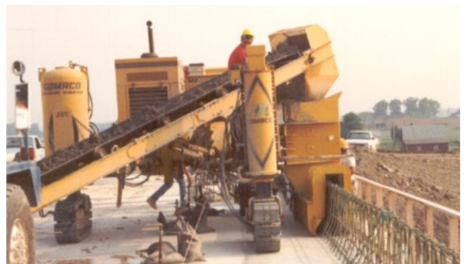
Figure 9-3 Slipform Machine
