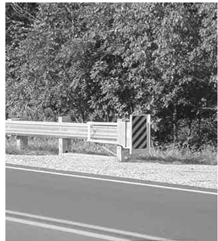
Figure 11-4 Guardrail End Treatment
