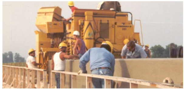
Figure 9-2 Hand-finishing Concrete Barrier
