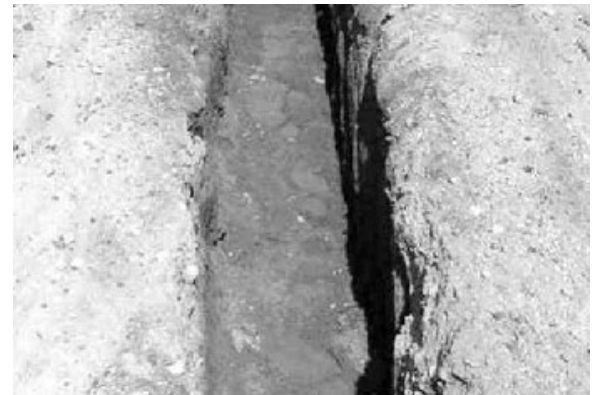
Figure 10-3 Underdrain Trench
