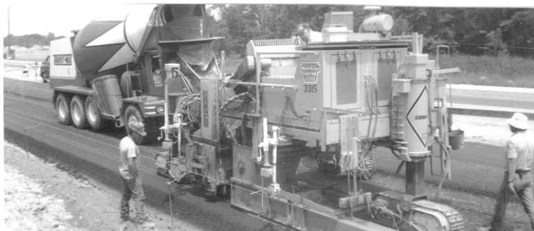
Figure 5-4 Concrete Curb Machine
