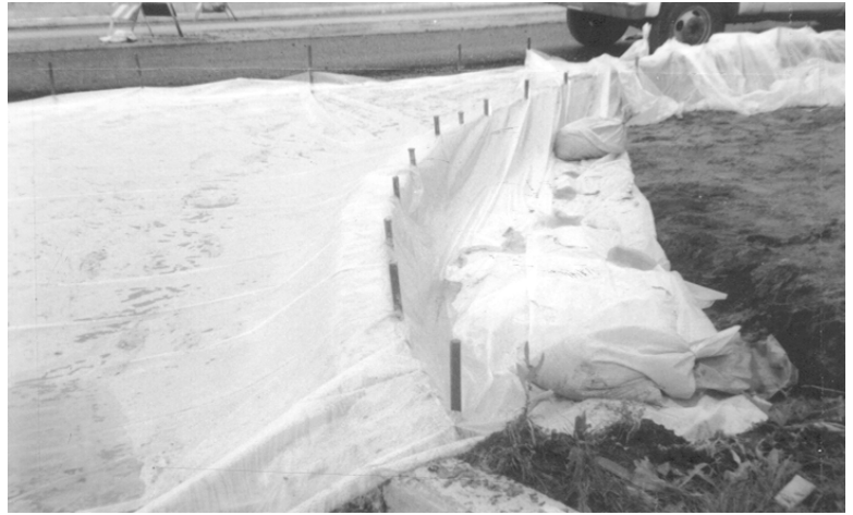
Figure 7-4 Curing with Plastic Sheeting
