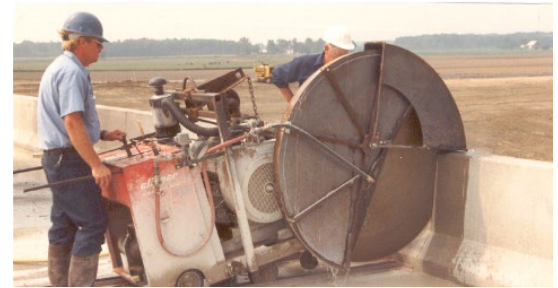
Figure 9-4 Sawing Concrete Joint
