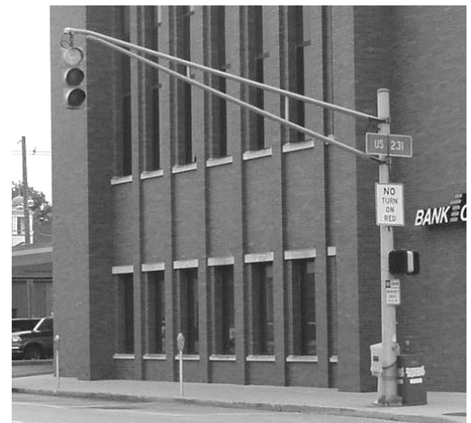
Figure 1-6 Pole and Mast Arm
