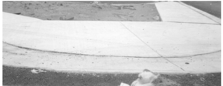
Figure 6-2 Contraction and Preformed Joints
