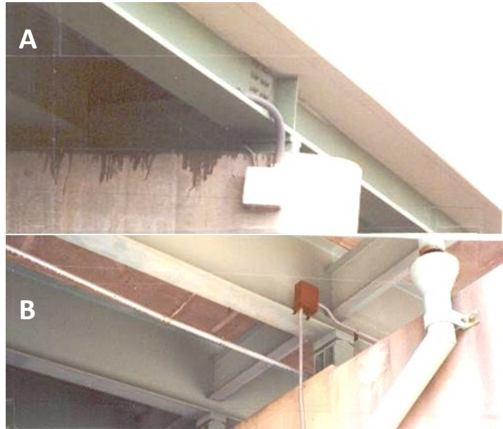
Figure 4-2 Errors in Underpass Breaker Box Installation (a) Top entry is not allowed (b) 2" conduit not attached at 4' intervals
