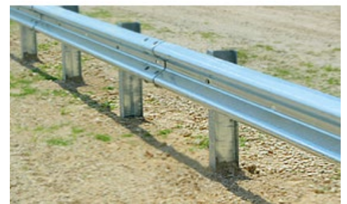
Figure 11-2 MGS W-Beam Midspan
