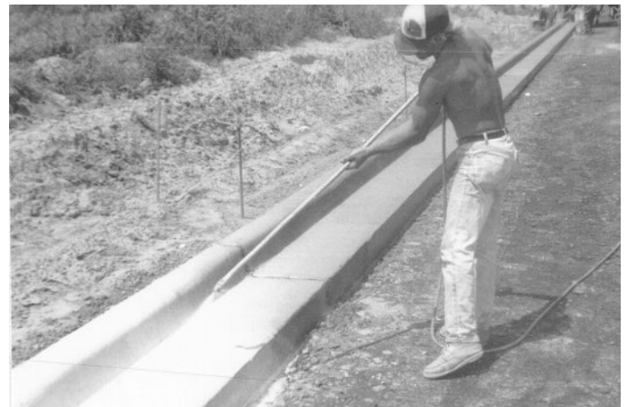
Figure 5-5 Applying Curing Compound
