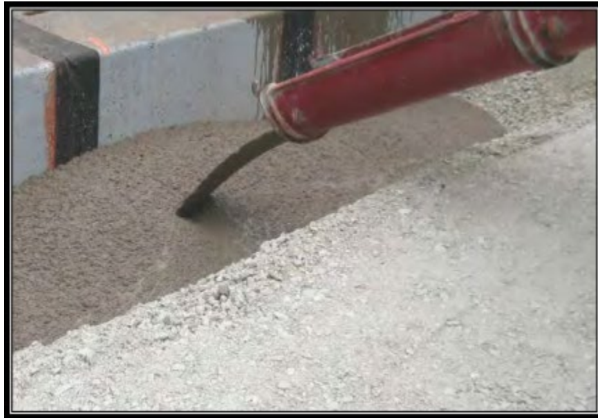
Figure 12-12-1 Flowable Backfill for Box
