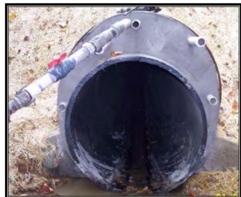
Figure 13-6 Grouting Pipe Liner
