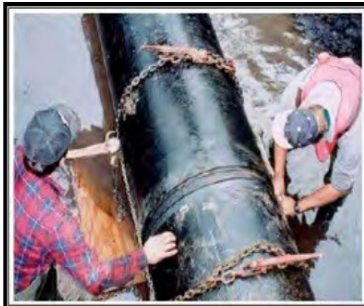
Figure 13-3 Jointing a Liner
