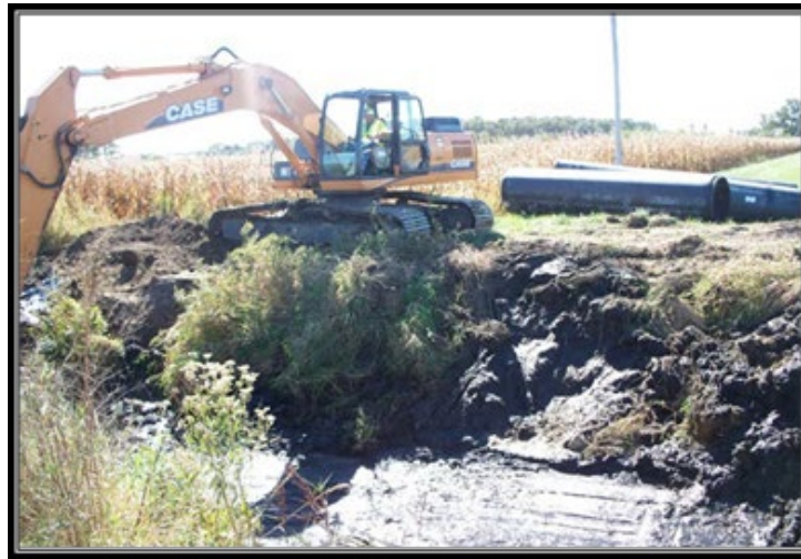
Figure 9-2 Figure 9-2 Removing Unsuitable Material
