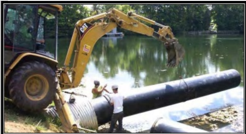
Figure 13-4 Pushing Pipe Liner over Water
