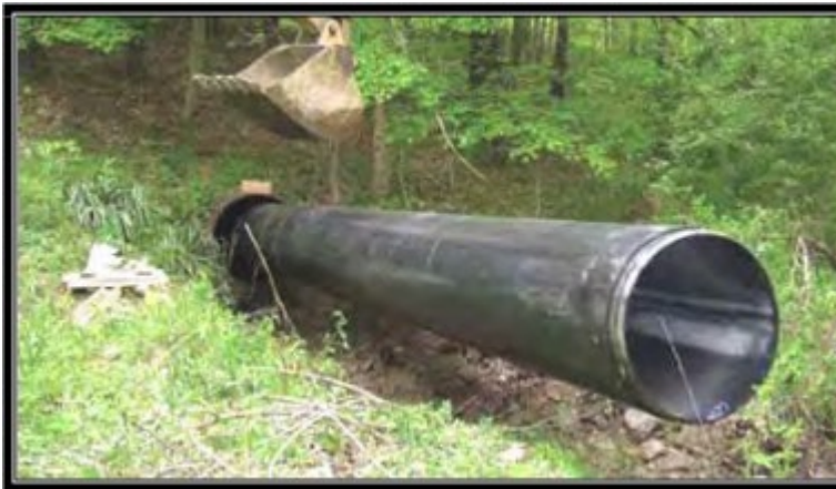
Figure 13-5 Pulling Pipe Liner
