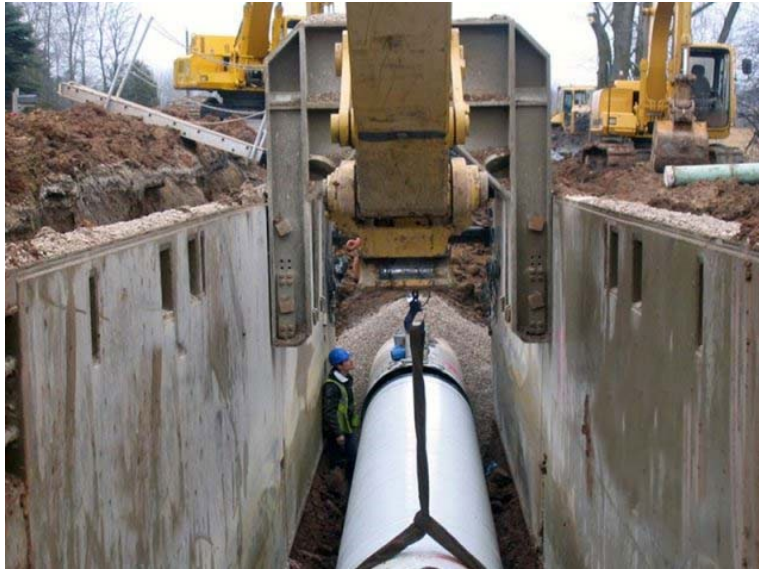
Figure 9-3 Trench Box Safety
