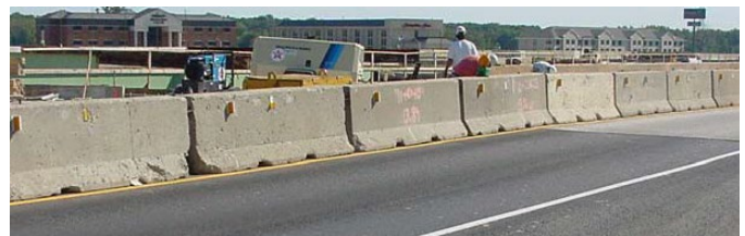
Figure 7-2 Temporary Traffic Barriers
