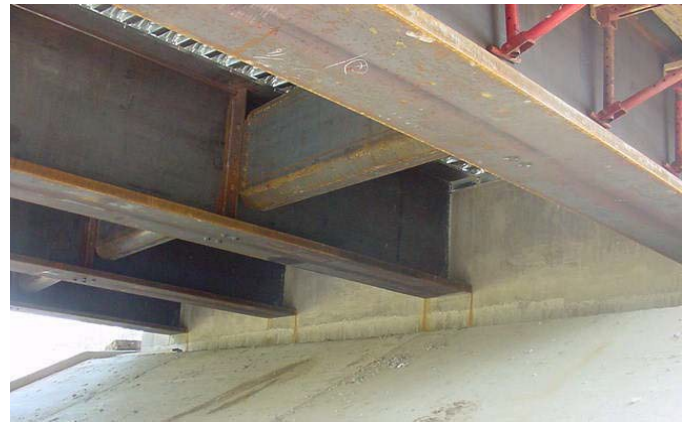
Figure 5-2 Integral End Bents
