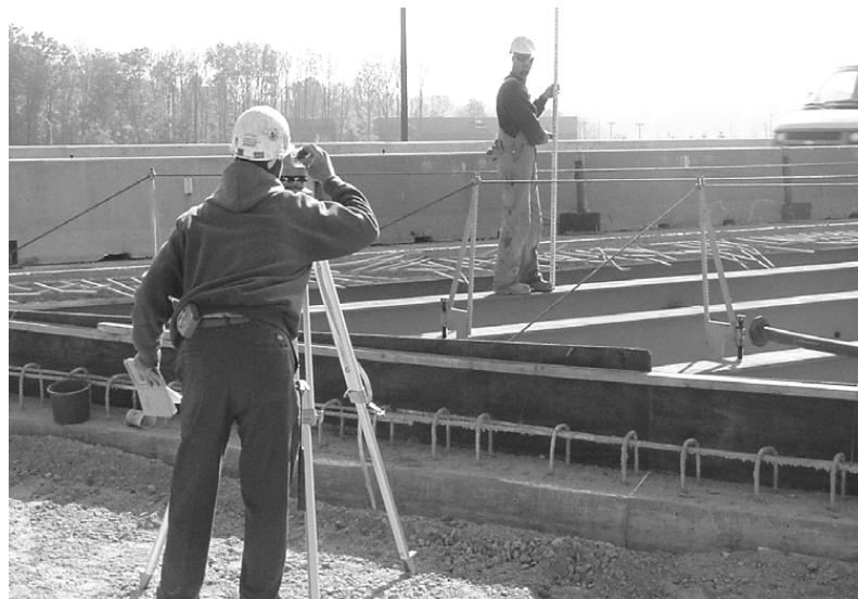
Figure 6-1 Girder Elevations
