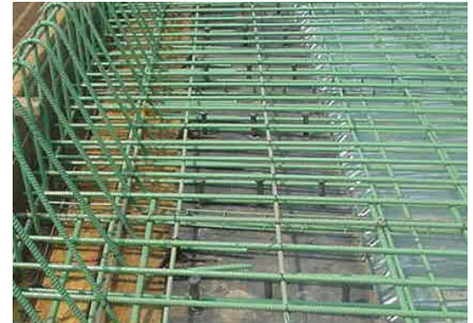
Figure 5-10 Shear Connectors
