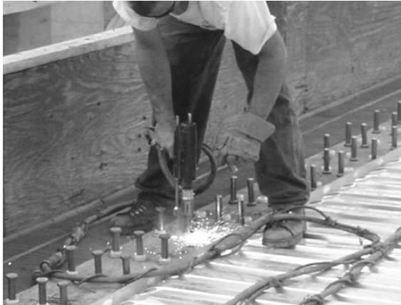
Figure 6-6 Shear Connector Studs
