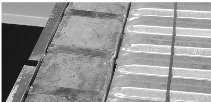
Figure 6-5 Deck Form Installation
