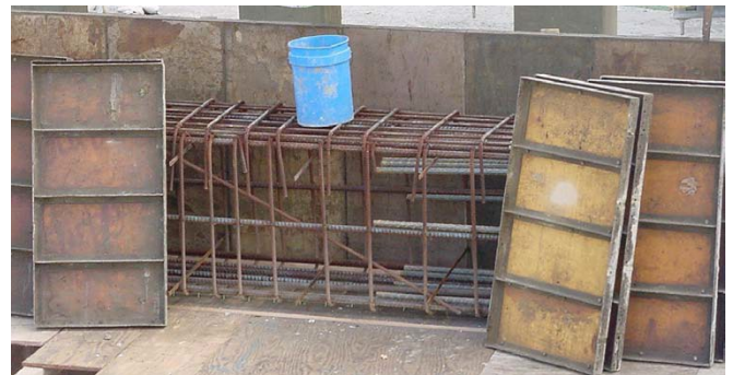
Figure 3-16 Form Clearance
