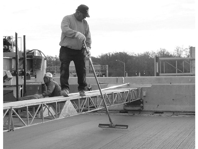
Figure 6-11 Concrete Finishing
