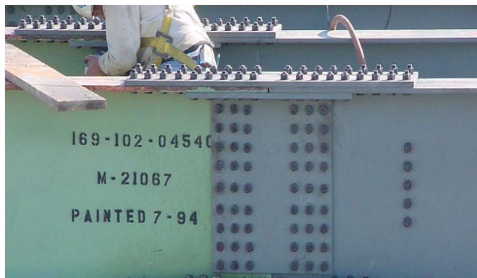
Figure 5-14 Splice Plate Bolts
