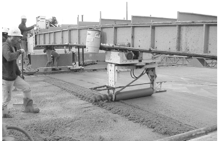
Figure 6-10 Concrete Vibrating and Striking Off
