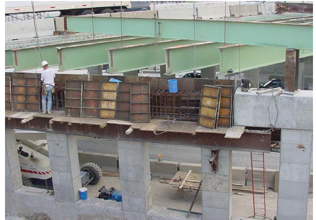
Figure 3-7 Formwork
