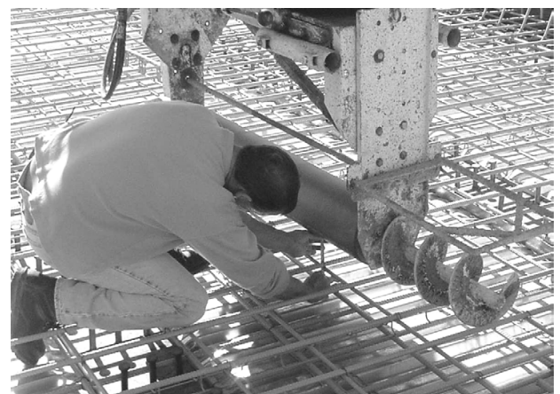
Figure 6-7 Checking Reinforcing Bar Clearance
