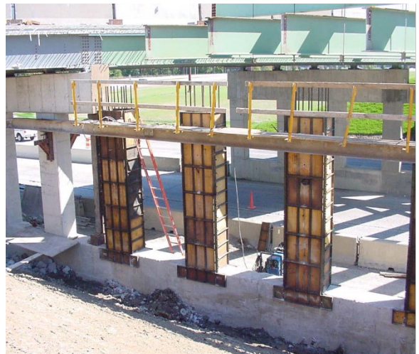
Figure 3-1 Bent Column Forms
