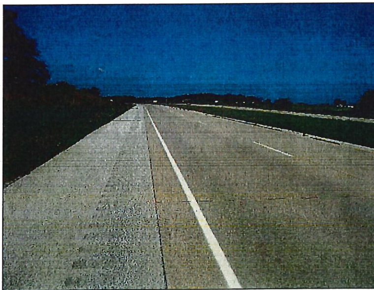
2. View looking west, from the eastern project study limits at U.S. 24.
