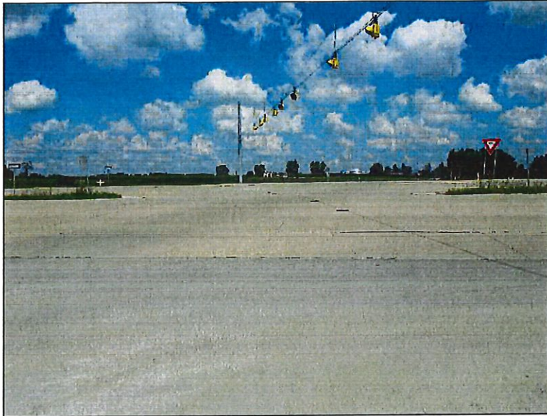
7. View looking north into the intersection of U.S. 24 and Cement Avenue.
