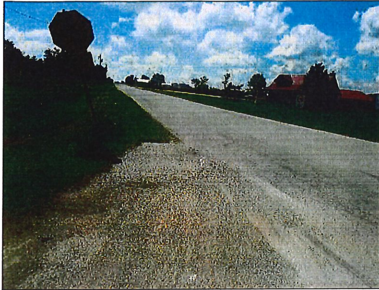
9. View from the intersection of U.S. 24 and Cement Avenue, looking south, at Cement Avenue.
