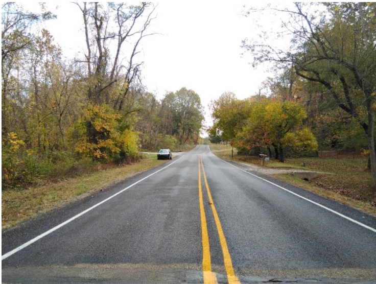
PP-14; Looking east along SR 340 and RSD 3 that is south of the road and west of the driveway.
