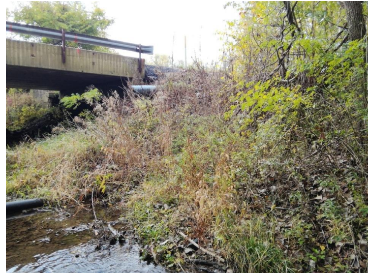
PP-4; Looking southwest along Purdy Run.
