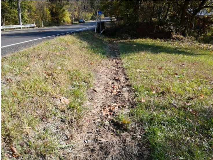
PP-12; Looking east at RSD 1 along the south side of SR 340.
