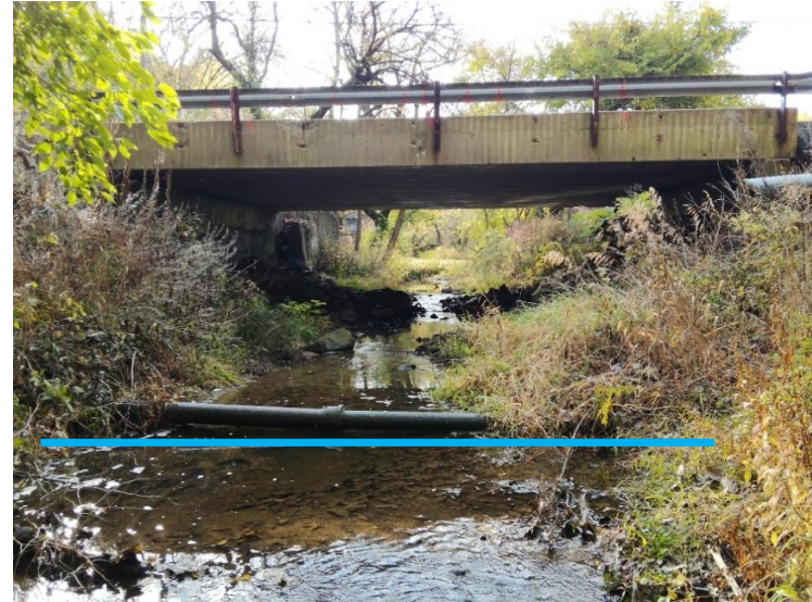
PP-2; Looking south, upstream at Purdy Run and the SR 340 bridge. OHWM at 39.507893, -87.201400
