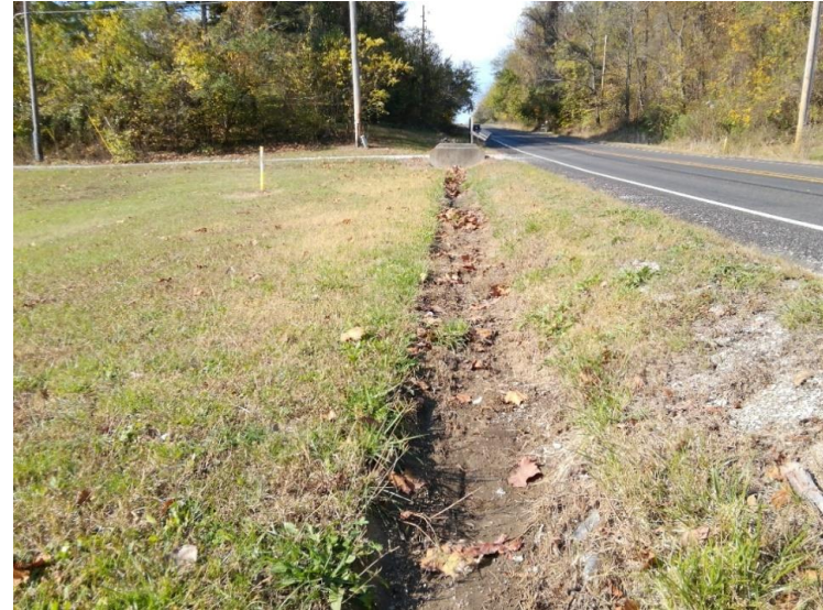
PP-13; Looking west at RSD 1 along the south side of SR 340.
