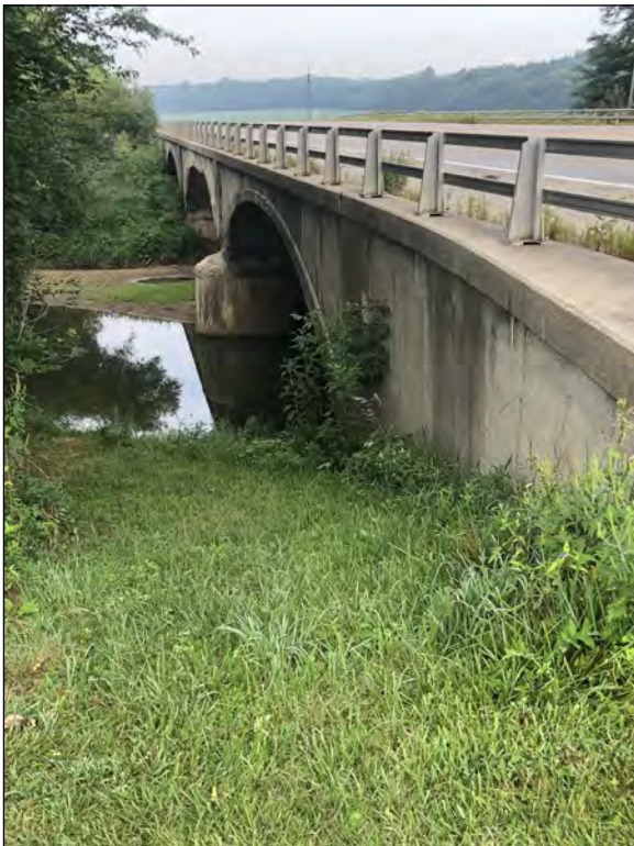
Picture 11—Southeast quadrant, Nolands Fork and structure; northwest view; 16 AUG 2019.
