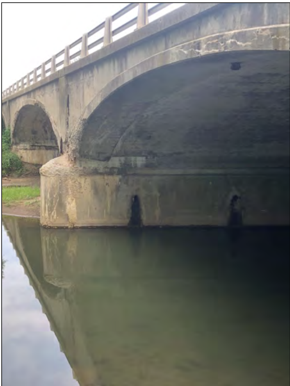
Picture 31—Nolands Fork and structure, northeast view; 16 AUG, 2019.
