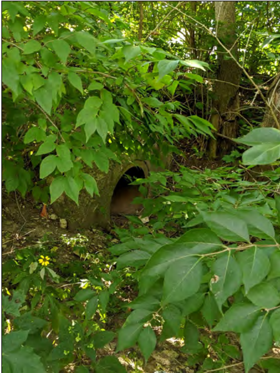
Picture 33—Pipe outlet to RSD1; east view; 16 AUG 2019.
