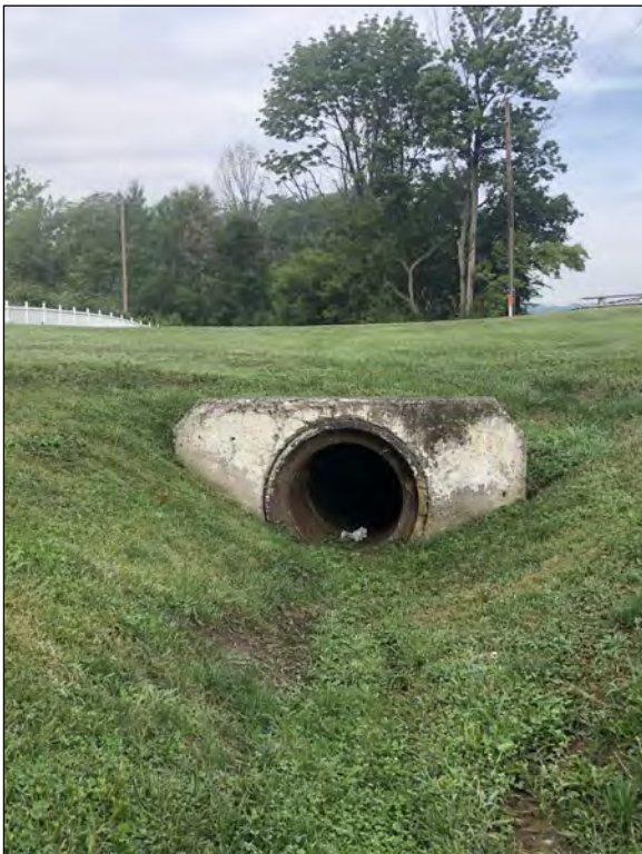
Picture 7—RSD 1 pipe; west view; 16 AUG 2019.
