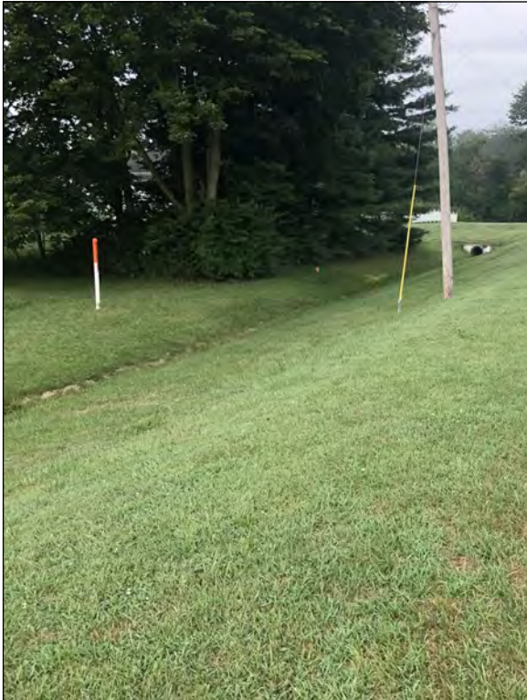
Picture 5—RSD 1 ; southwest view; 16 AUG 2019.
