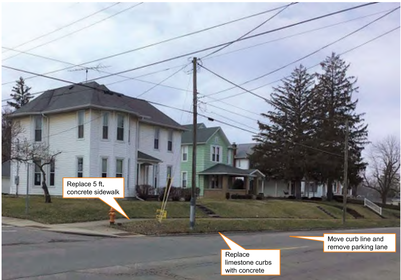
25 Looking southwest across the SR 46 and Wilder Street intersection at "Contributing" houses within the Greensburg Eastside Residential Historic District.
