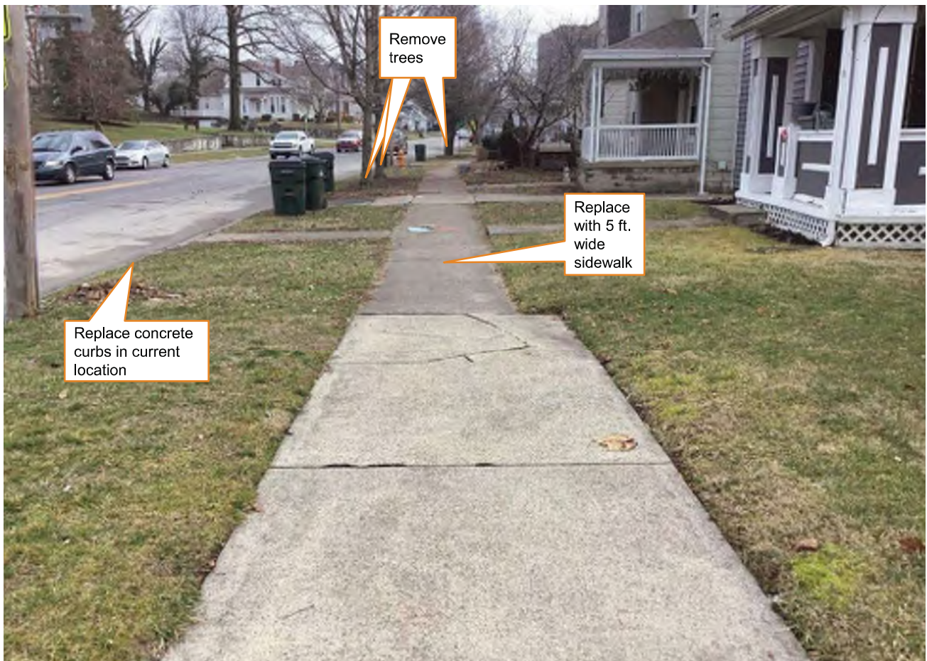
8 Looking east along the south side of SR 46 in the Greensburg Eastside Residential Historic District.
