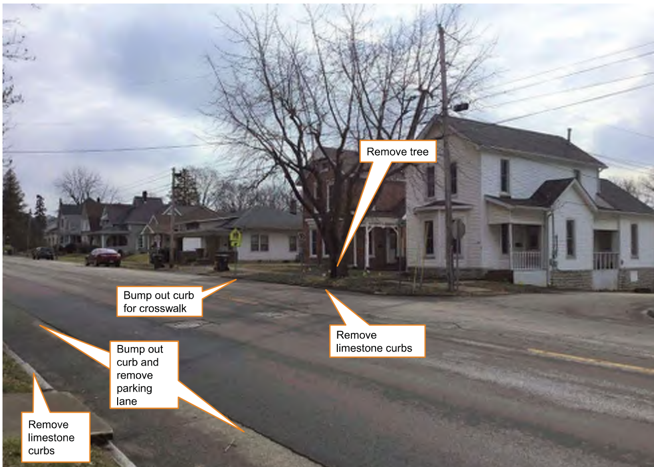
10 Looking southeast across SR 46 towards Poplar Street in the Greensburg Eastside Residential Historic District.
