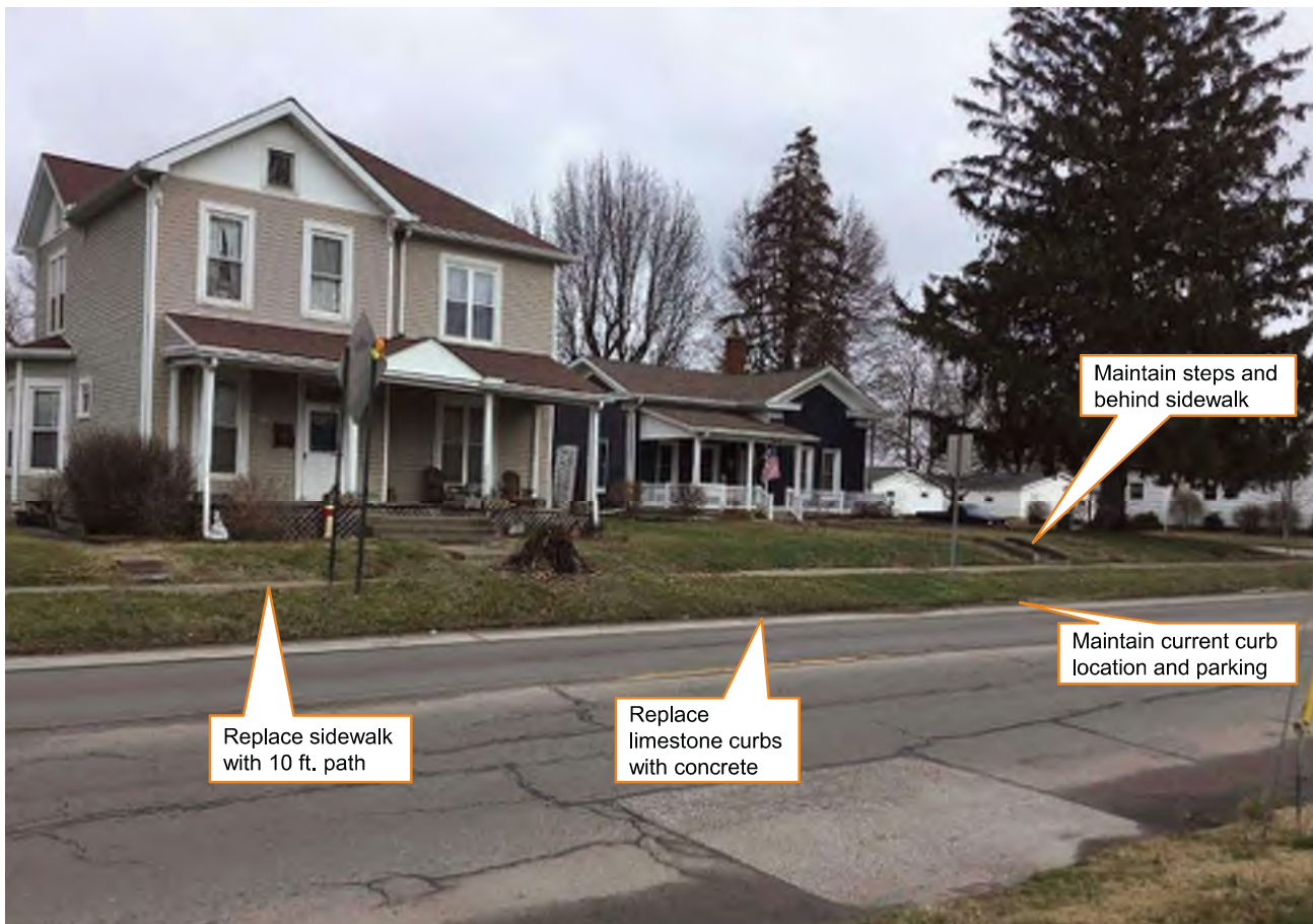
29 Looking northeast across SR 46 towards Warren Street at “Contributing” houses within the Greensburg Eastside Residential Historic District.
