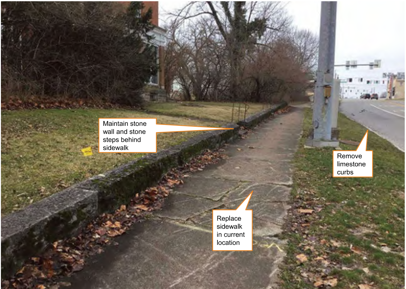
2 Looking east in front of the NRHP-eligible Charles Zoller House.
