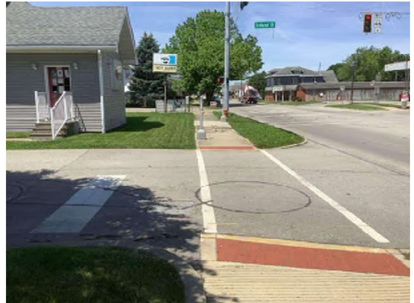
24. Facing west from the SR 46 and N. Ireland St. intersection at the surrounding landscape.
