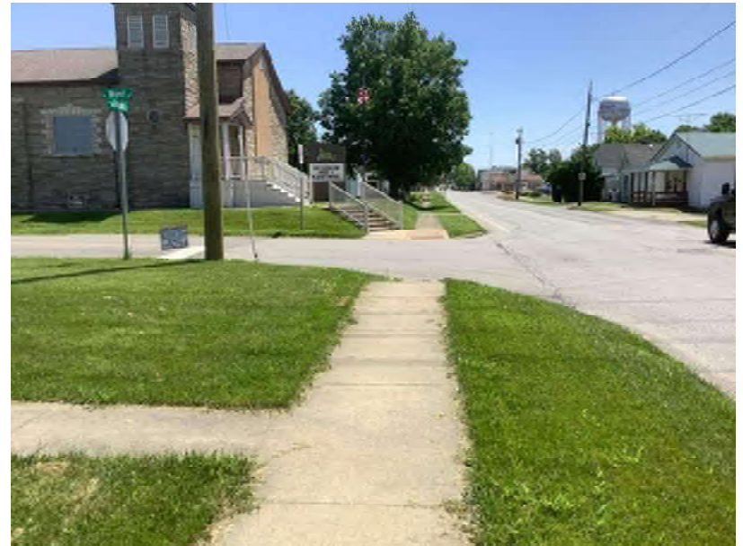
20. Facing east looking at the intersection of SR 46 and West St. along the westbound lane of SR 46.
