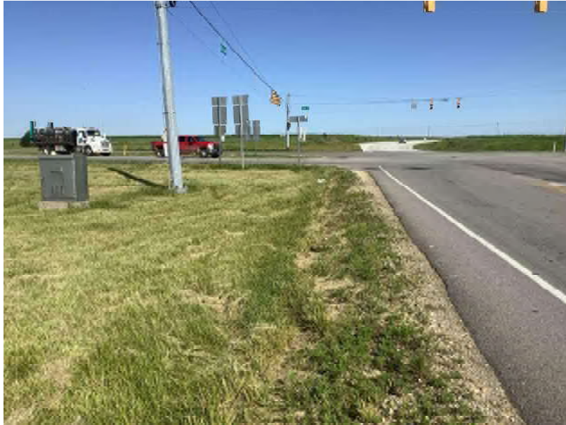
1. Facing northwest towards the northwest end of the project area (Des No. 1800255) looking at SR 3 and SR 46 intersection.
