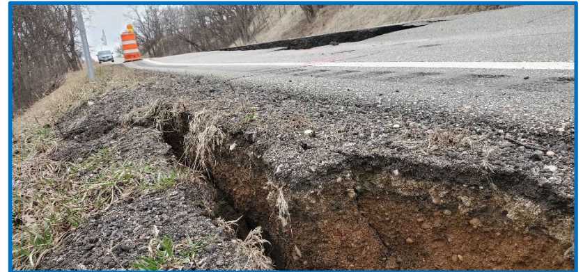
Model assist in proactive identification of slope failures like deep-seated slide in TH-67
