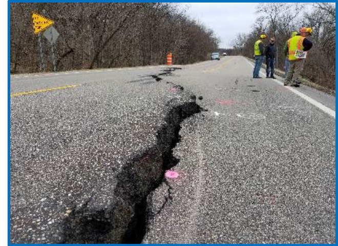
Model assist in proactive identification of slope failures like deep-seated slide in TH-67
