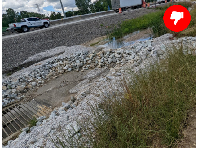
Trap placed within ditch and allowing sediment to reach the inlet. The flow was not controlled, which may indicate additional measures are needed, and the sediment trap needs maintenance.
