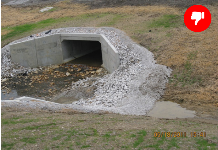
Sediment trap with too much filter stone.
