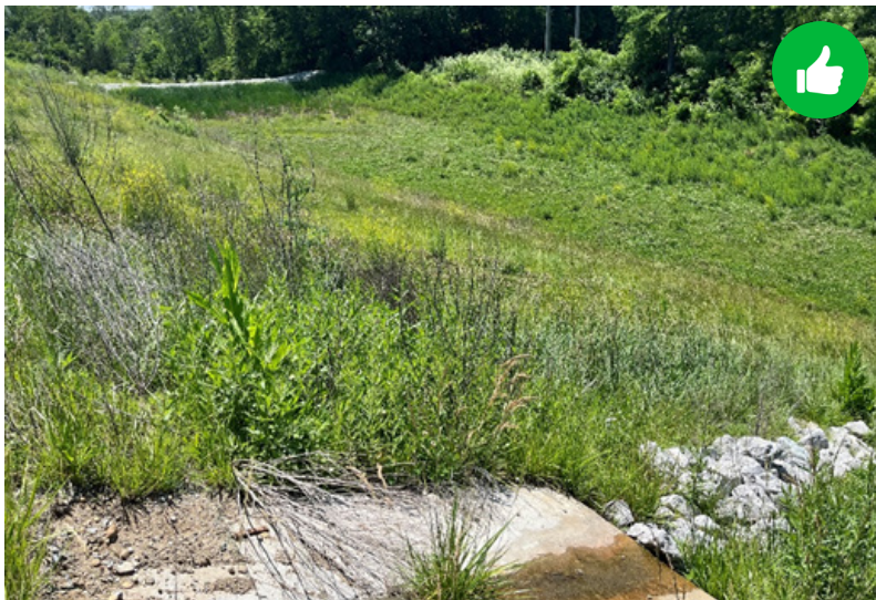
Sediment trap placed in an appropriate location close to stream with filter stone.
