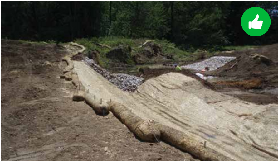
Stable diversion interceptor around a box culvert installation (not pictured).
