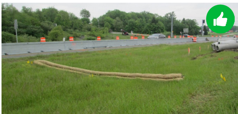
Filter sock installed in a pyramid and high on sides of bank, to ensure flow does not go around measure.
