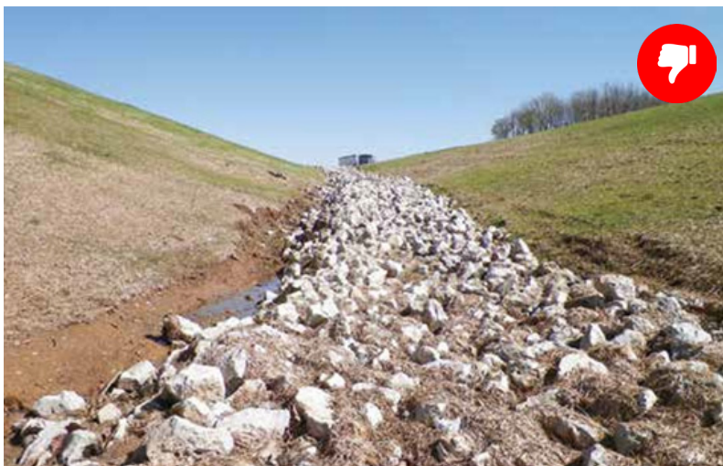
Riprap is not extended far enough up the slope and not shaped correctly, causing scour.
