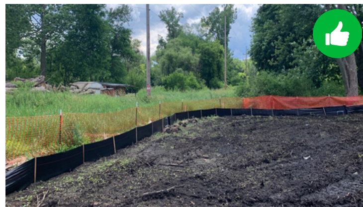
Silt fence and protective resource fence protecting a wetland (environmentally sensitive area).
