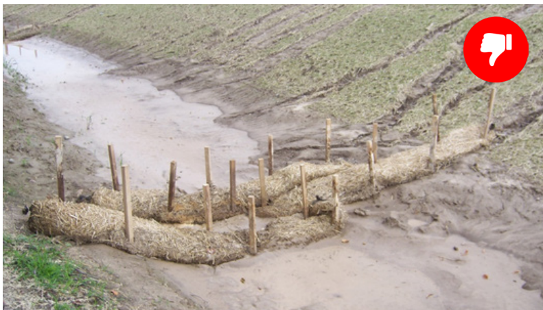
The water volume and velocity in this area are too much for traversable check dams. There should be more focus on erosion control with seed, mulch and erosion control blanket.
