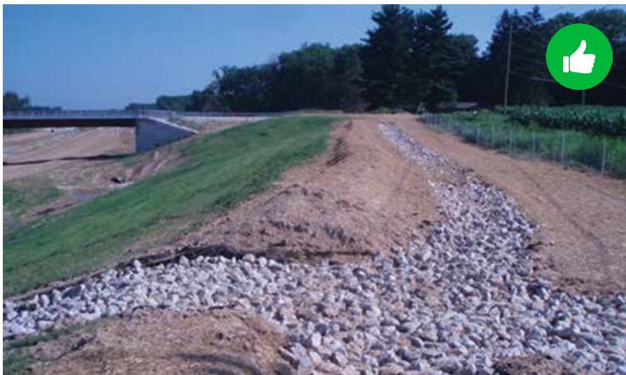
Example of permanent diversion interceptor installation.
