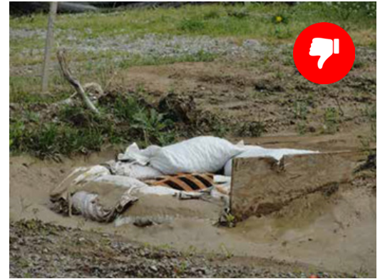
Inappropriate and ineffective inlet protection.
