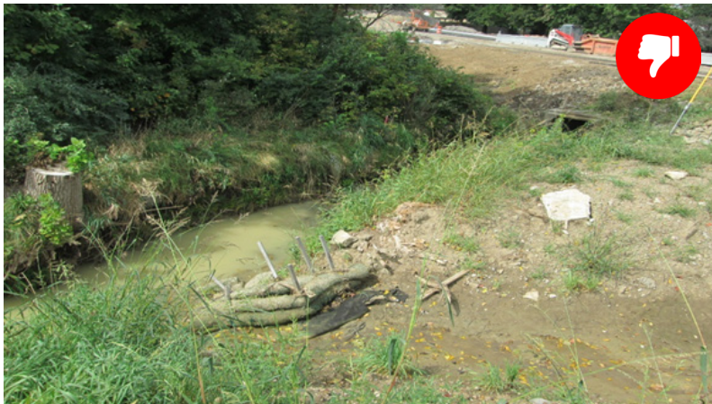
Filter sock check dams undermined due to high velocities.
