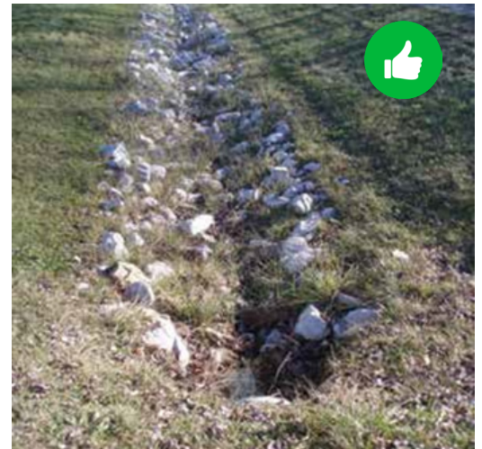
Permanent riprap ditch with correct shape and placement.
