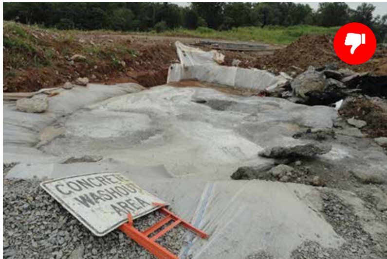
Concrete washout is part of a good housekeeping plan. Concrete washout not properly maintained.
