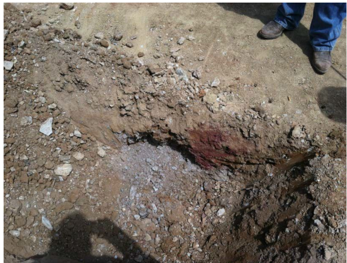
(b) Poorly mixed lime-soil modified soil
