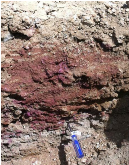
(a) Well mixed lime-soil modified soil
