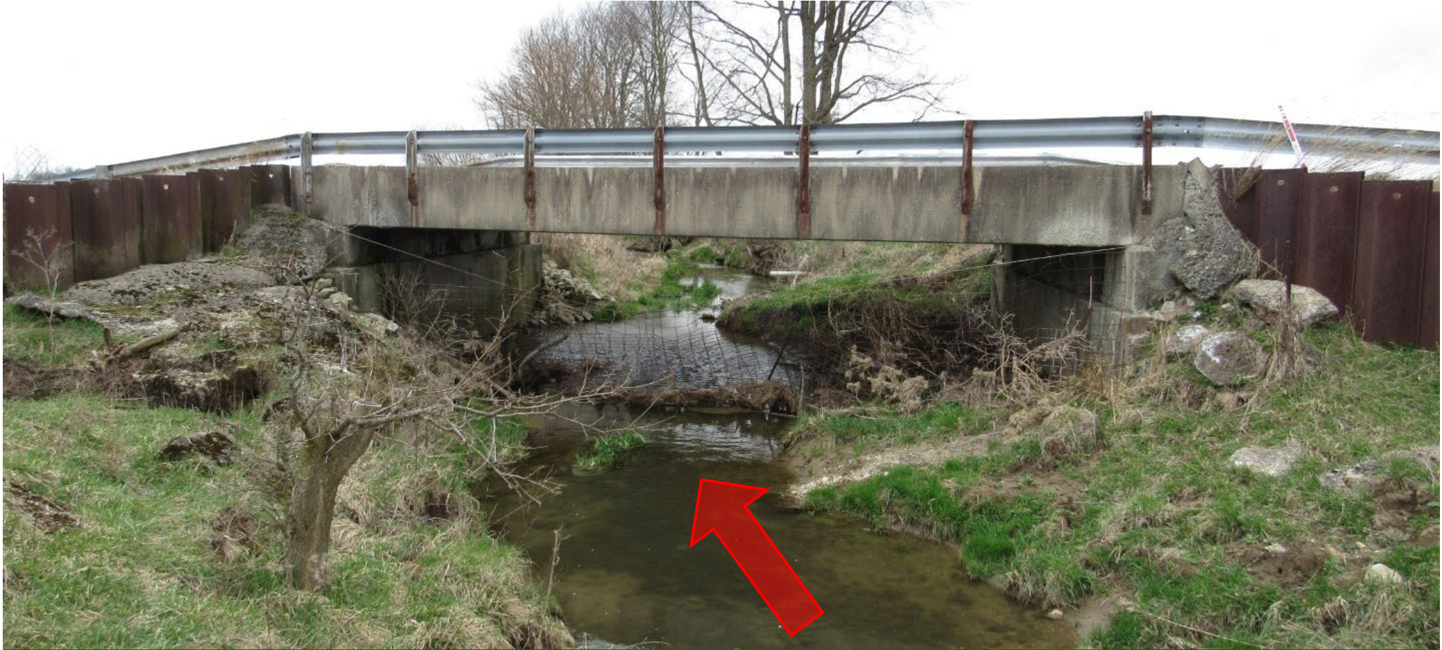
East (upstream) side of bridge - cattle fence with minor debris
