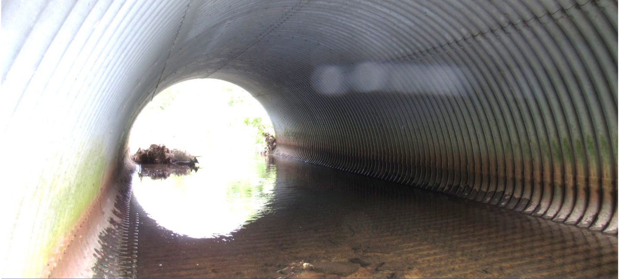
Typical view of pipe interior
