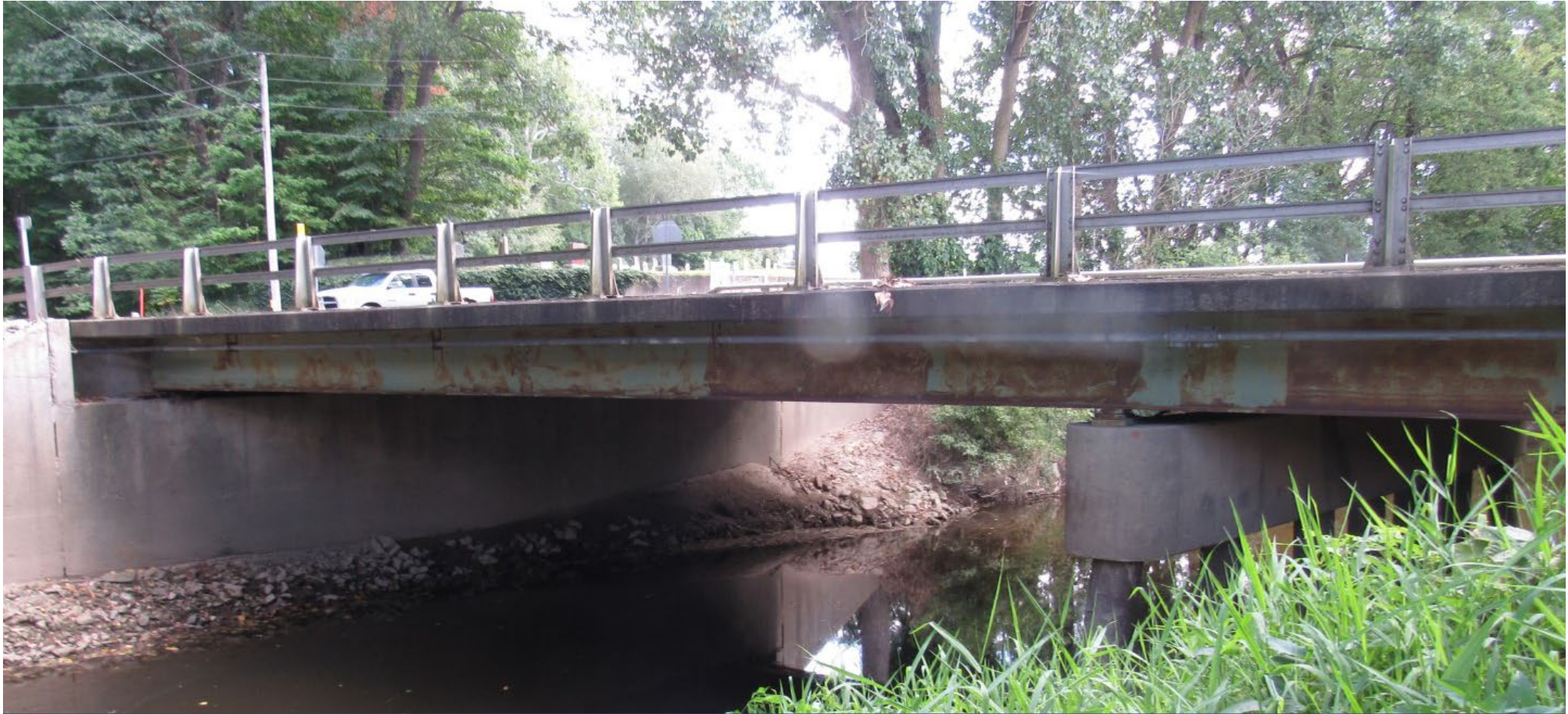
Two-span steel beam bridge with concrete deck built in 1972
