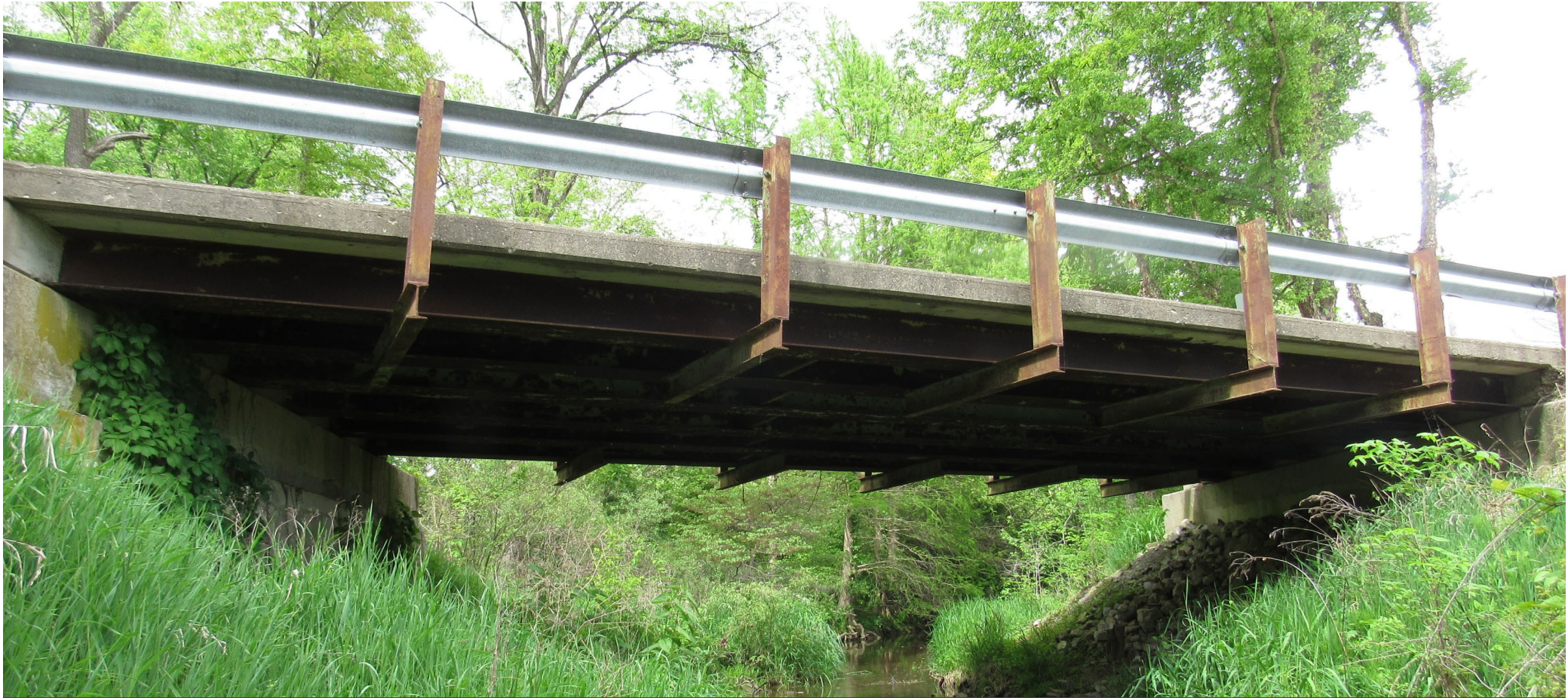
Single-span steel beam bridge
