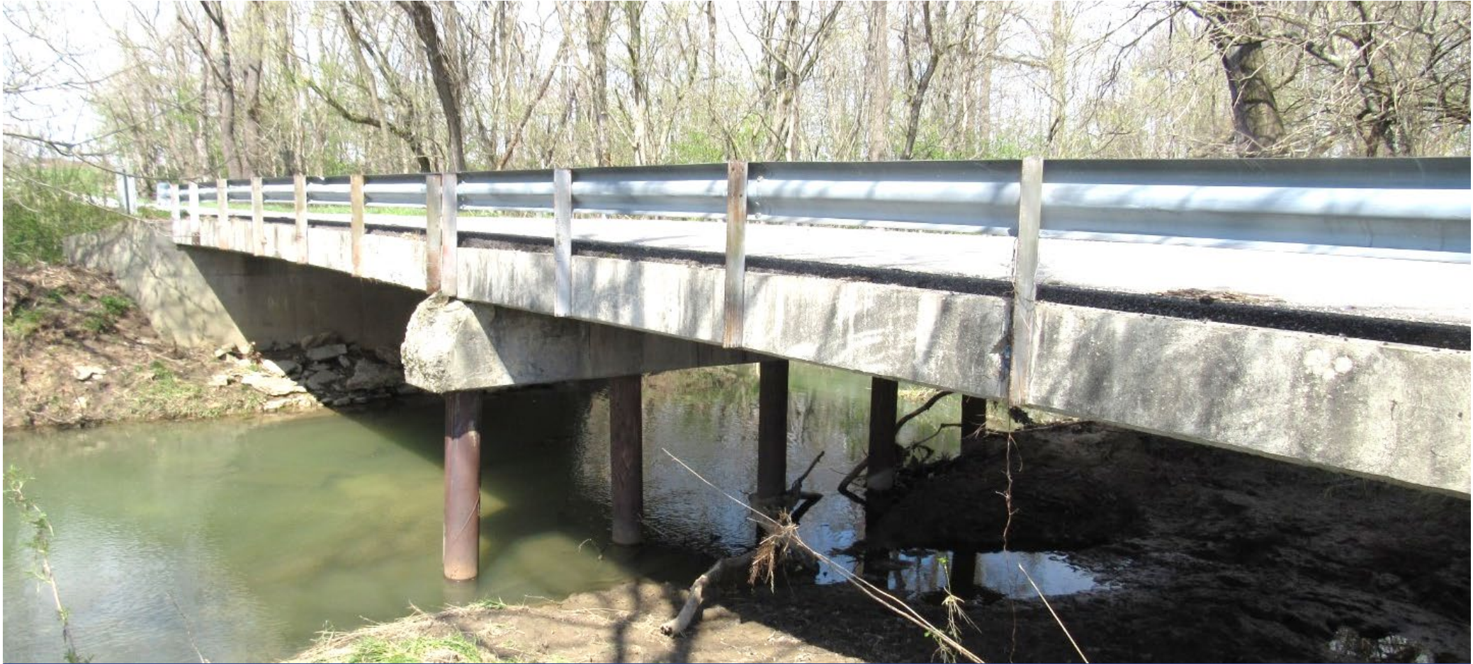
Two-span bridge with concrete wall abutments and center open pile bent
