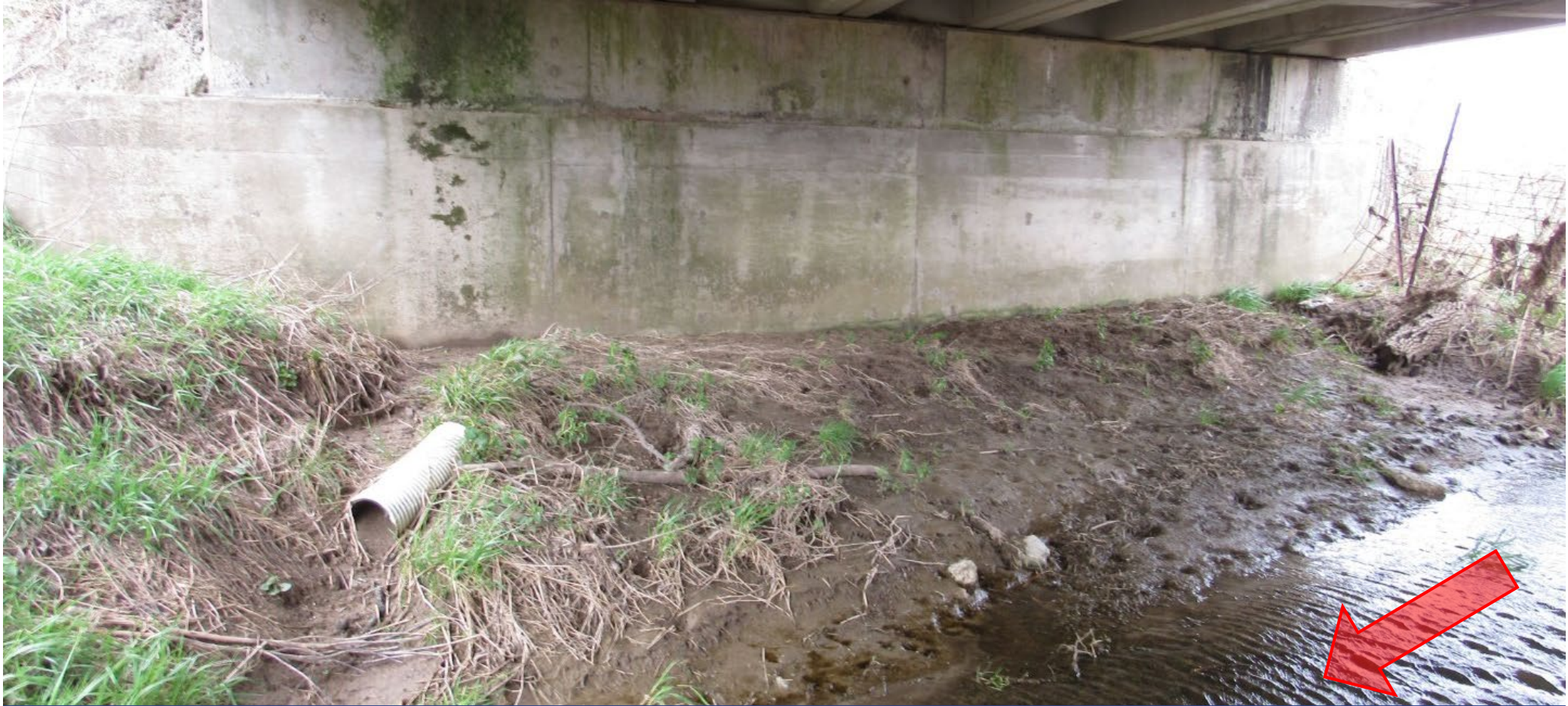
North abutment - channel shifted away
