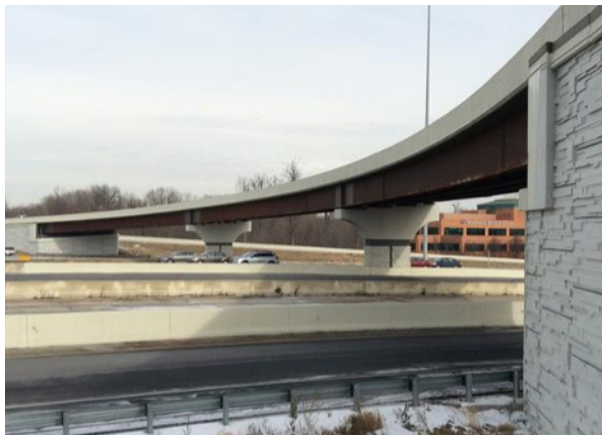
Ramp I-465 to US31N over I-465 EB/WB Ramps
