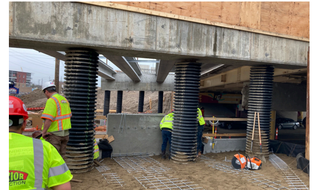
Low headroom was a challenge during the North Split Project.
