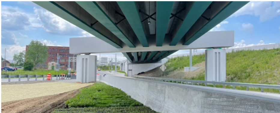
North Split Straddle Bent
