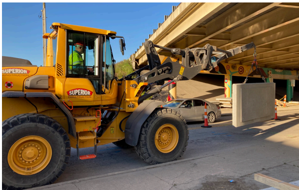
North Split MSE wall construction.
