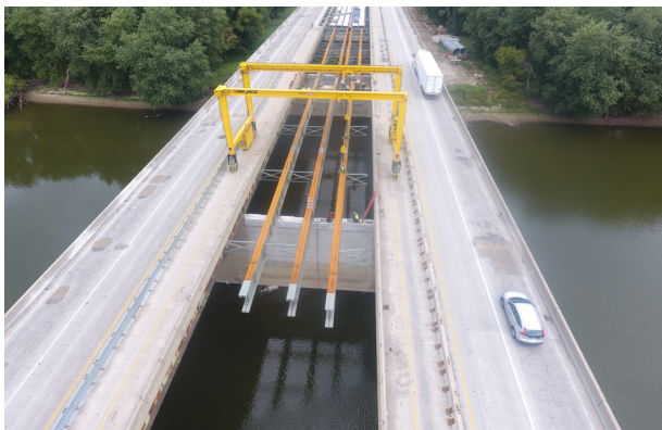
Gantry Innovation at I-65 over the Wabash River Experience of the Firms
