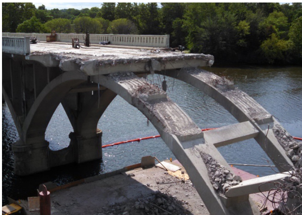
Demolition of US 24 Bridge Replacement over the Tippencanoe River
