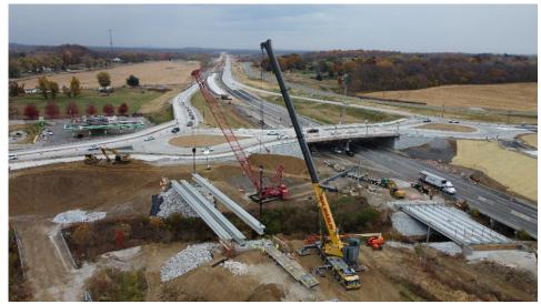
Rieth-Riley implemented the approved plan. This plan included installing temporary pavement for the access points, temporary barrier wall and temporary construction attenuators in a manner that would still provide positive protection for the traveling public on the roadway but would also grant space for construction traffic to make a protected left turn into, or out of, the construction site.
