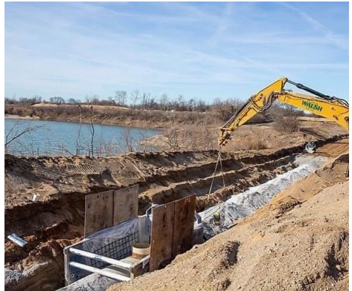
FIGURE 4.3 // INNOVATIVE IDEA IMPLEMENTED ON I-69 SECTION 6 CONTRACT 5.
