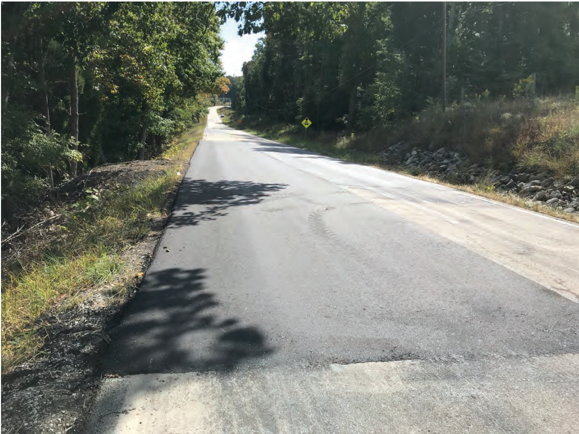
2. Looking southeast at new temporary overlay in project area
