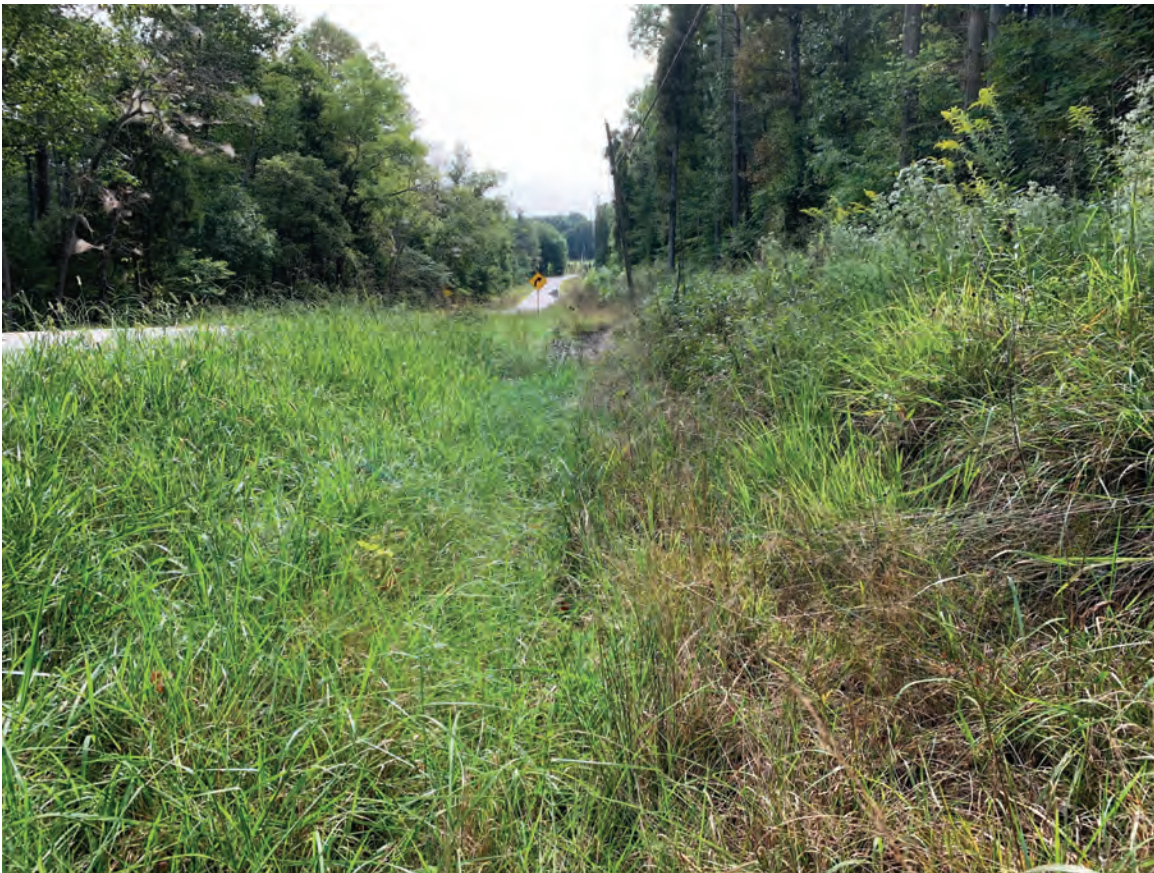
10. View of roadside ditch, looking east
