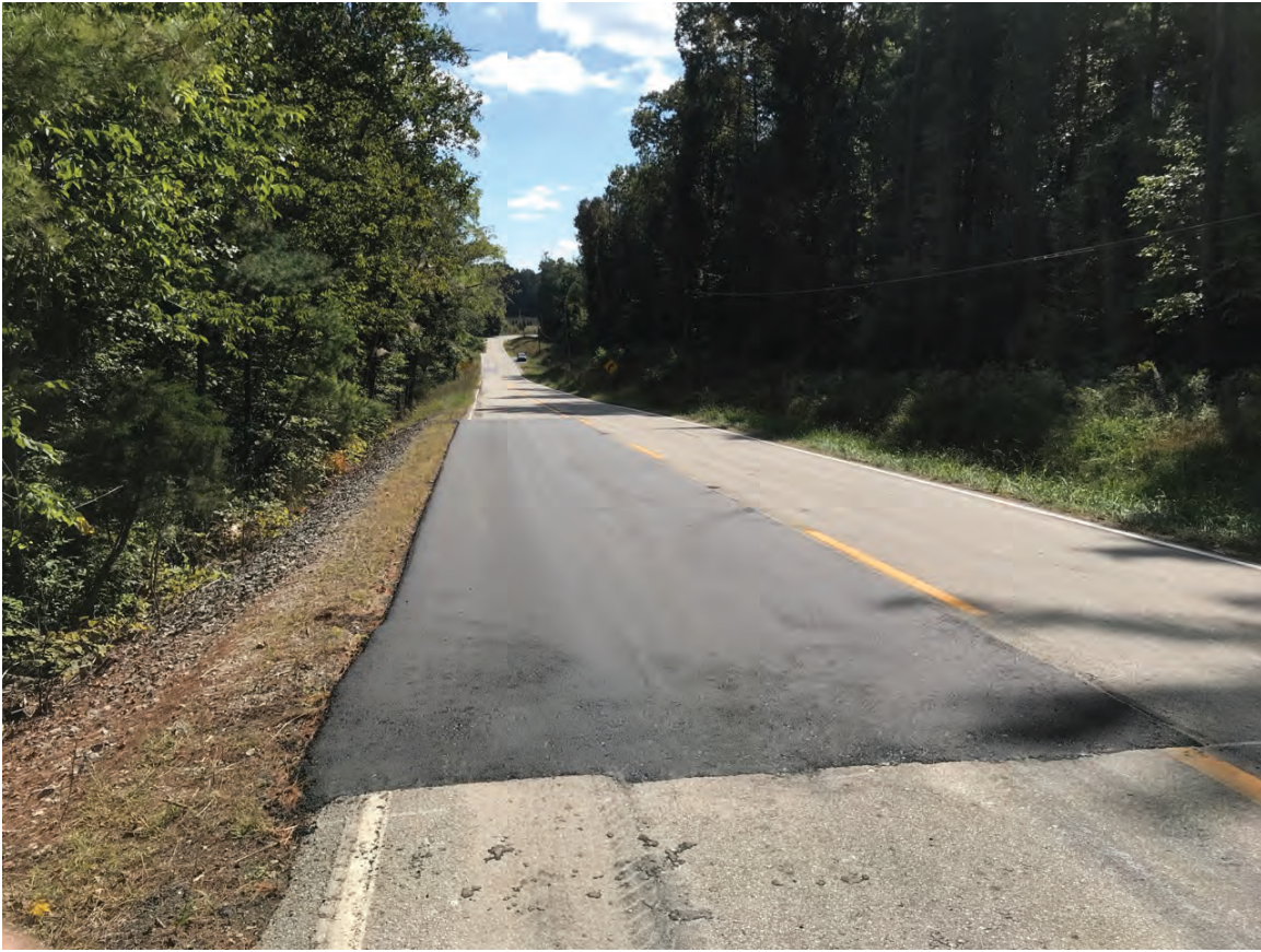
3. Looking southeast at recent temporary overlay in project area
