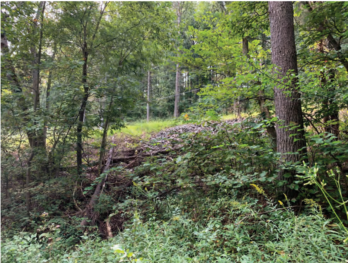
8. Looking southeast at SR 62 embankment
