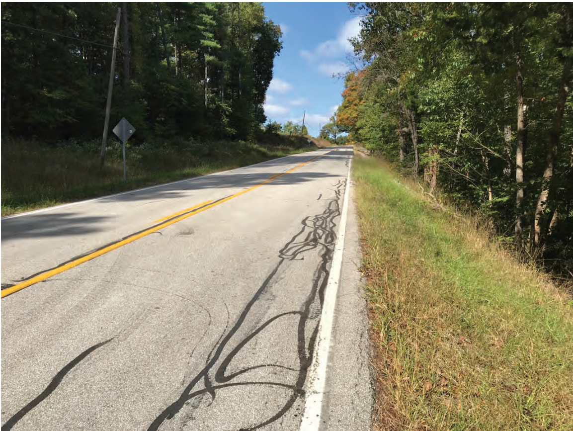
4. Looking northwest across project
