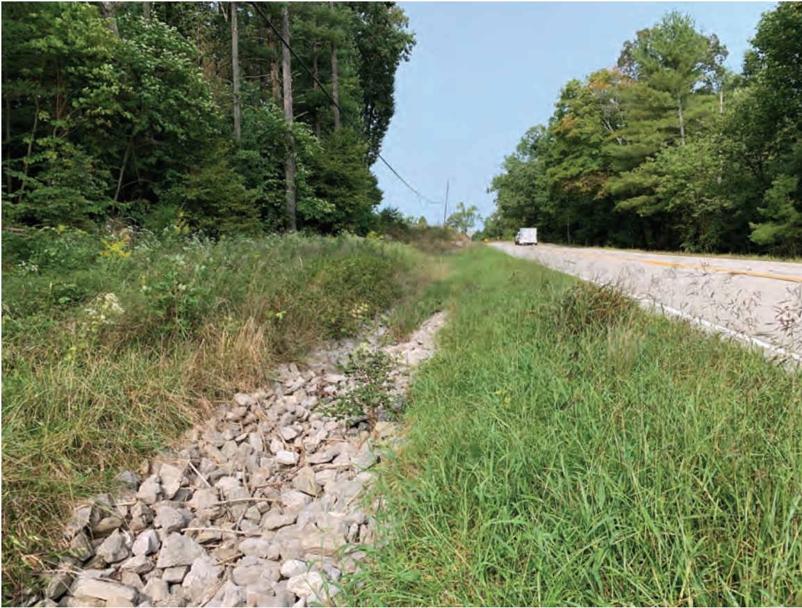
9. View of roadside ditch, looking west
