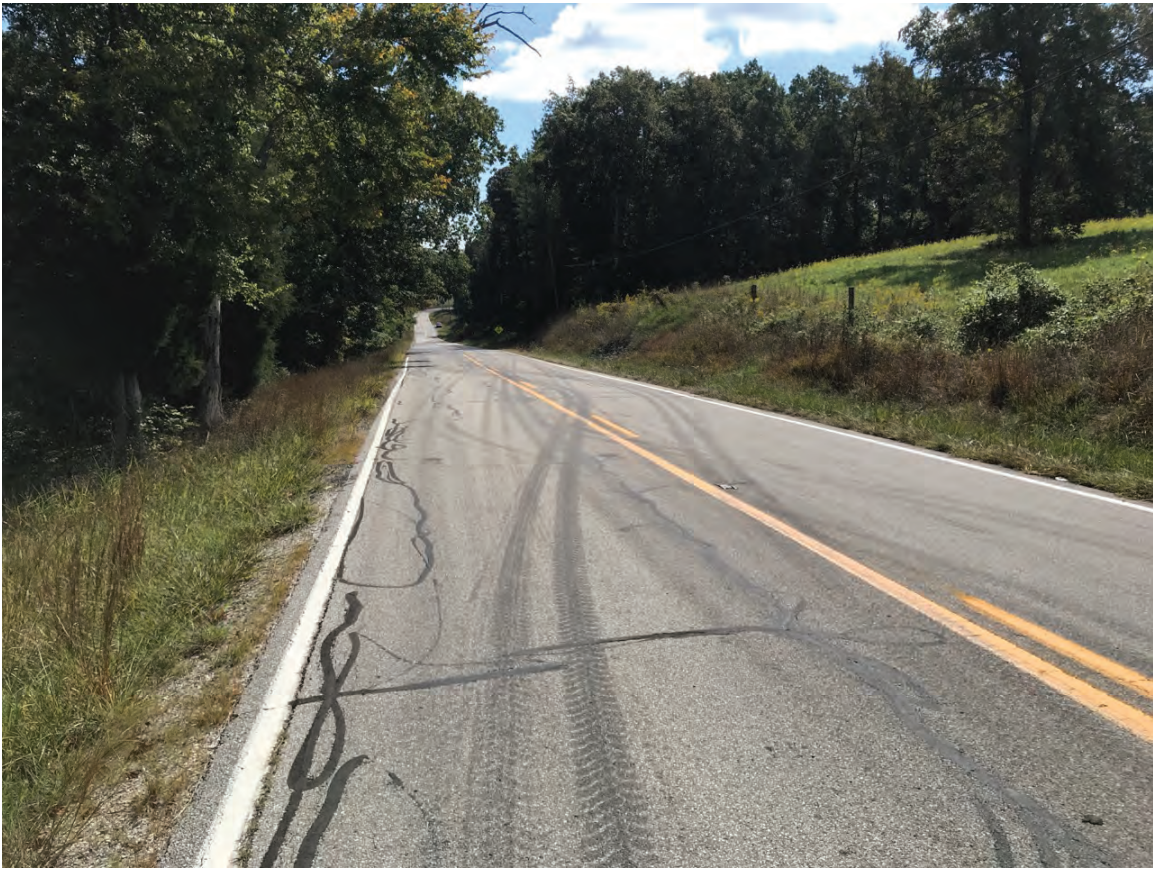
1. Looking southeast into project area
