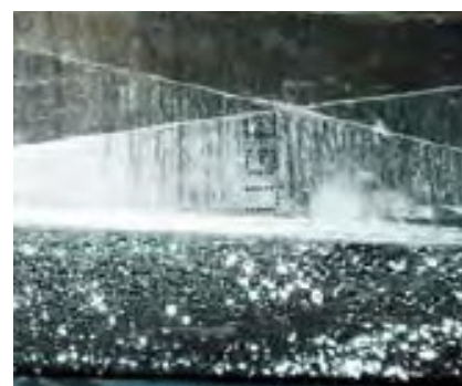
Duct condensation heater
