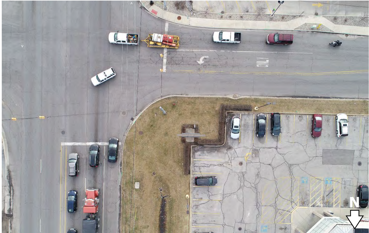
Figure 46 An aerial image of the northwest quadrant of the intersection of US 41 and W 133 rd Ave. The image is oriented south.
