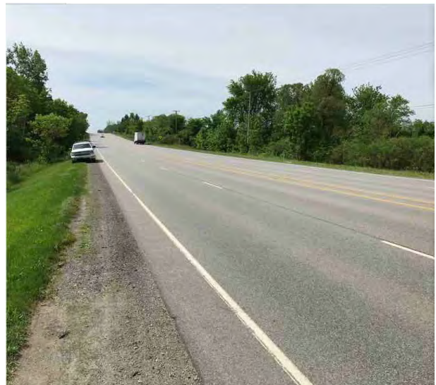
Figure 29 The eastern shoulder of US 41, facing south.
