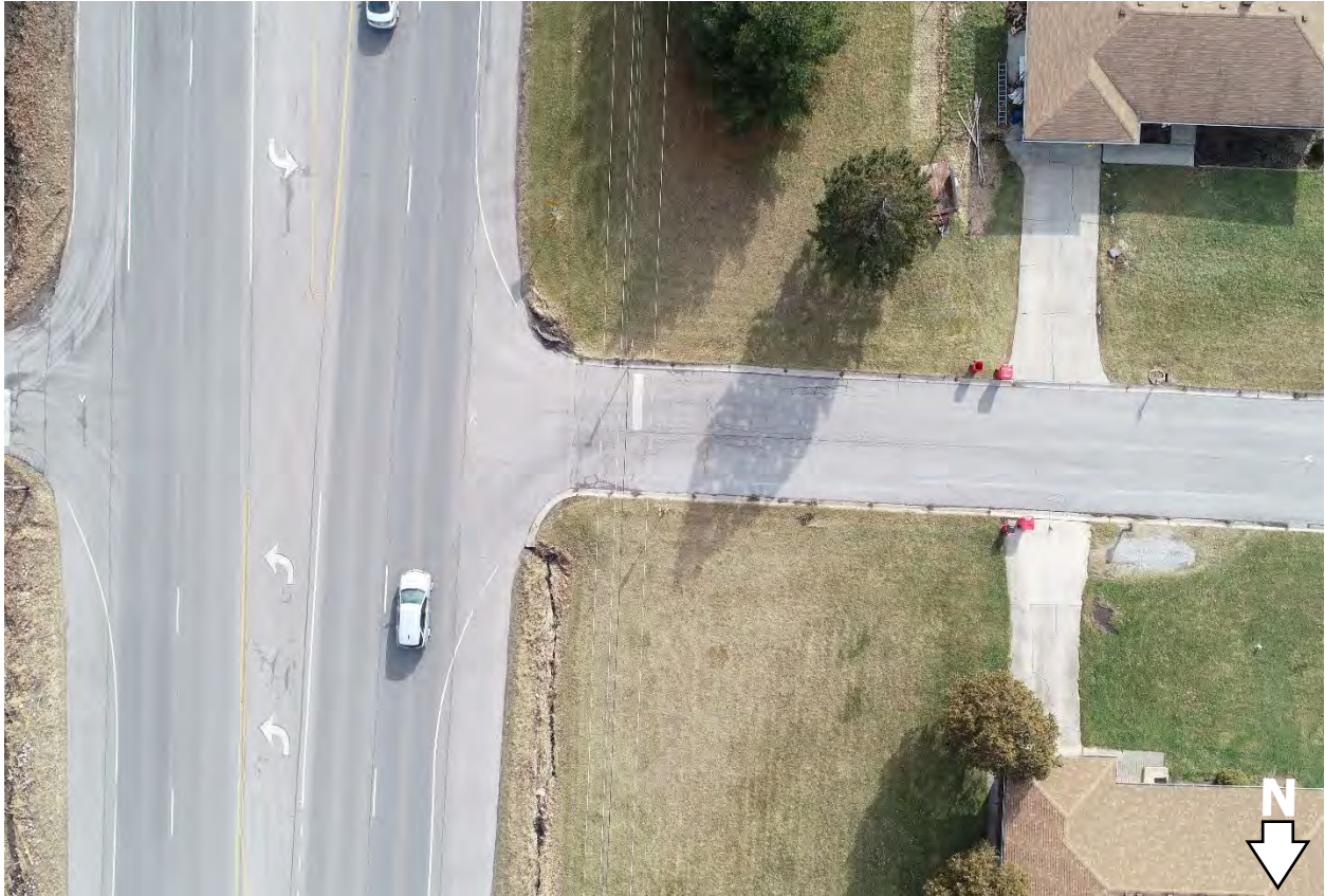
Figure 52 An aerial image of the western approach of the intersection of US 41 and W 135 th PI. The image is oriented south.
