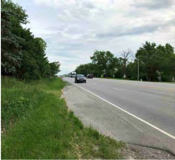
Figure 11 The western shoulder of US 41 facing north.
