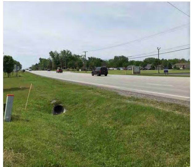
Figure 37 The eastern shoulder of US 41 facing southwest.
