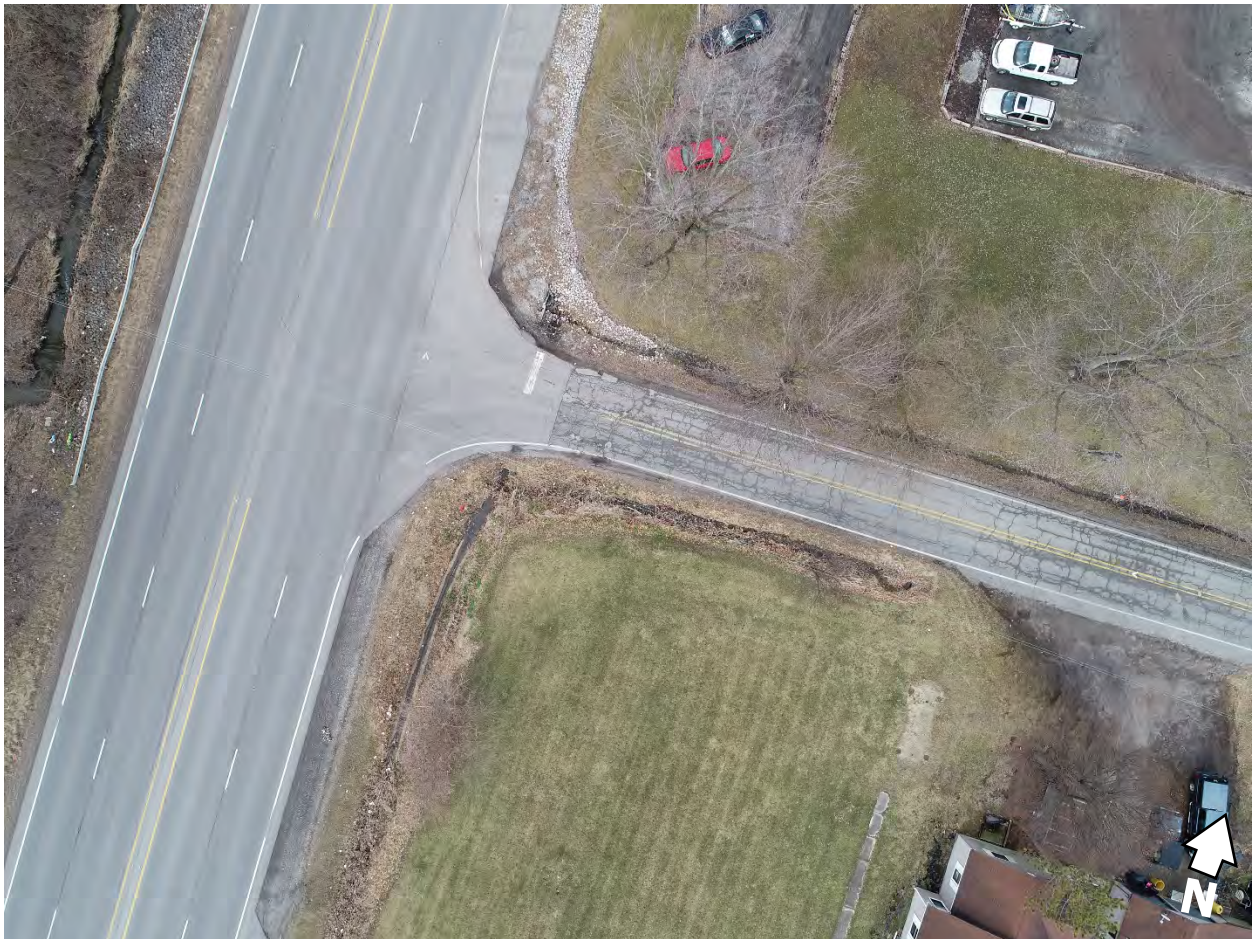
Figure 18 An aerial image of the intersection of US 41 and W 117 th St. The image is oriented north by northwest.
