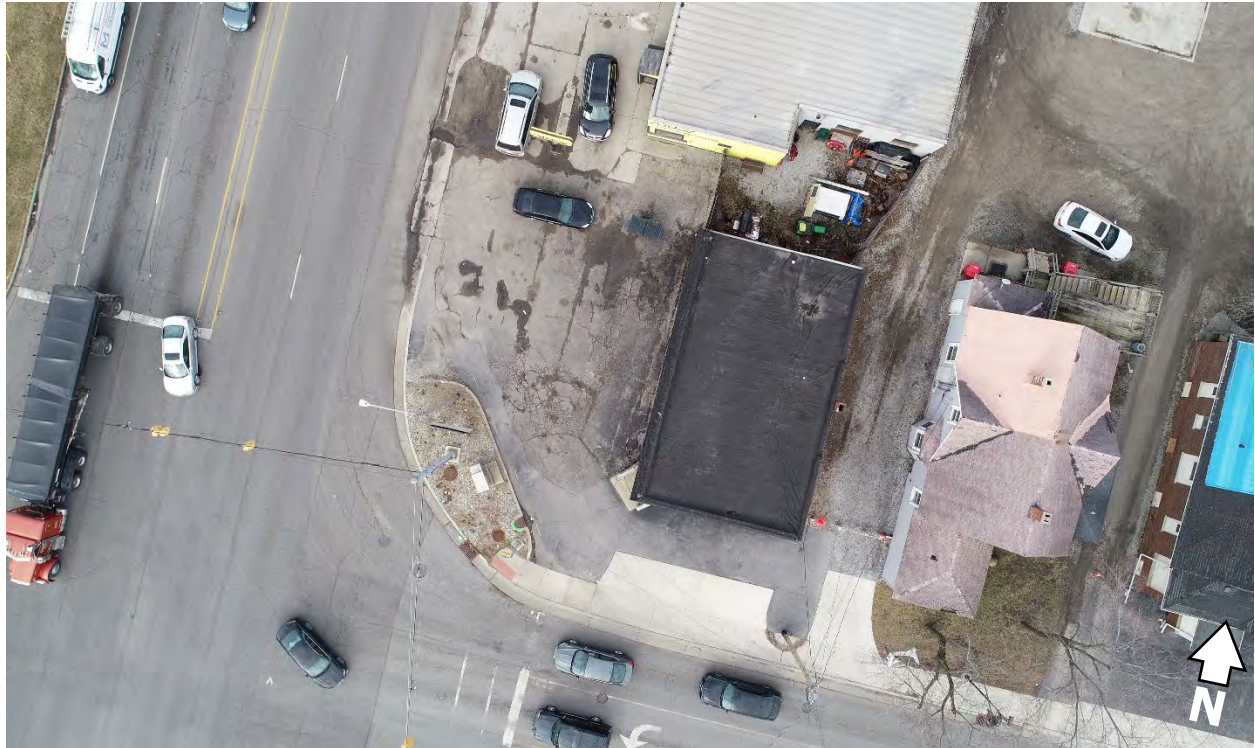
Figure 48 An aerial image of the northeast quadrant of the intersection of US 41 and W 133 rd Ave. The image is oriented north by northwest.
