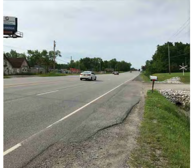
Figure 9 The western shoulder of US 41 facing south.
