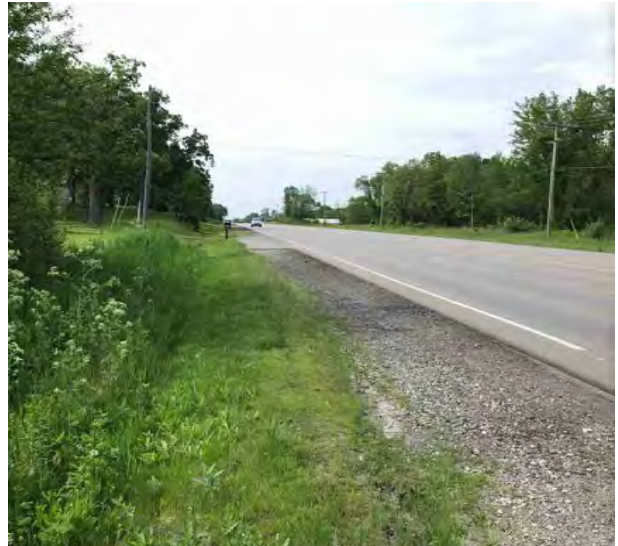
Figure 22 The eastern shoulder of US 41 facing south.
