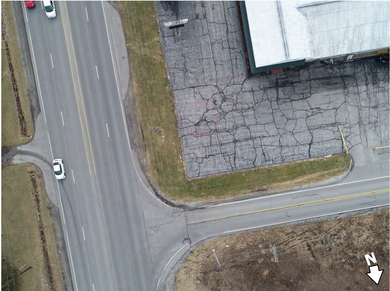
Figure 23 An aerial image of the intersection of US 41 and W 119 th Ave. The image is oriented south by southwest.
