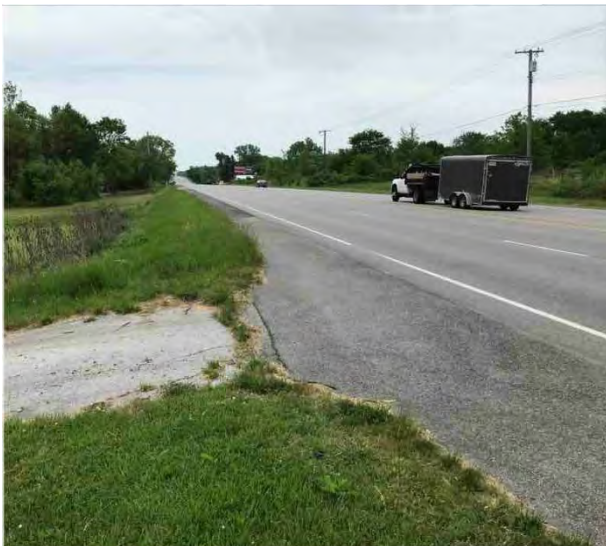
Figure 13 The eastern shoulder of US 41 facing south.
