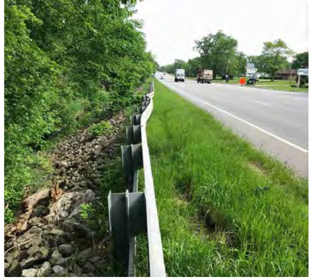
Figure 20 The western shoulder of US 41 facing north.
