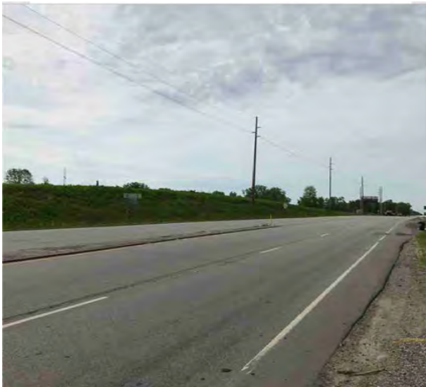
Figure 6 The western shoulder of US 41 facing southeast.
