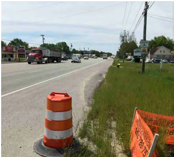
Figure 31 The western shoulder of US 41 facing south.
