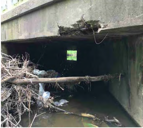
Figure 16 The eastern outlet of structure no. CV 041-045-257.55.
