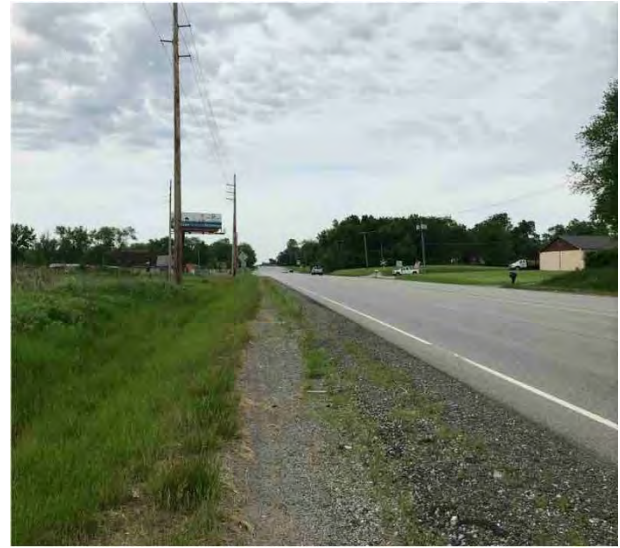
Figure 7 The eastern shoulder of US 41 facing south.
