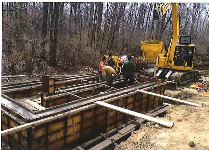
Farmland, IN: Pouring concrete walls for Disinfection Channel
