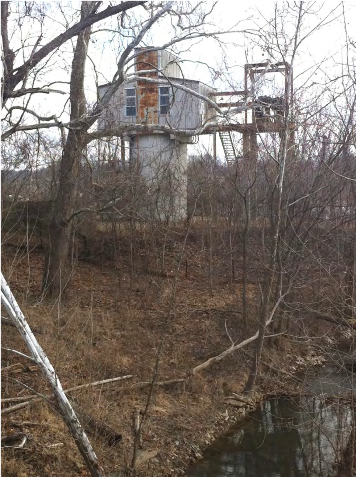
Figure 67: Collector Well CW-2
