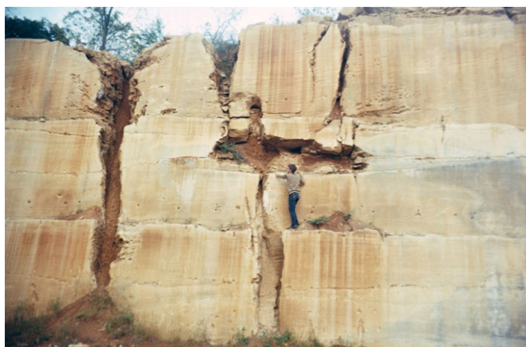
Figure 56. Photo of epikarst, which is near-surface dissolution of limestone that creates cavities and enlarged natural pipes that can convey water and contaminants into the subsurface. These voids are often filled with soil and surrounded by vegetation, so the additional vulnerability to water quality and infrastructure is not evident. Photo by Noel Krothe, date unknown.
