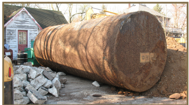
8,000 gallon tank removed
