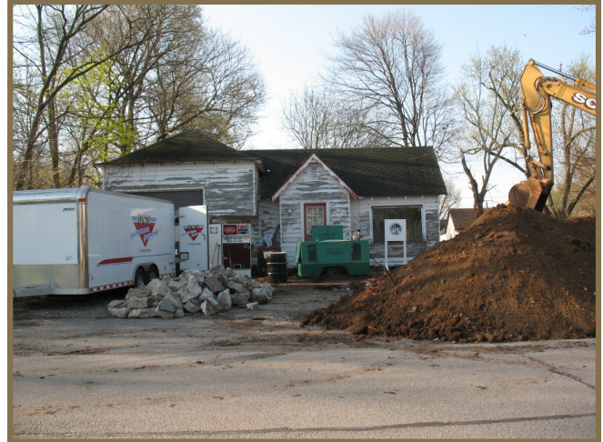
Work being performed at Site
