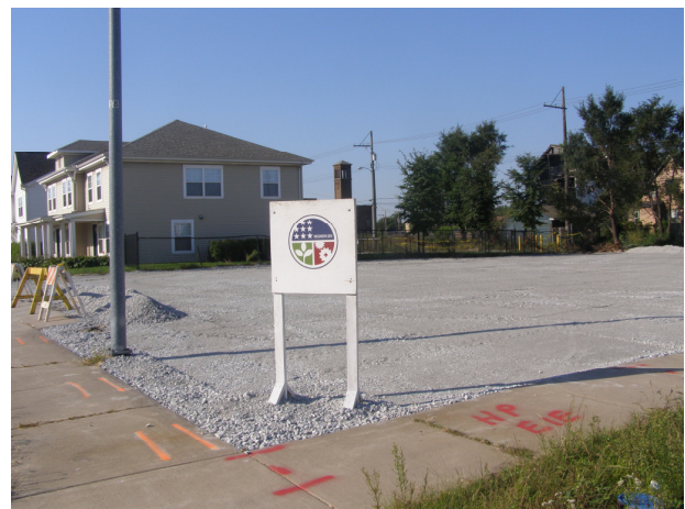
Site after demolition and UST removal
