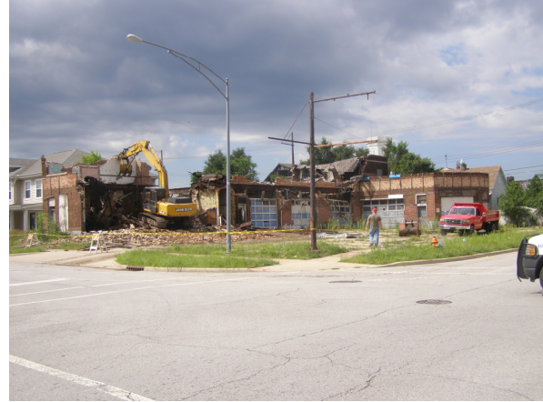
Building demolition funded with state Supplemental Environmental Project funds
