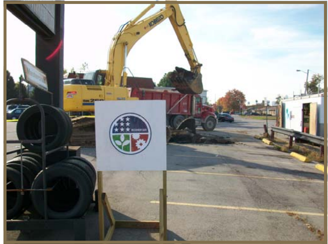
ARRA sign posted on-site, with excavation underway.
