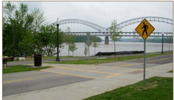
River bank stabilization activities designed by the U.S. Army Corps of Engineers made this portion of the trail possible.
