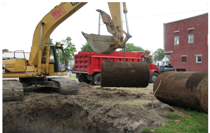
Removal of underground storage tanks
