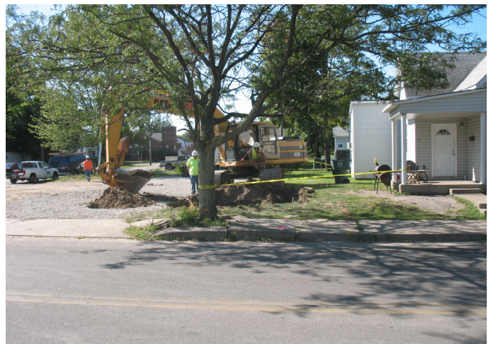
Excavation of soil from adjacent property
