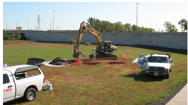
Former Tank 8 Test Pits
