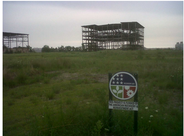
Former Building 13-H
