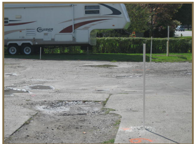
Former gasoline tank basin
